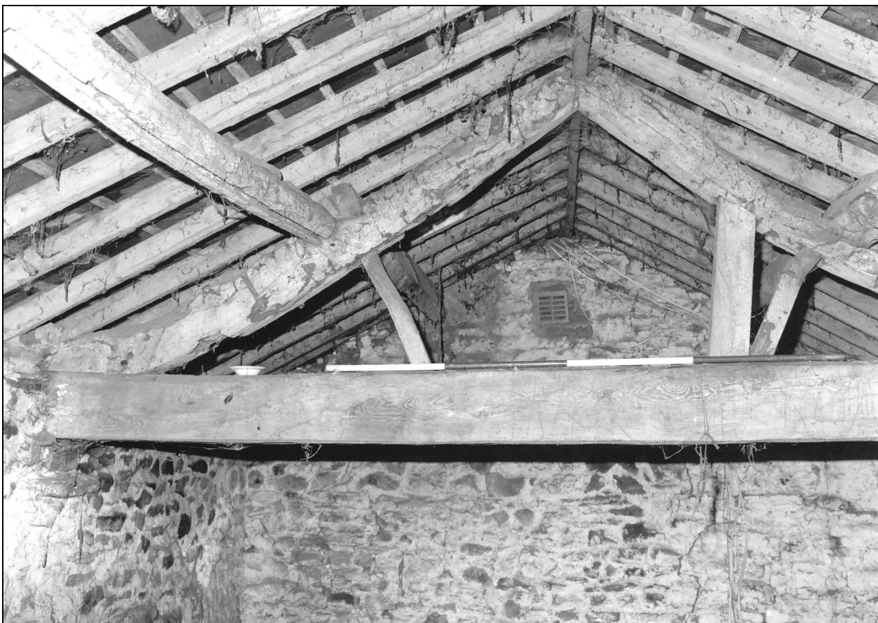
Photo 21: Roof truss in barn, from the south-west
