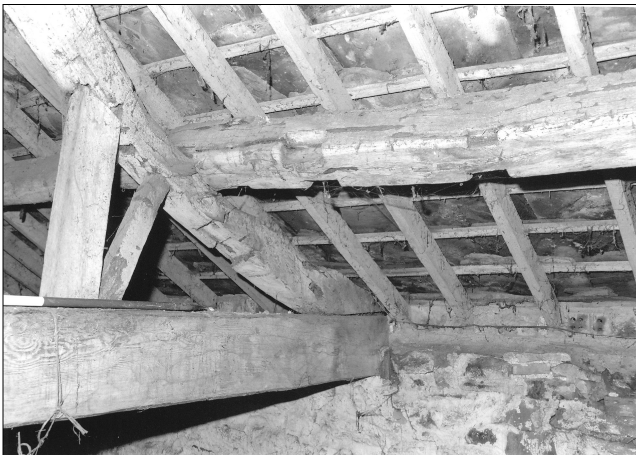
Photo 24: Detail of purlin and north end of roof truss in barn, from the east
