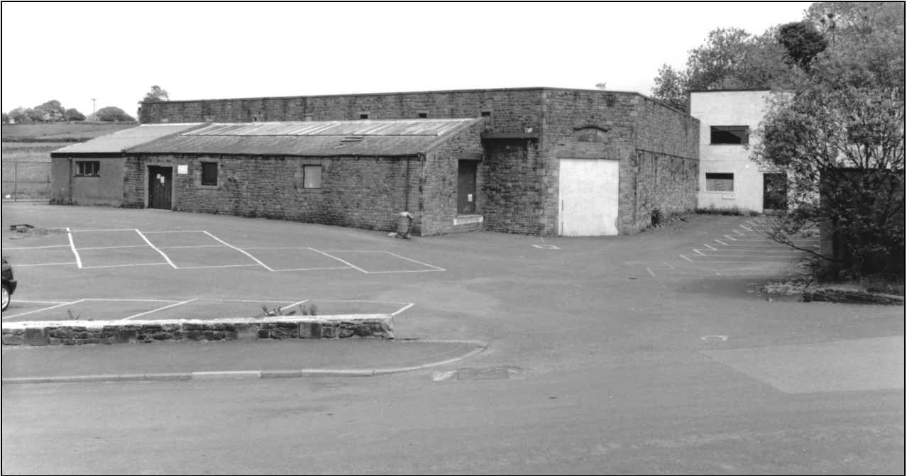
Photo 1: General view of the 1912 weaving shed, from the south-west
