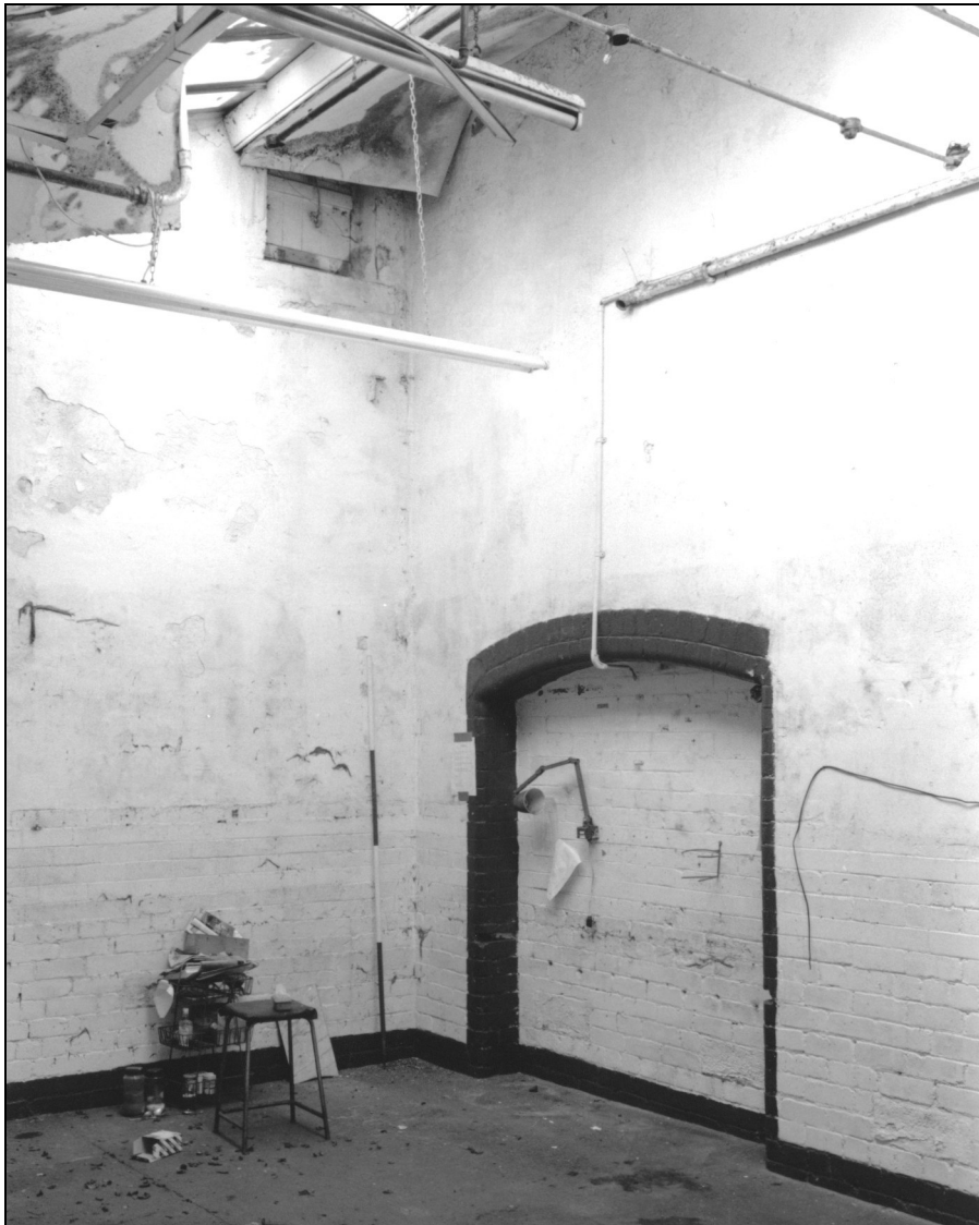
Photo 25: Interior of weaving shed: blocked external doorway and ventilation shutter, in south-east corner
