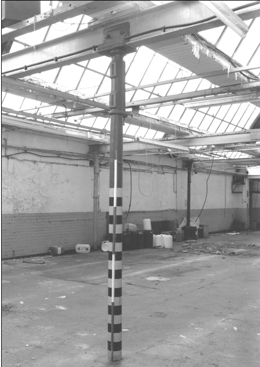
Photo 27: Interior of weaving shed: detail of column, from the south-west
