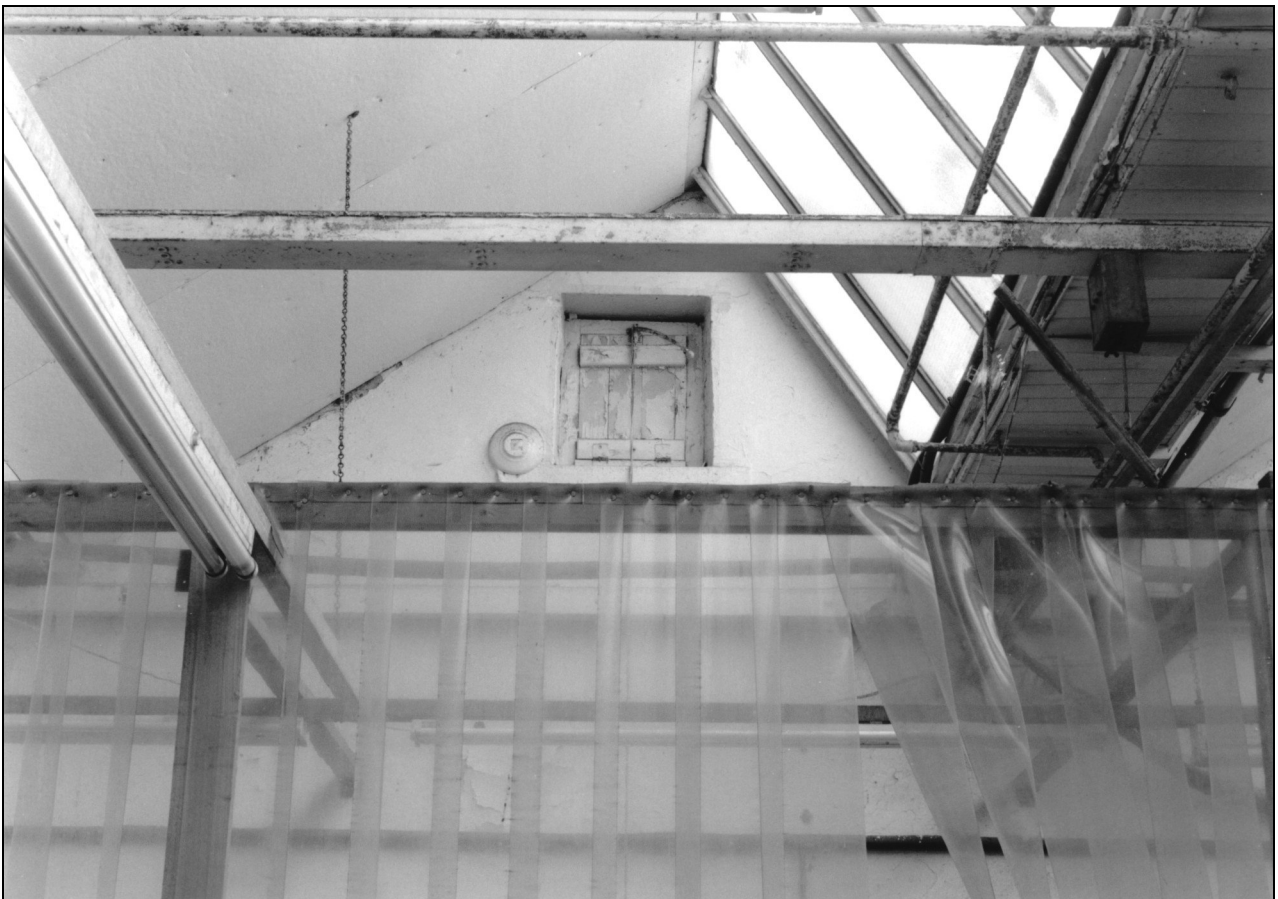
Photo 33: Interior of weaving shed: detail of ventilation shutter in west side
