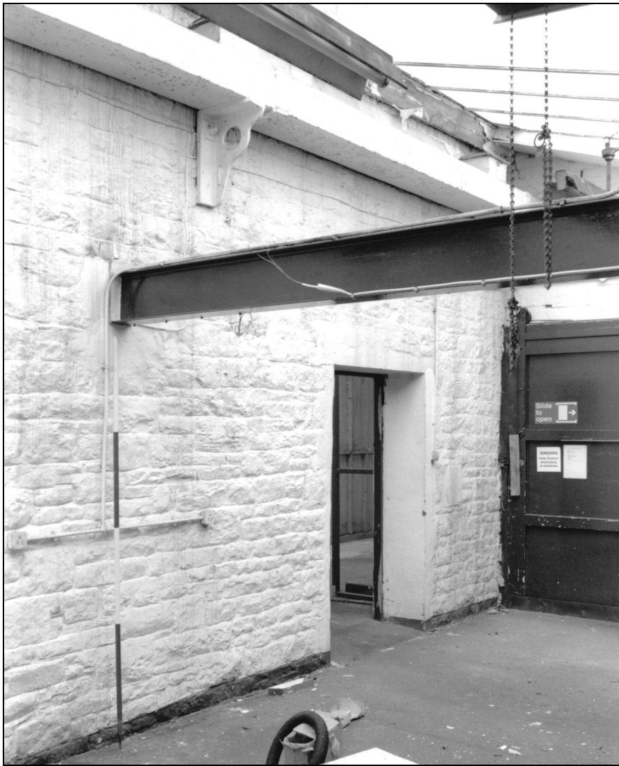
Photo 16: Interior of west addition, showing cast iron gutter on original external wall, from the north-west
