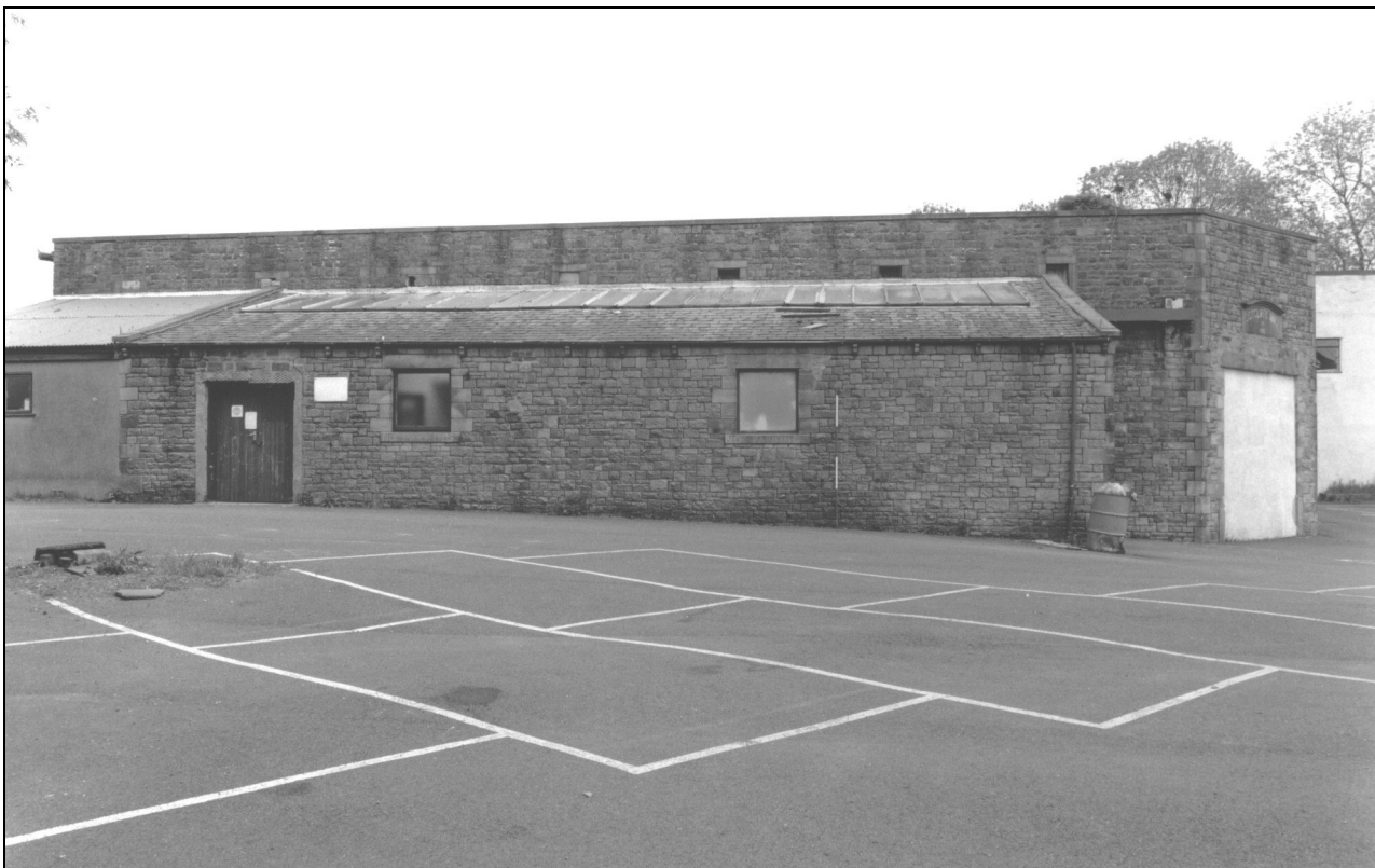
Photo 10: The weaving shed and west addition, from the west
