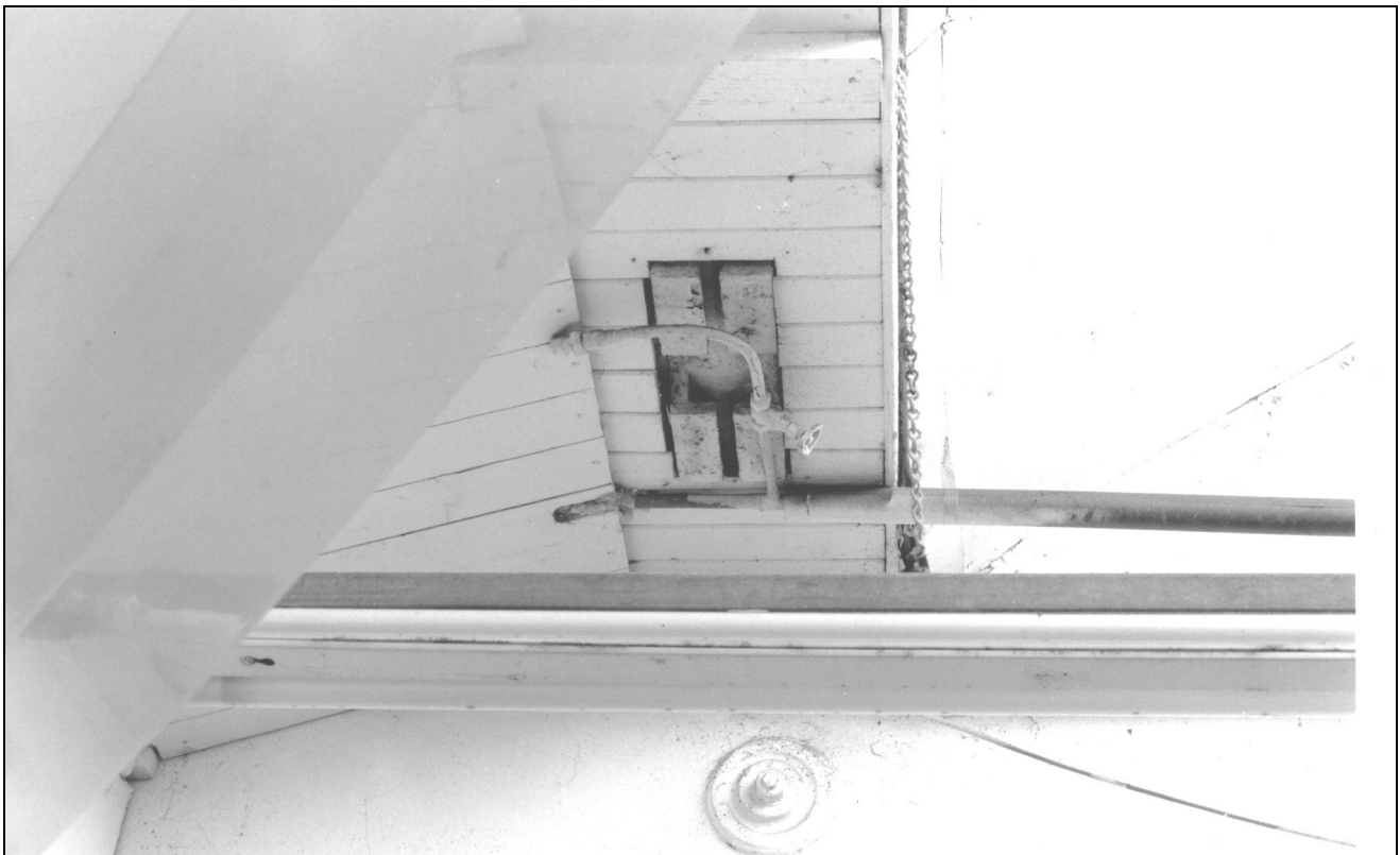
Photo 31: Interior of weaving shed: detail of shaft hanger below roof valley, from the west
