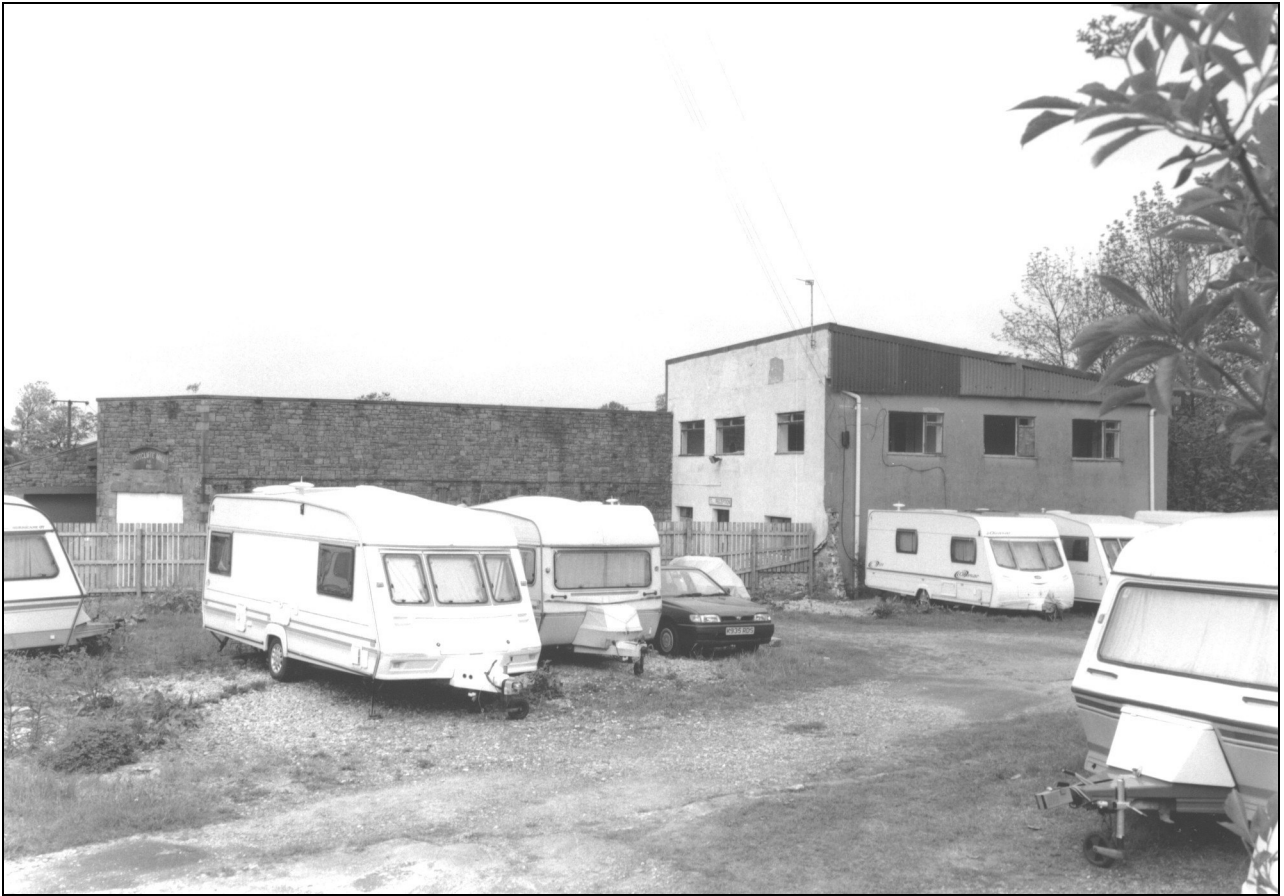
Photo 3: The weaving shed and office block, from the south, across the site of other demolished buildings
