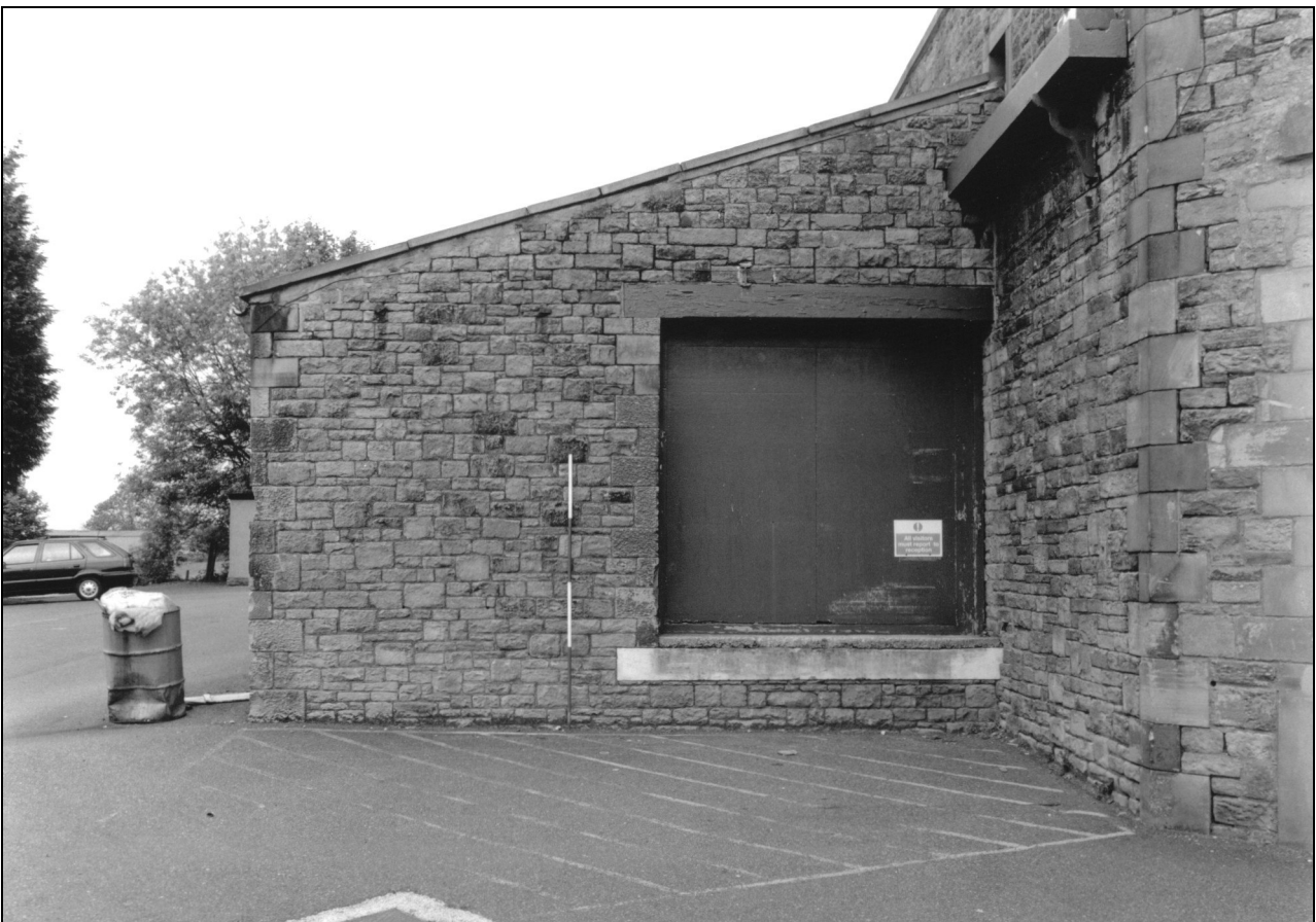
Photo 34: South side of west addition to weaving shed
