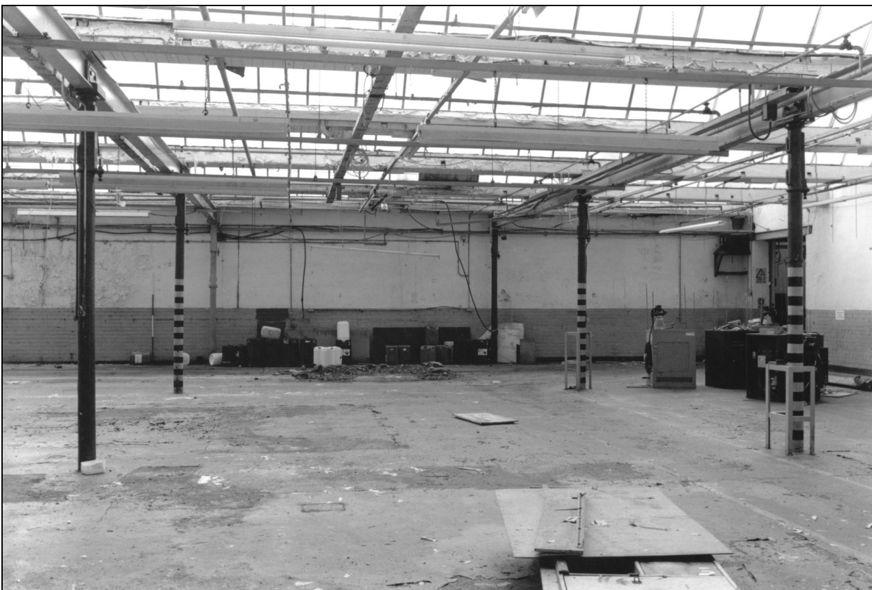
Photo 23: Interior of weaving shed: north side, from the south
