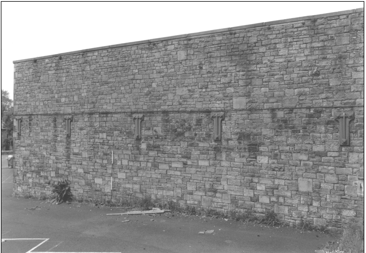
Photo 6: South side of weaving shed, from the south-east, showing tie-plates for interior shaft
