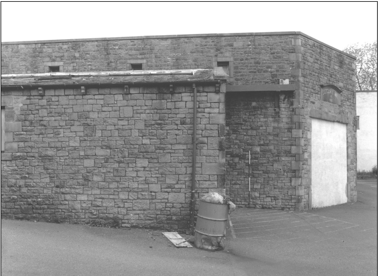
Photo 11: Detail of west elevations of weaving shed and west addition
