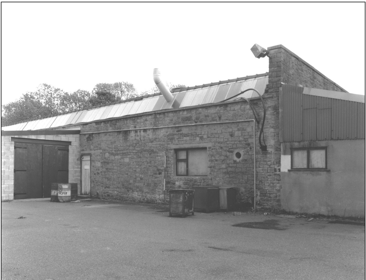
Photo 12: North side of weaving shed, from the north-west
