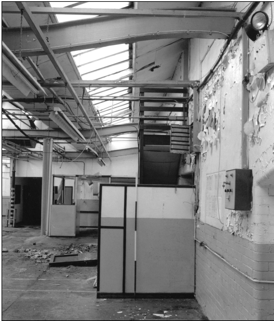
Photo 30: Interior of weaving shed: south side, from the west, showing curved beams overhead
