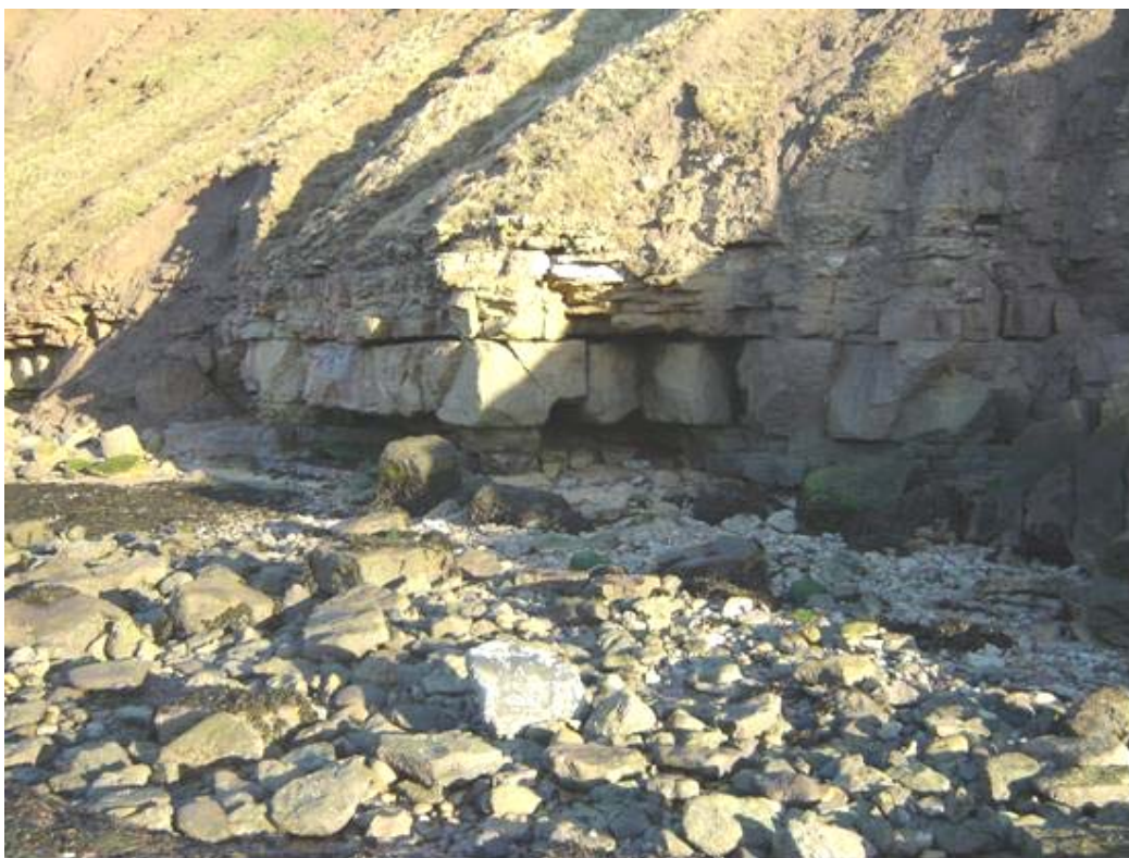
Plate 44 Quarry on southern side of Filey Brigg, near Agony Point (FY9), showing remains of supporting pillars, looking north-west
