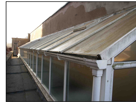
7.9 View along parapet on east side of church hall looking south.
