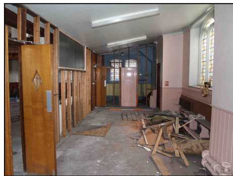
4.4 View of partitioned area at west end of church.
