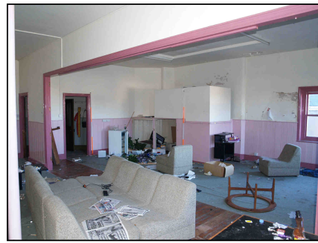
7.2 View of south end of Room F1.
