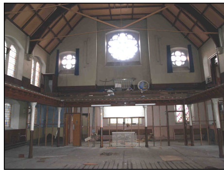
4.1 View of west end of church.
