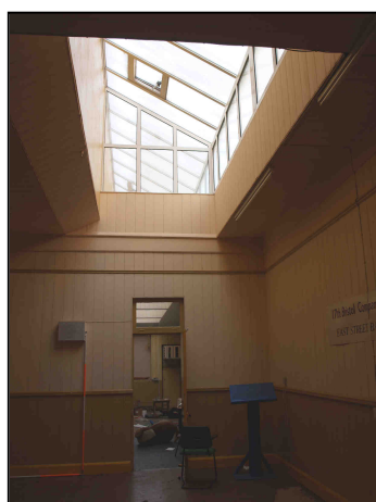
6.7 View of skylight in Room G2 looking northwest.
