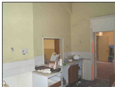
6.5 View of north side of Room G4.
