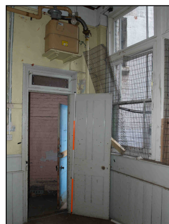
6.8 View of south side of Room G3.
