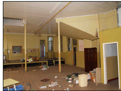
6.2 View of south end of Room G1 looking south.
