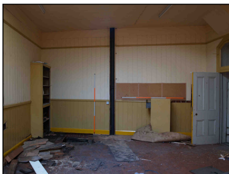
6.4 View of south end of Room G2.
