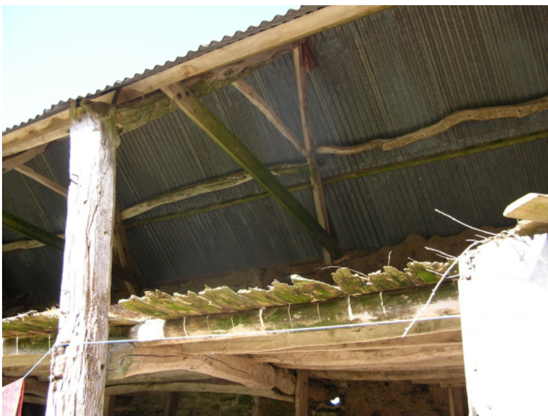
Plate 30. The linhay barn hayloft and roof of the northern range, from the south-east, showing the A-frame roof with pegged lap-jointed collars
