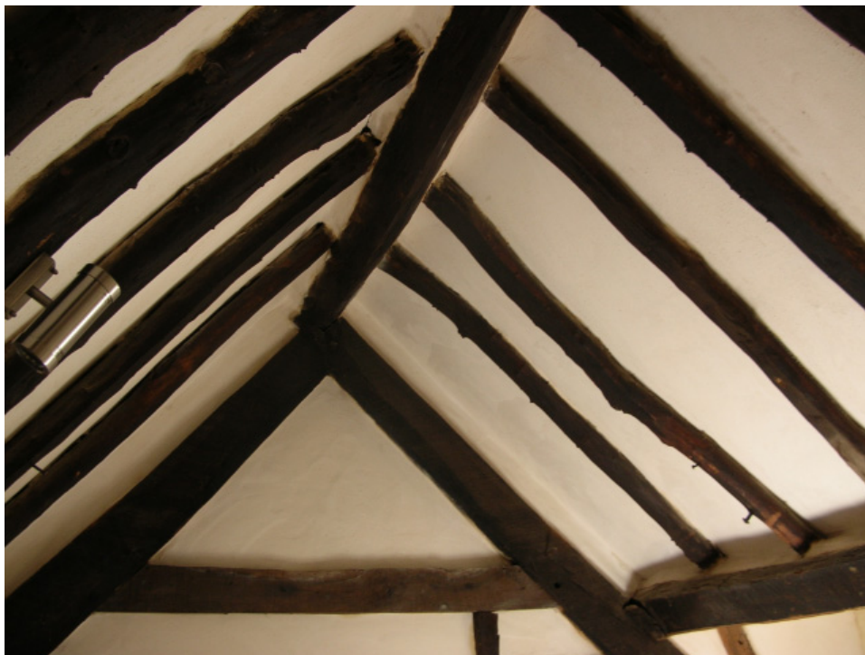
Plate 25. Roof of side-pegged jointed cruck construction in the main bedroom above the hall, from the west
