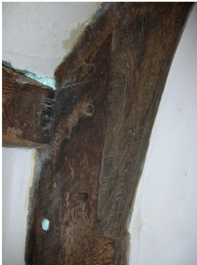
Plate 14. Cruck hip with pegs and protruding wall plate in the north-east corner of the gallery
