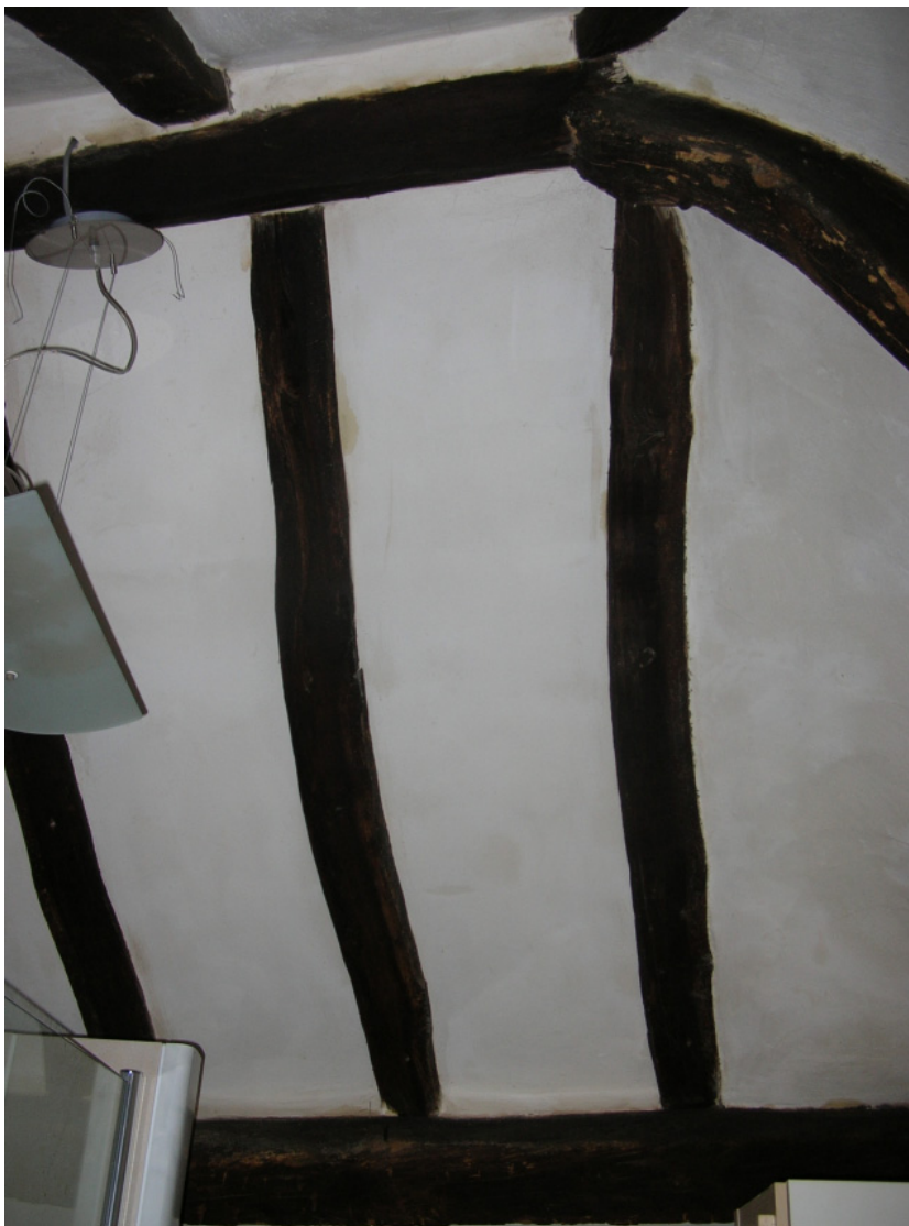
Plate 23. The side-pegged jointed cruck roof trusses within the bathroom (above the inner room), from the north
