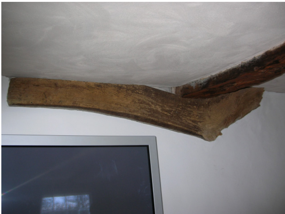
Plate 21. Re-used cruck blade supporting the crossbeam in the lounge of the western extension, from the south
