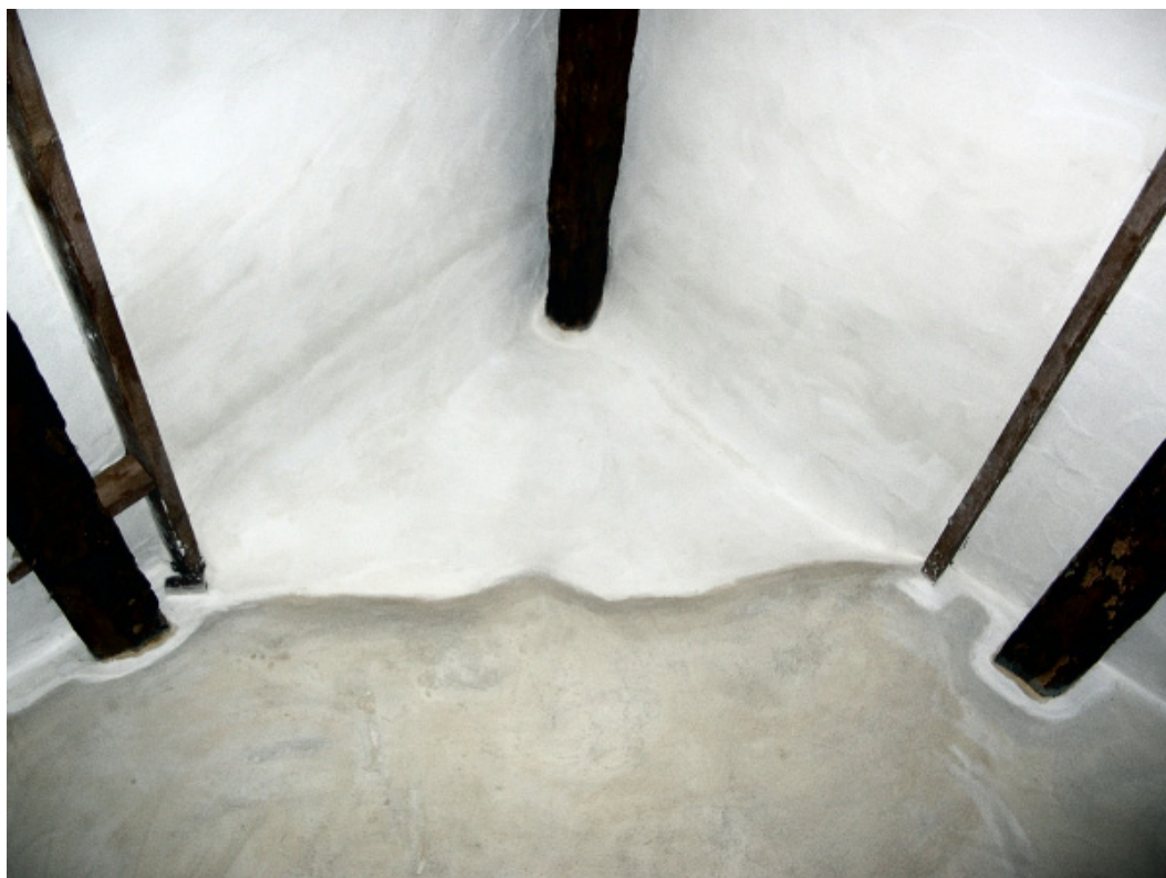
Plate 16. Wall between the service end and the cross-passage, from the east. Note the change in the depth of the render above the purlins
