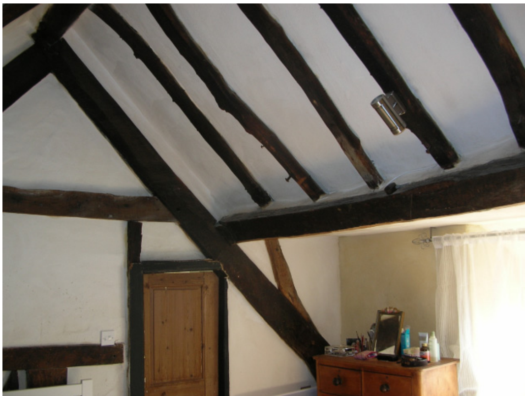
Plate 29. The main bedroom above the hall from the north-west, showing the extra room created between the original eaves and purlins after the eaves were raised
