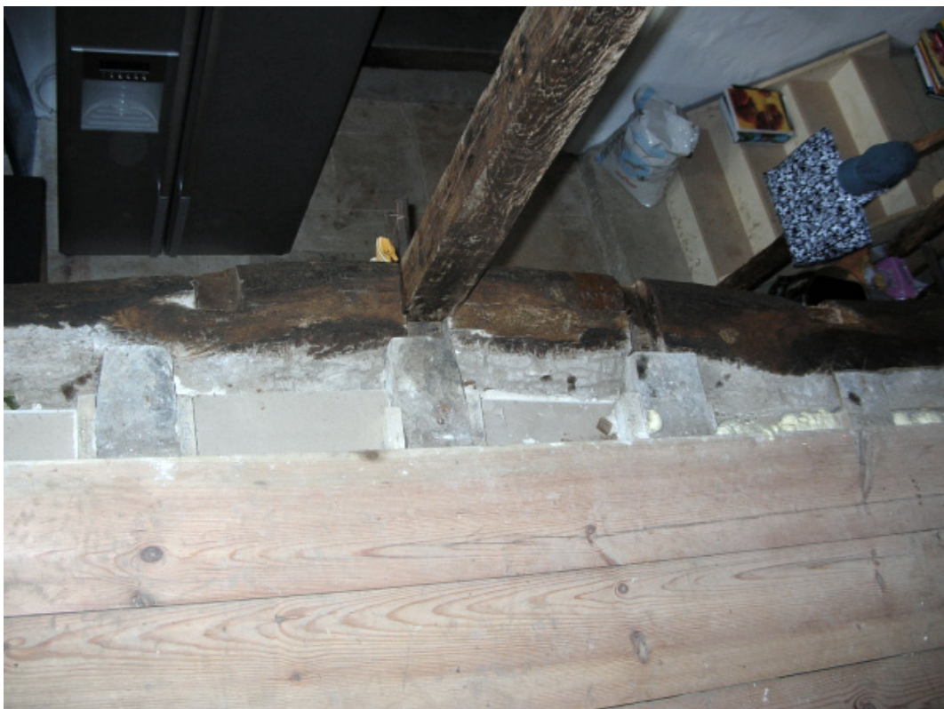
Plate 15. View from gallery looking down into the kitchen, from the east. Note the beam slots in the crossbeam pointing towards the west
