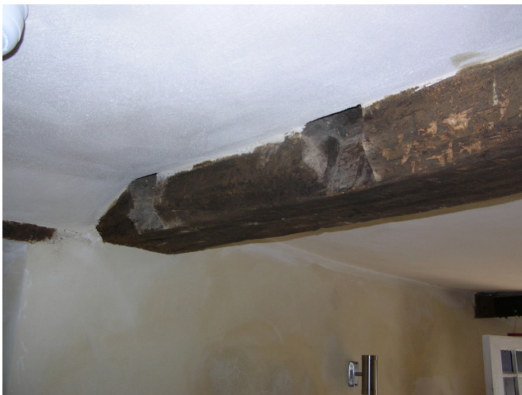
Plate 20. Two vertical beam slots within the east to west crossbeam in the inner room, from the north-west
