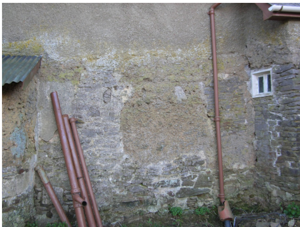
Plate 10. North elevation of original building, between the bread oven and smoking chamber chimneys to the left and the stair turret to the right, showing remedial work in the cob walling
