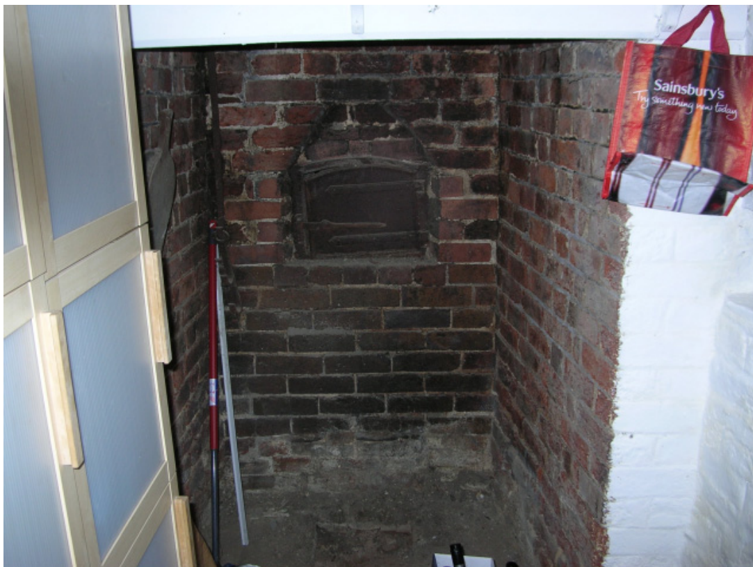
Plate 17. Bread oven and smoking chamber at the northern end of the cross-passage, with part of the original rubble wall to the right
