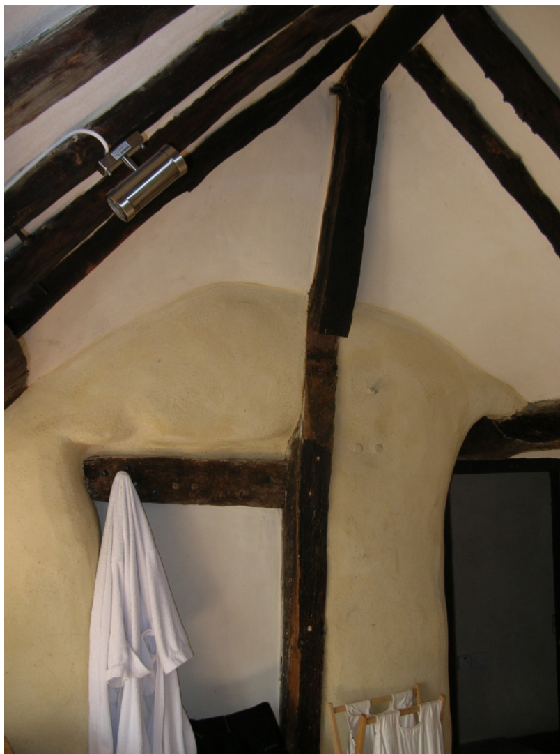
Plate 27. East facing wall of the main bedroom showing two lapped vertical timbers supporting the ridge pole, and a blocked doorway, from the south-east
