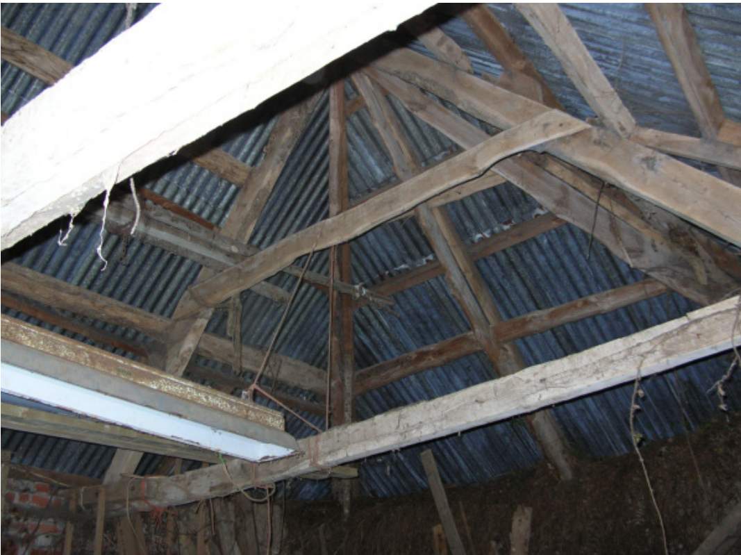
Plate 32. A-frame truss roof with pegged lap-jointed collars within the byre of the southern range, from the north-east
