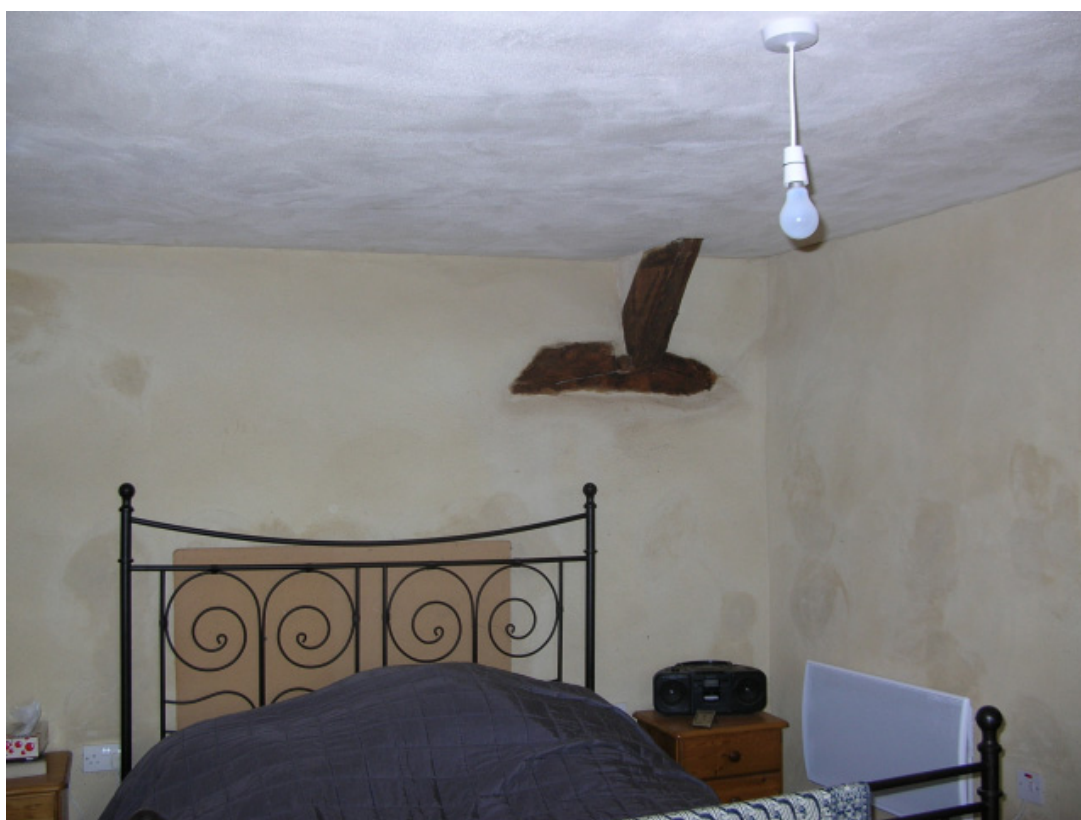
Plate 22. Junction of A-frame rafter and wall plate visible in the northern wall of the eastern bedroom within the western extension
