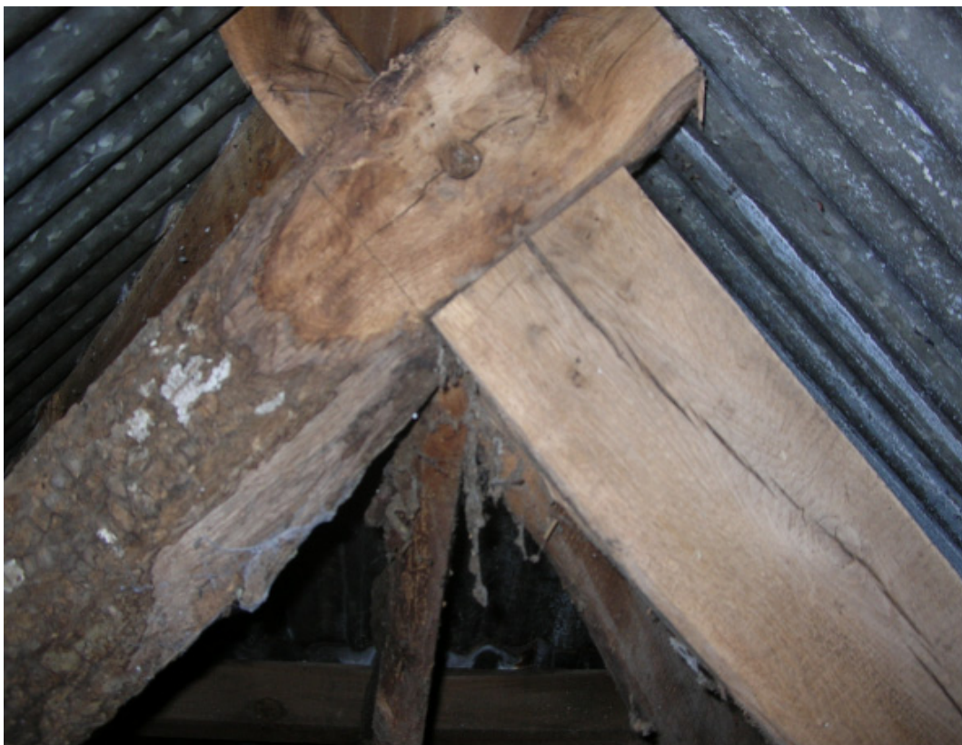
Plate 33. Close-up of a the ridge element of the A-frame truss roof with pegged lap-jointed collars within the byre of the southern range
