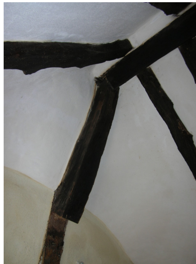
Plate 28. Close-up of two lapped vertical timbers supporting the ridge pole in the east facing wall of the main bedroom, from the south-east
