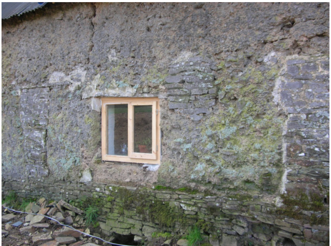
Plate 8. Three rubble-filled blocked openings at eastern end of north elevation of original building, from the north-west
