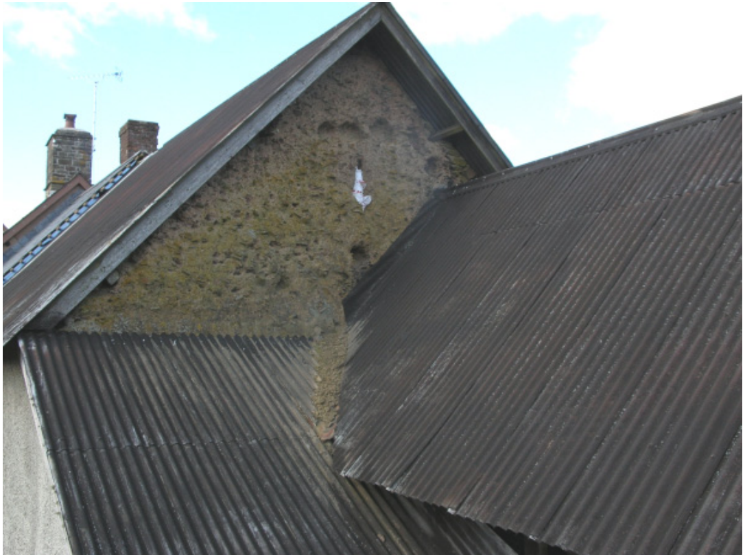
Plate 7. Eastern gable of hayloft, constructed of cob with ventilation slit in centre
