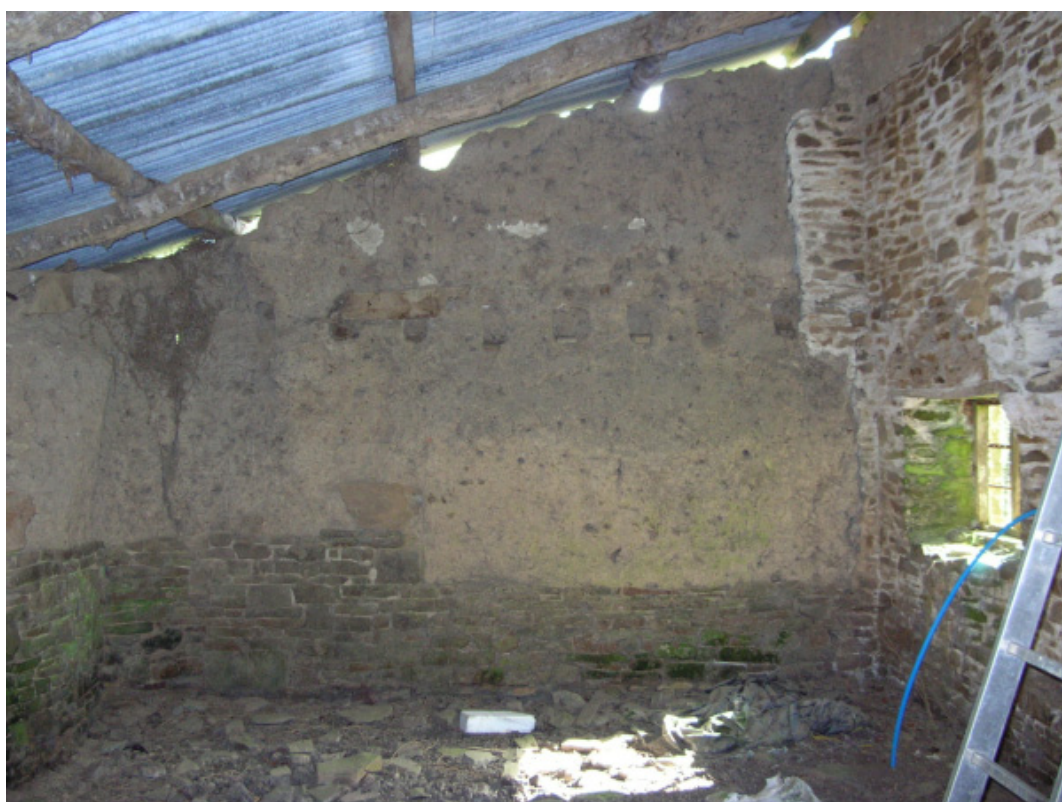
Plate 36. Interior of angled building at east end of southern linhay showing joist holes in cob wall, and rubble wall on the right, from the north-west
