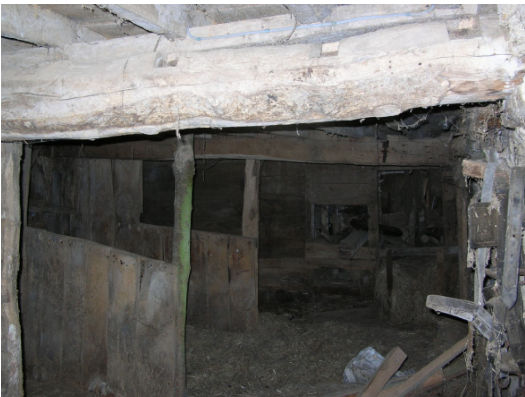
Plate 34. Original crossbeam of southern byre with joist slots, below new crossbeam supporting hayloft floor, from the north-east
