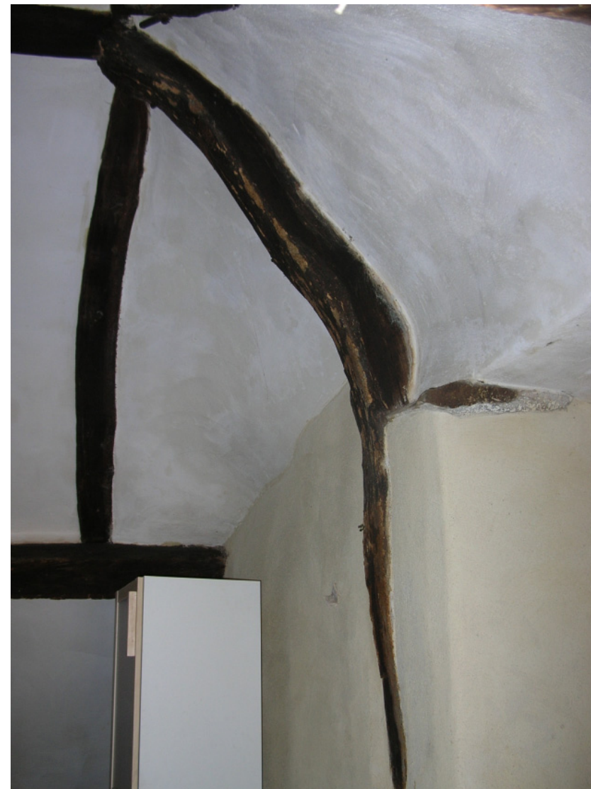
Plate 24. The curved King Post supporting the ridge pole of the roof above the bathroom (above the inner room), from the north
