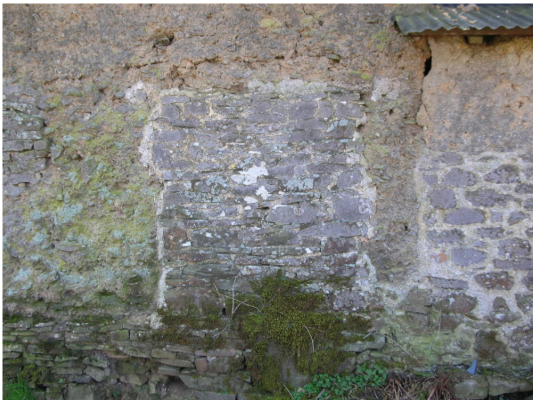
Plate 9. Rectangular blocked opening in north elevation of original building, to the left of one of the bread oven and smoking chamber chimneys
