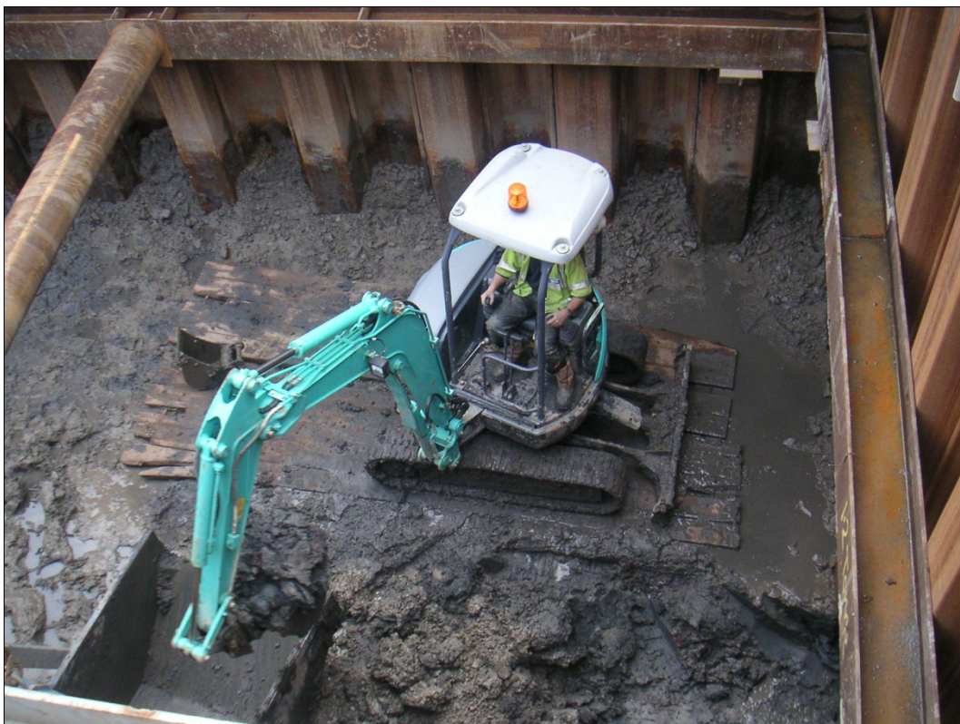
Plate 2. Machine excavating trench surrounded with sheet metal shoring
