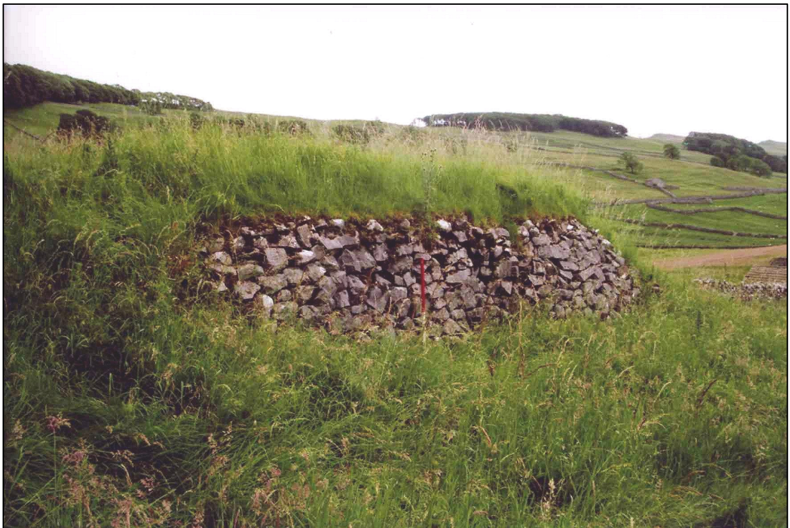
Plate 4: Revetment on west side of platform (Site 12), looking S.
