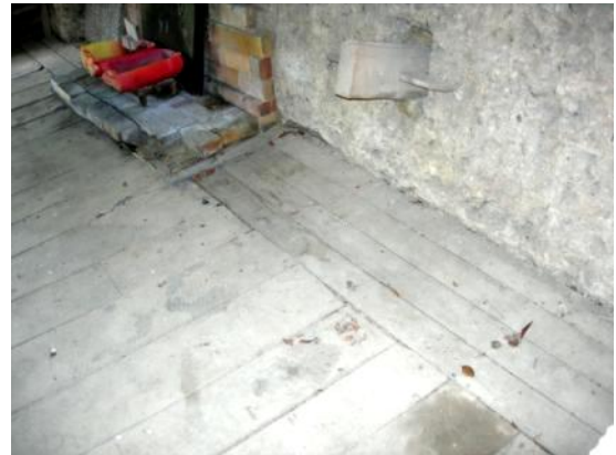
Detail of floor boarding in S linhay
