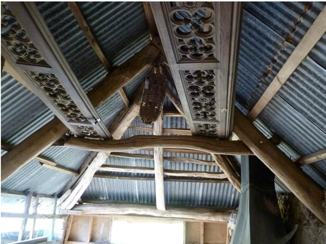
P12. Roof structure in southern linhay, looking east
