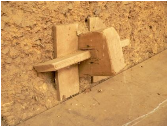
Pegged end of lean-to rafter, S wall
