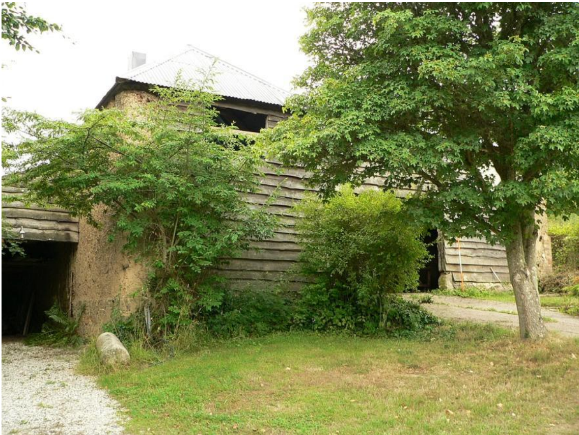
P2. East elevation, from the south-east, with the lean-to extension on the left side
