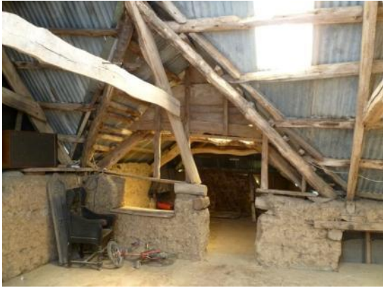
Cut through to tallet floor, N linhay
