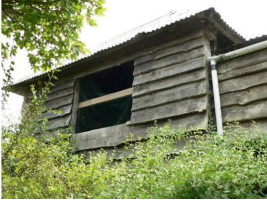
Weatherboarding on S linhay, E end
