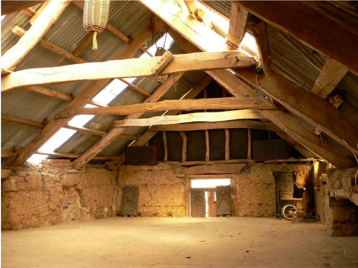
P9. First floor and roof of threshing barn, looking north
