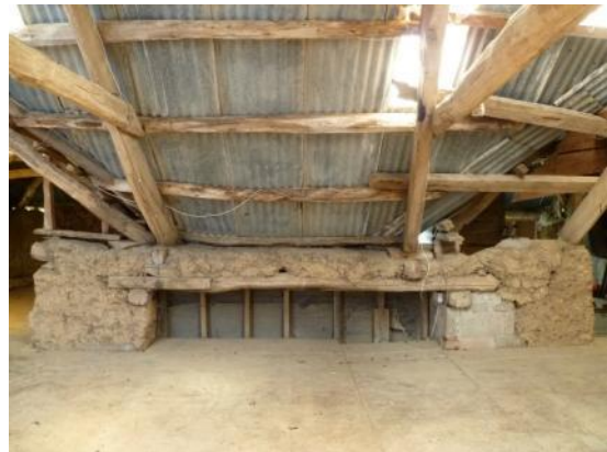
Beam and cob over head of E doorway
