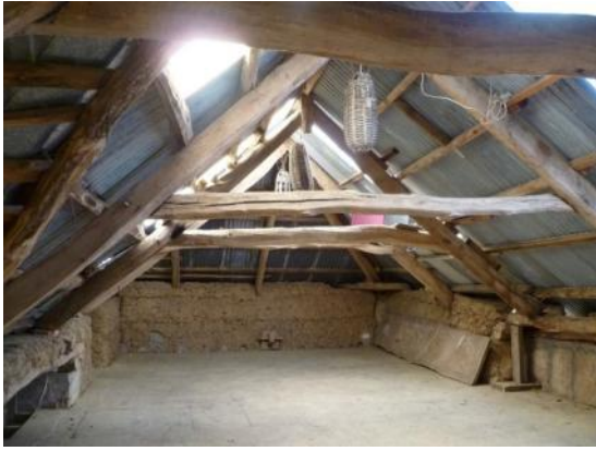
First floor of barn, looking S
