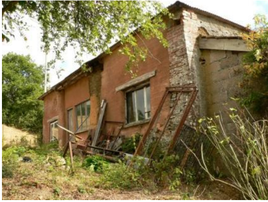
W elevation of barn from SW
