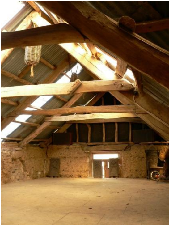
Barn roof, looking
