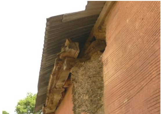
Porch over W central doorway to barn
