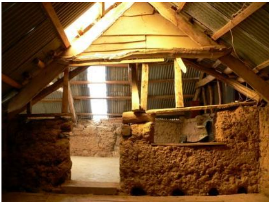
N linhay, looking W to barn wall
