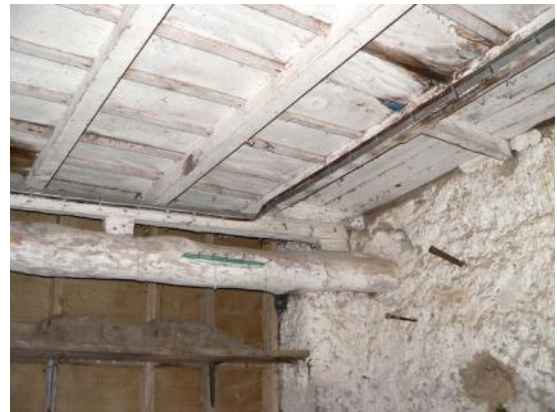
E end of S linhay, with secondary timber above cross beam to level floor. Note boarding to wall where floor was formerly open for feeding mangers
