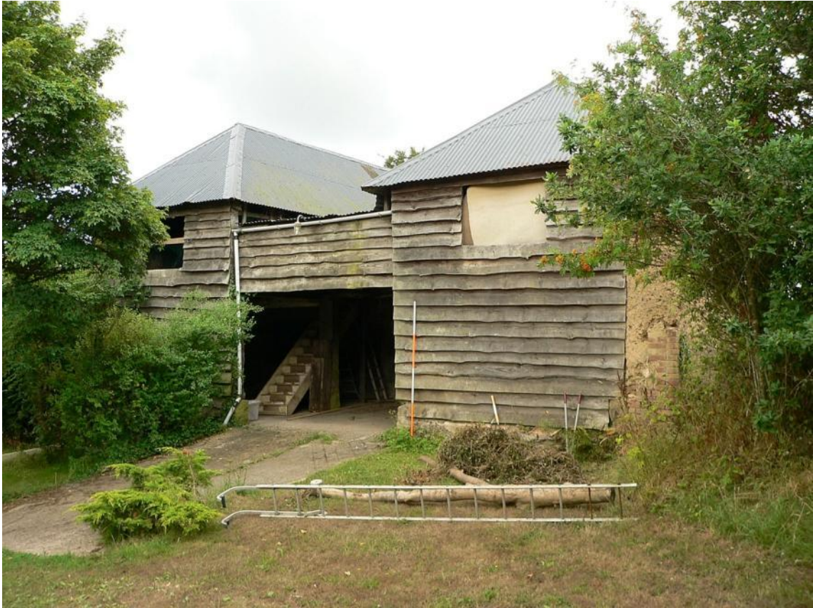
P3. East elevation, from the north-east
