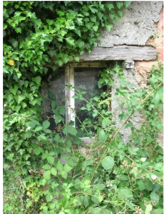
Window in S wall of lean-to
