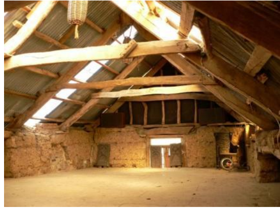
Barn first floor and roof, looking N
