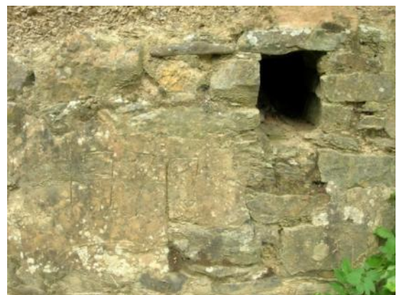
Date '1970' and drain, SE corner of S linhay
