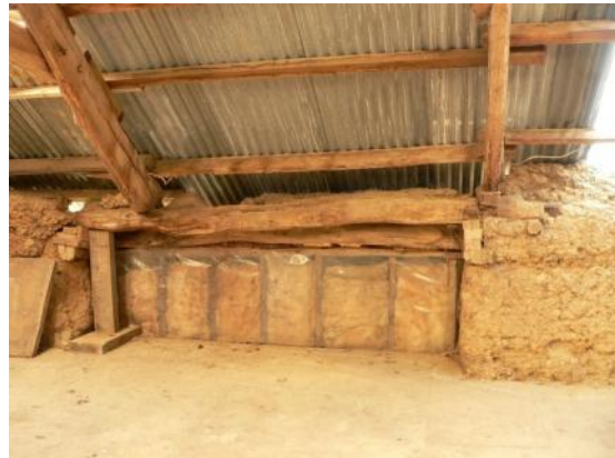
Beam over head of W doorway
