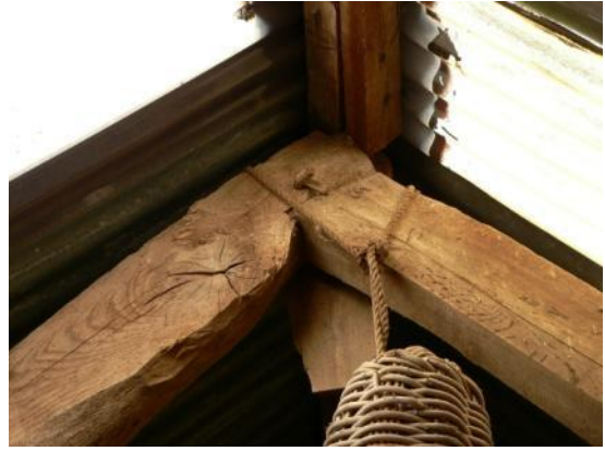
Detail of pegged apex of principals, T4
