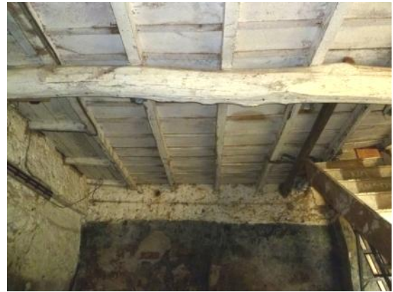
Central cross beam and ceiling on S linhay
