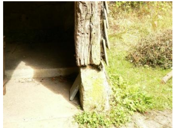
Foot of front linhay post, N side
