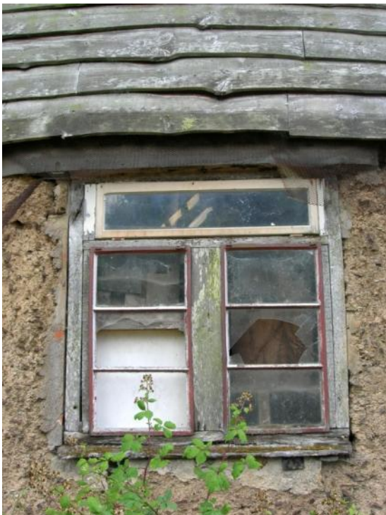
Window in N gable end of barn
