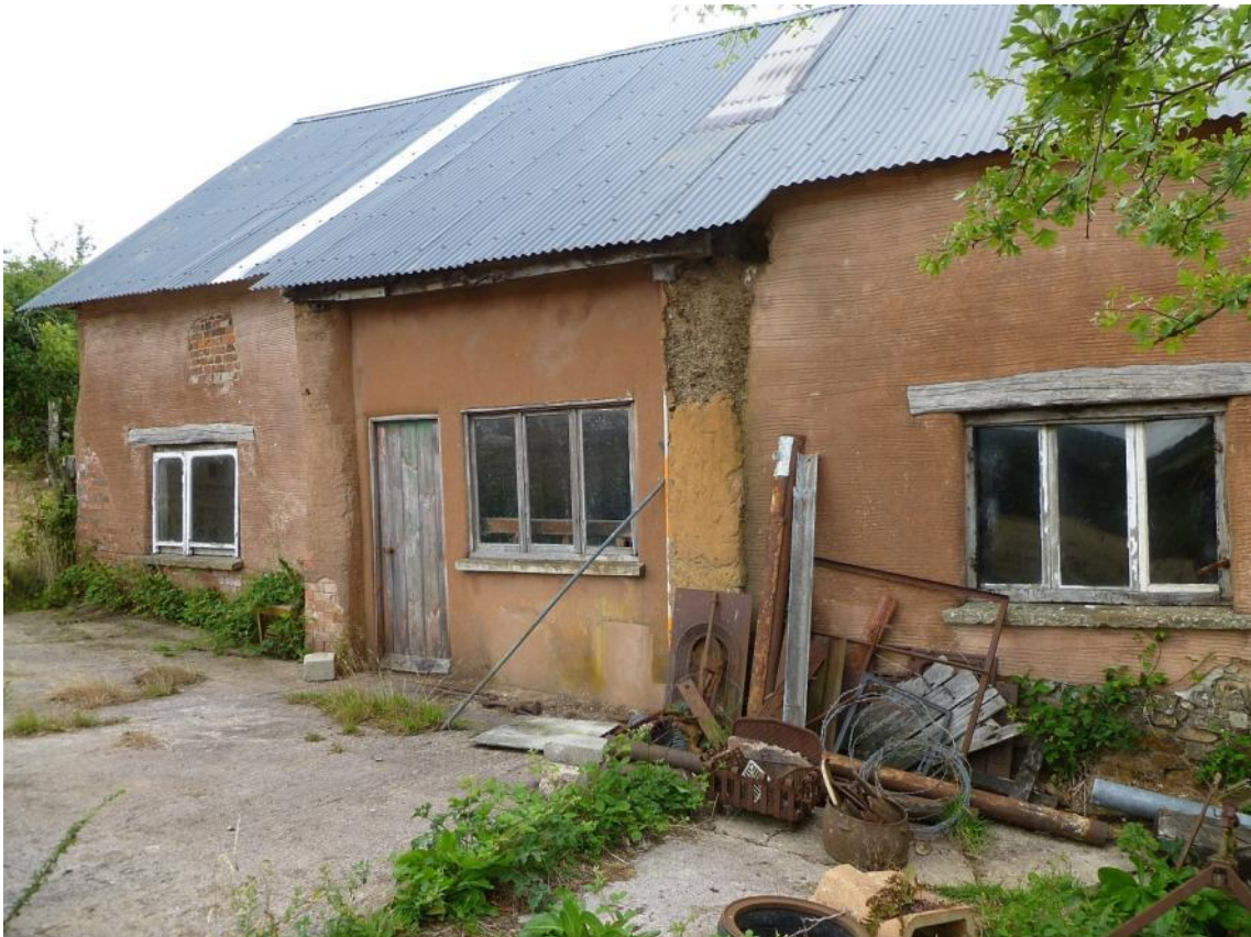
P5. West elevation, from the south-west, showing position of former central doorway
