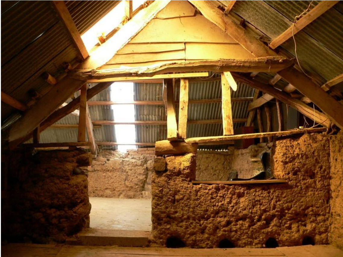
P11. First floor west end of northern linhay, showing cut through barn wall
