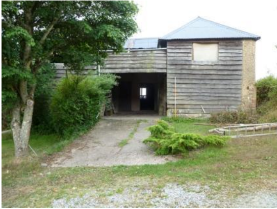
Entranceto barn and E end of N linhay
