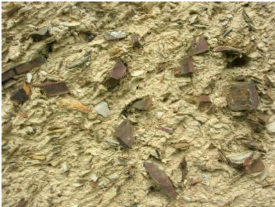
Close up of cob with large shillet inclusions
