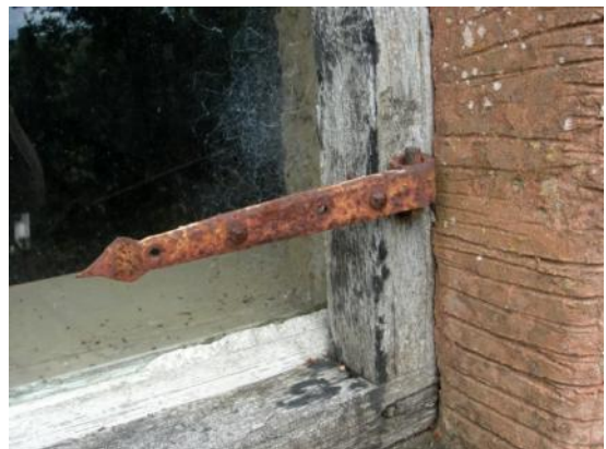
Detail of shutter hinge on S window frame
