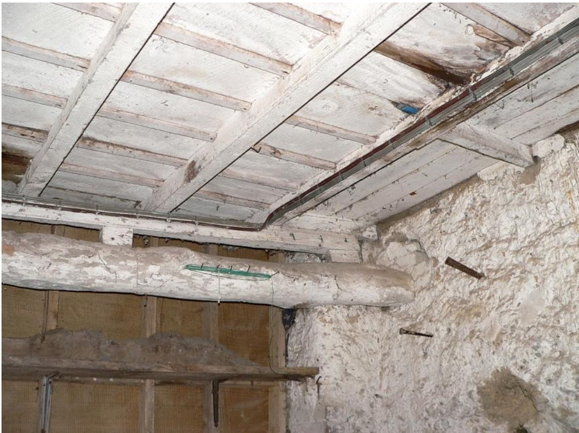
P8. Ground floor ceiling structure in northern linhay
