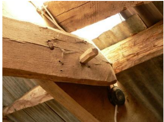
Detail of faceted peg and spike to collar, T4
