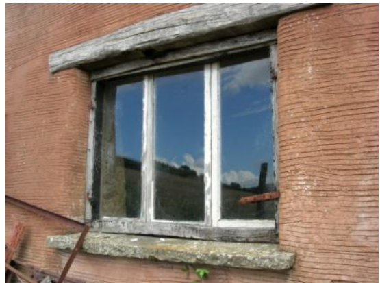
S window on W side of barn
