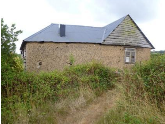
N elevation of N linhay and barn
