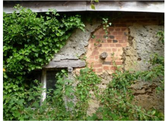
Brickwork repair to cob S wall of lean-to
