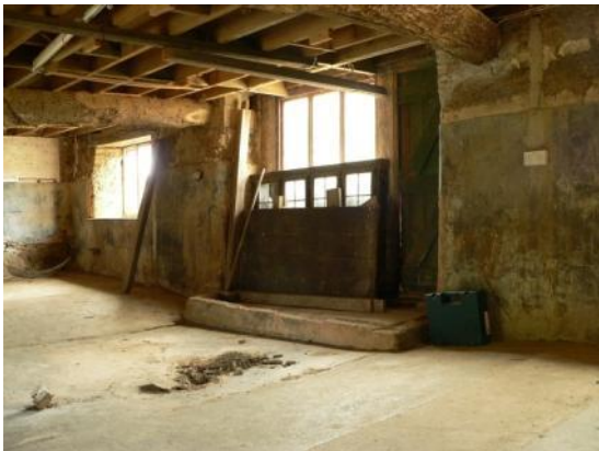
W doorway to barn, from NE
