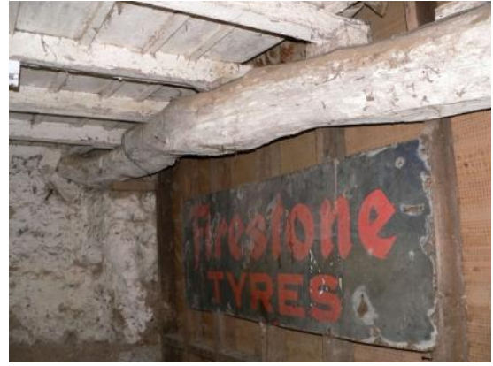
Rustic main beam at E end of N linhay
