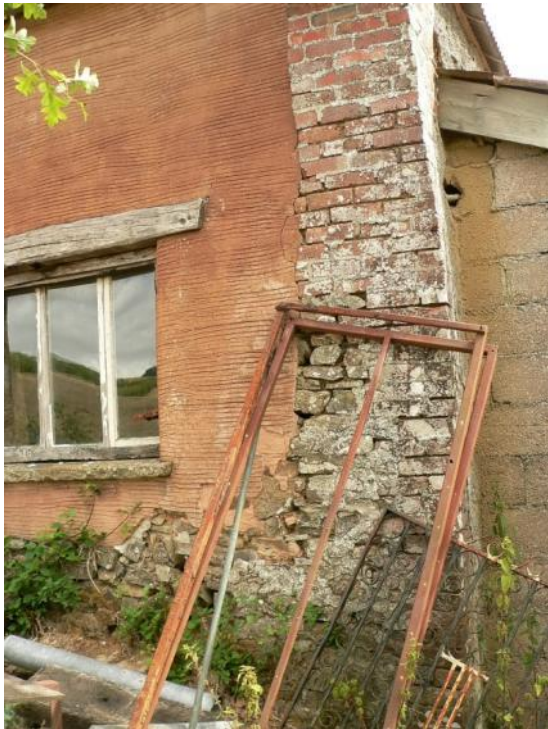
SW corner of barn and end of lean-to
