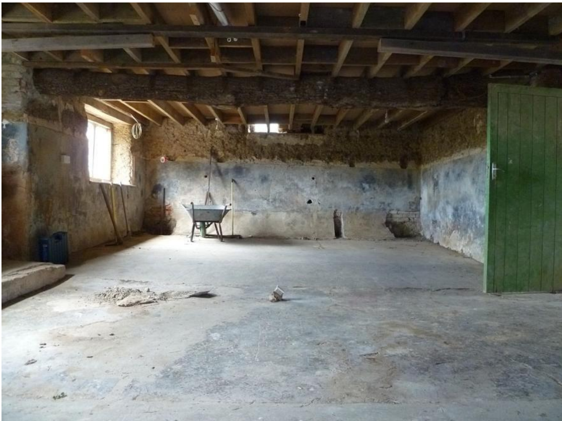
P10. Ground floor of threshing barn, looking to north end
