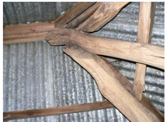
Apex of hip rafters in S linhay
