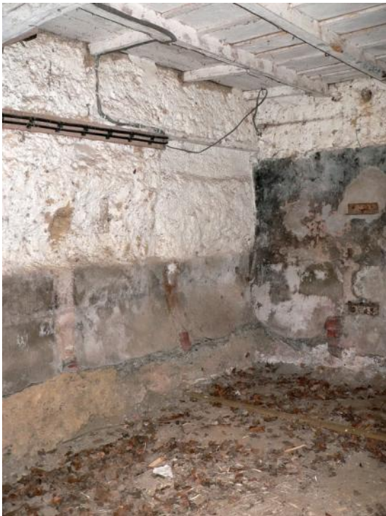
W bay, S linhay, looking to SW corner, with remains of feed/water trough along foot of wall and blocked opening
