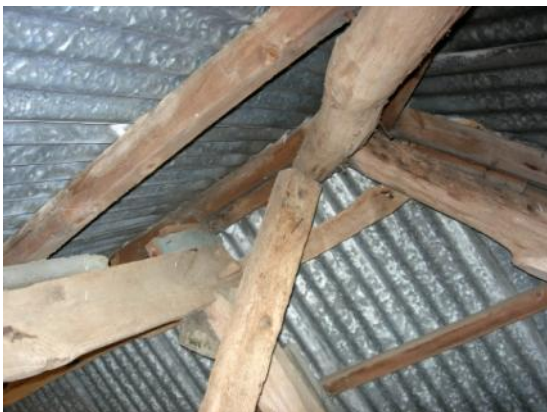
Apex of truss and hip rafter prop, N linhay
