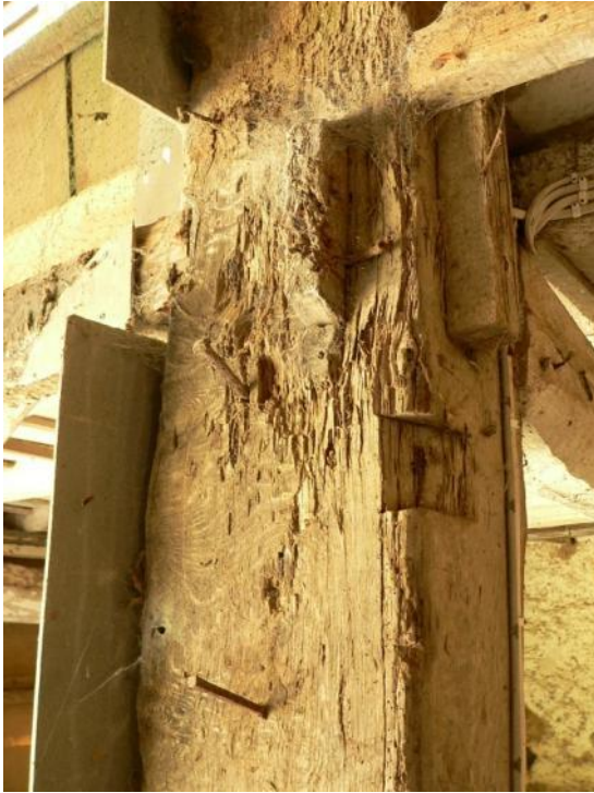
Reused timber, front post to S linhay
