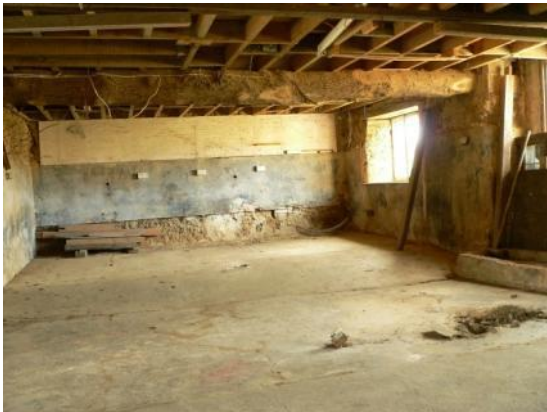
Barn ground floor, looking S
