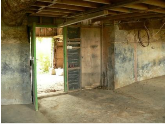
E doorway to barn, from W
