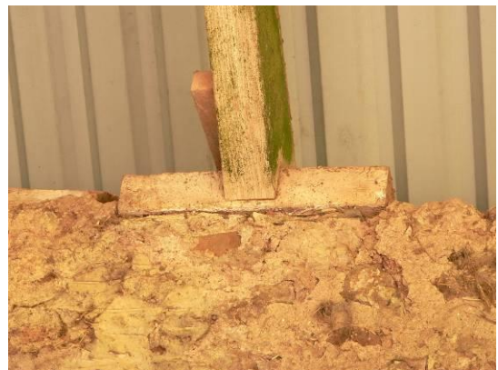
Detail of principal bearing on wall head
