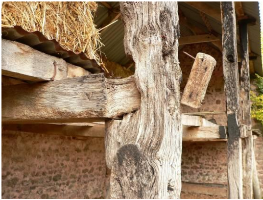
Weathered joint between beam and post
