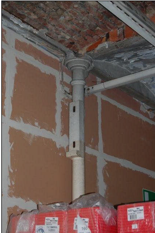
Plate 27: D-shaped bolting head, first floor, Building C
