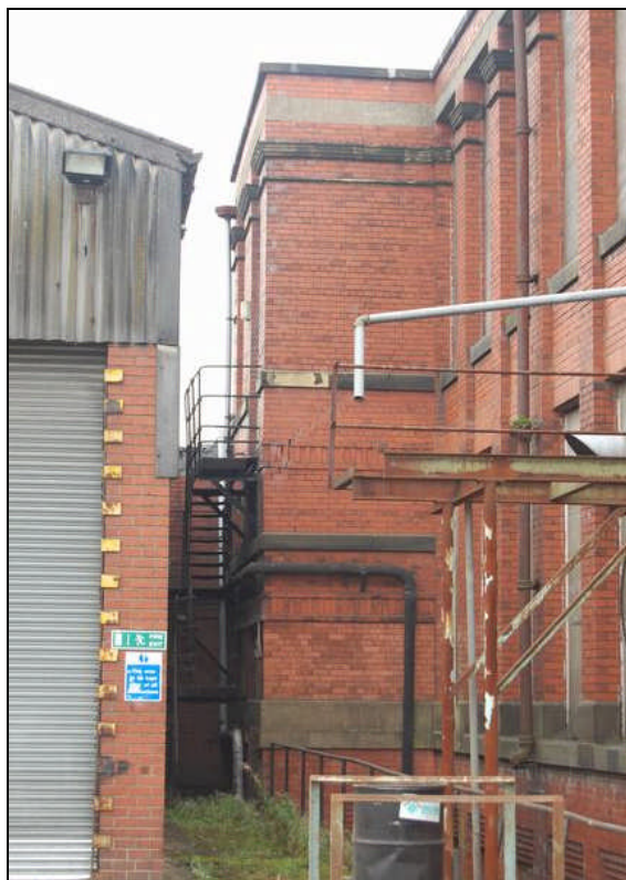
Plate 17: Brick-built hoist tower along south elevation, Building C
