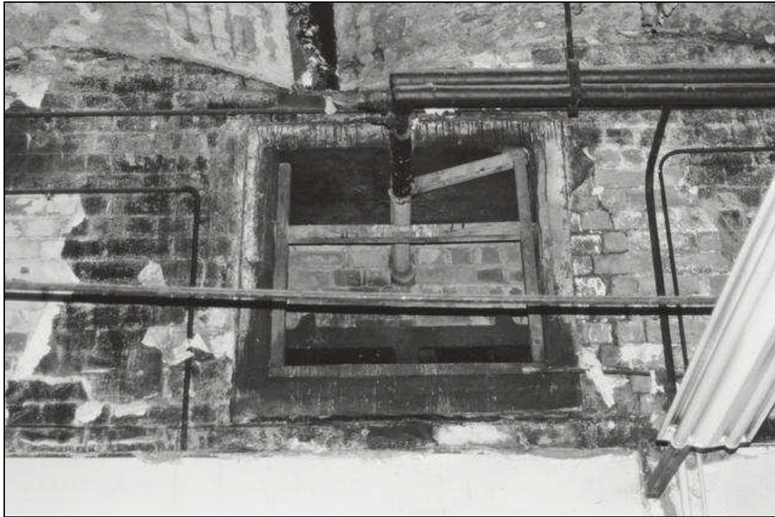
Plate 29: Example of wall box to rope race, first floor, Building C
