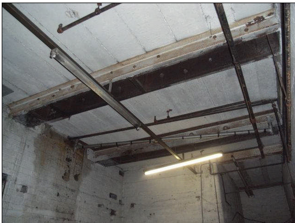
Plate 24: Box girders within rope race, Building C
