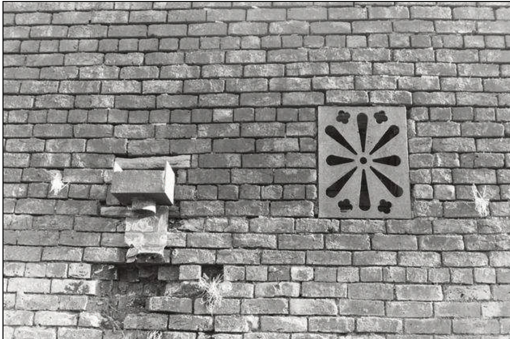
Plate 13: Vent and end of valley gutter, west elevation, Building B
