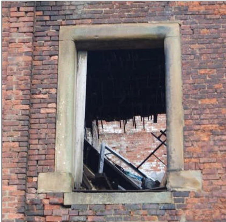
Plate 5: Loading door with sandstone surround, south elevation, first floor, Building A
