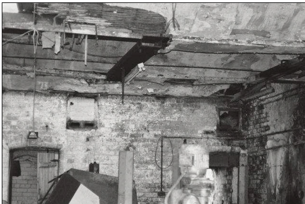
Plate 16: Wall boxes to south wall, Building B
