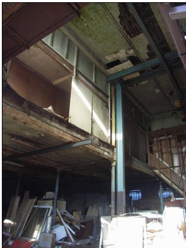
Plate 11: Modern inserted steel structure to southeast corner, Building A
