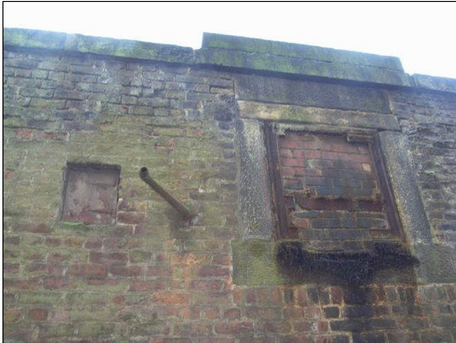
Plate 31: Wall box and hatch, south elevation, Building F
