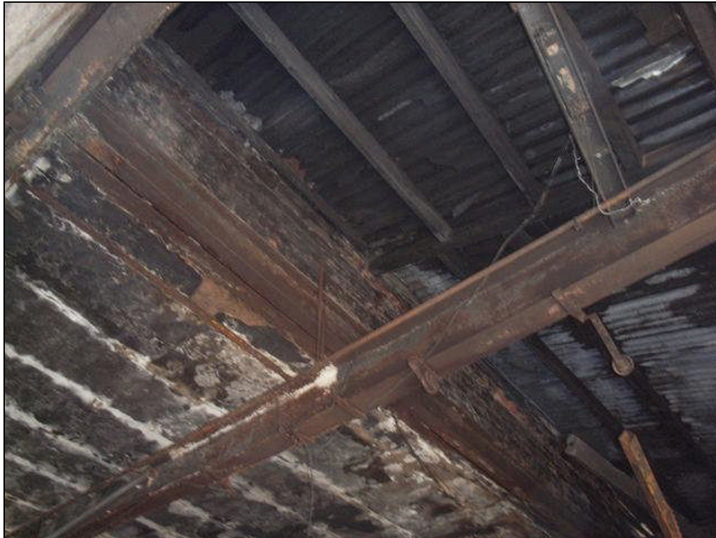
Plate 27: Interior of Building D, showing inserted girder supporting originally external wall of 2-storey portion
