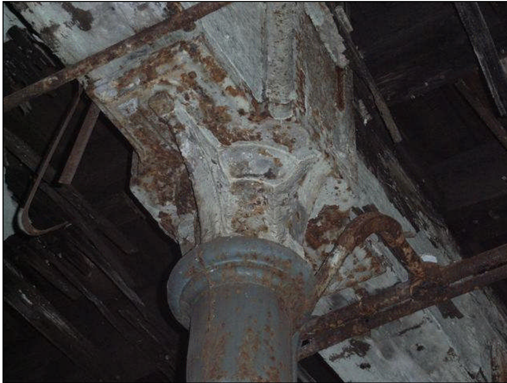
Plate 9: Cast iron column head, ground floor interior, Building A
