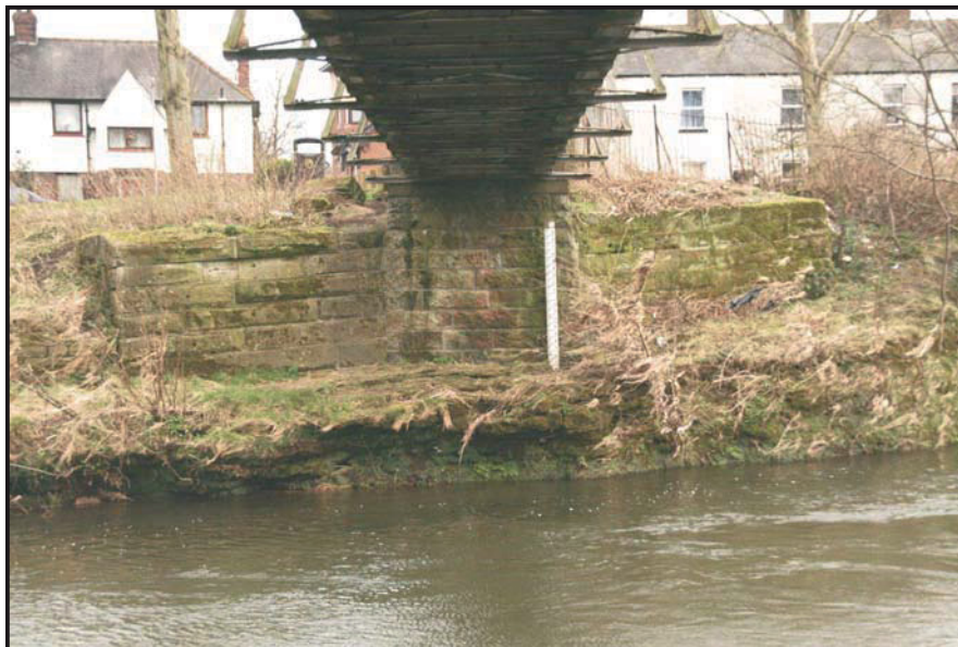
Illus. 06: The masonry of the larger, east abutment of the footbridge.
