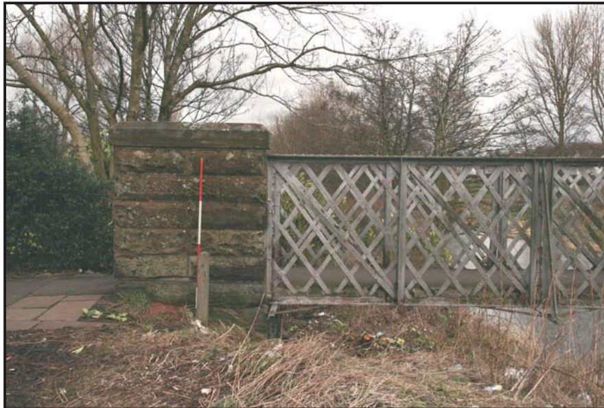
Illus. 05: The SW pier of the Denton Street bridge, the only one of the four piers to retain its capstone in place.
