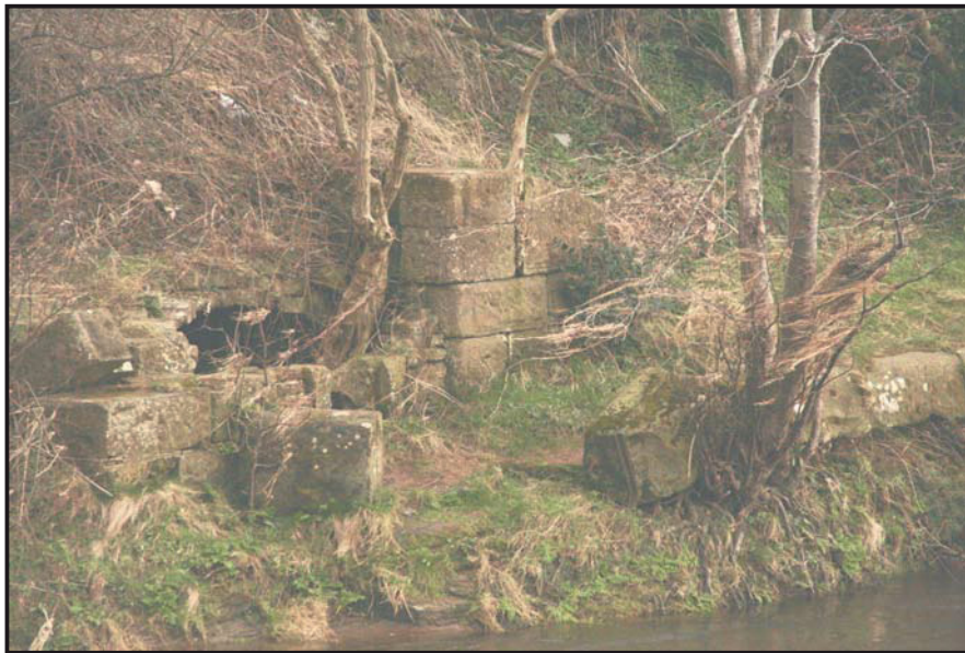
Illus. 09: View of the masonry associated with the Corporation Dam intake and headrace.
