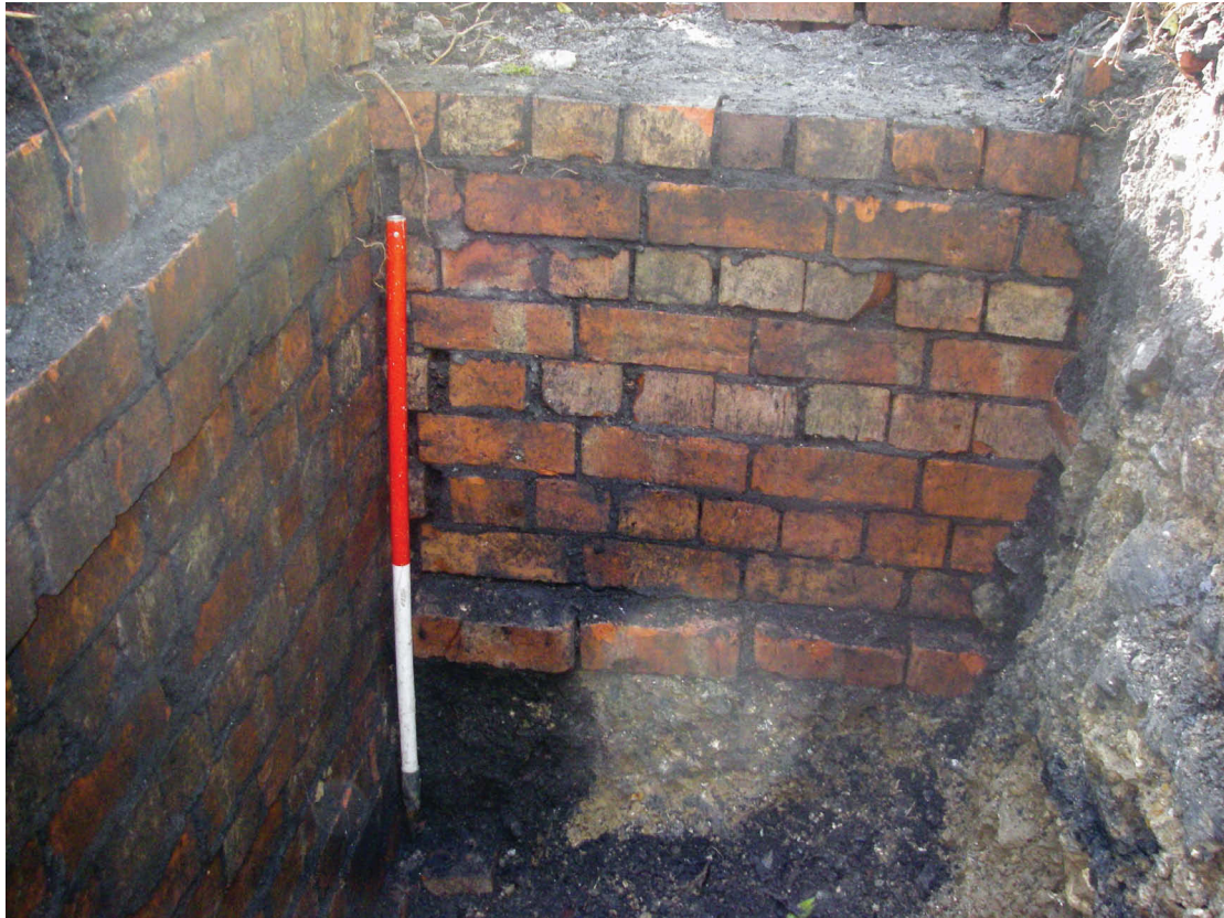
Plate 4: Western wall of pit and southern rope channel, showing cuts into embankment material (107), looking south
