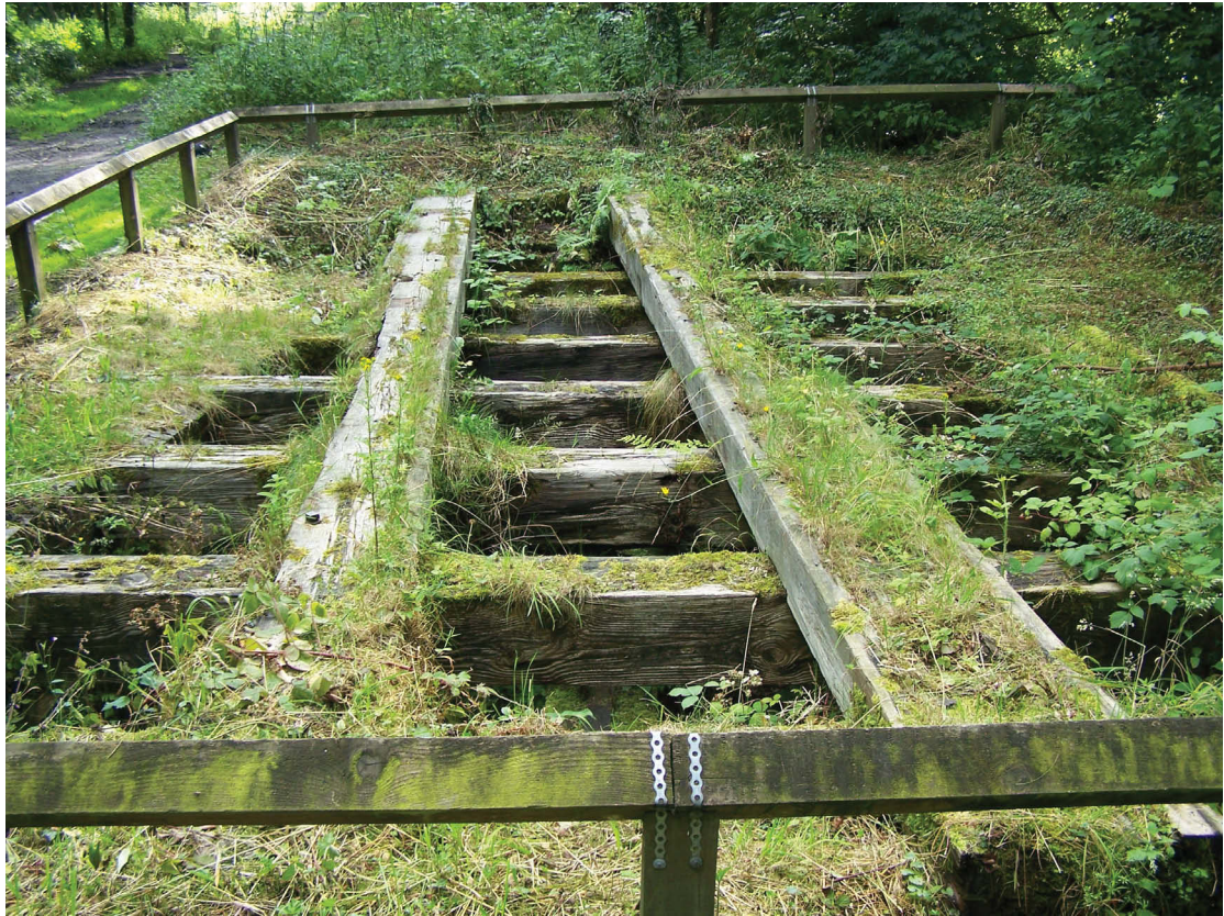
Plate 1: Wheel pit before remediation works, looking east
