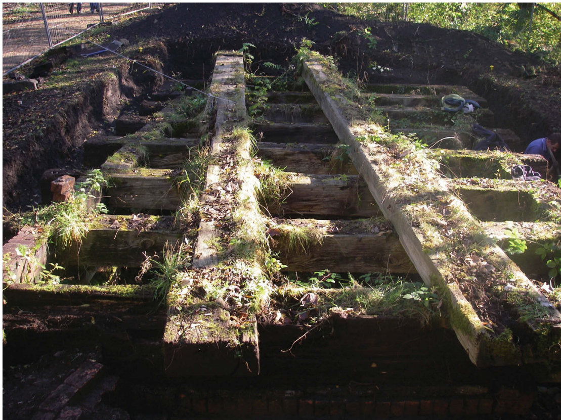
Plate 7: Wheel pit structure post-excavation, looking east
