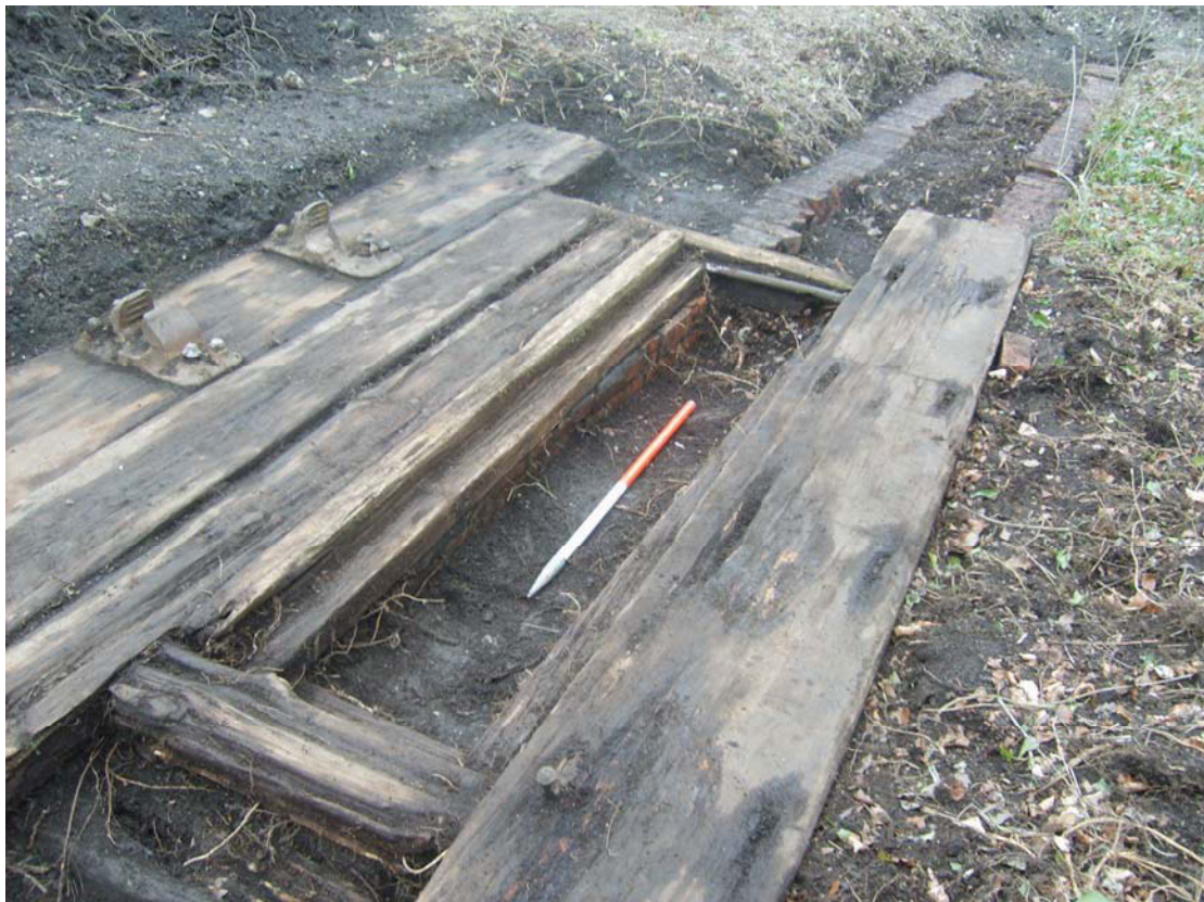
Plate 6: Gap in [304] where cable emerged from runnel; note brick runnel wall [308] running beneath timber. Looking north-east.
