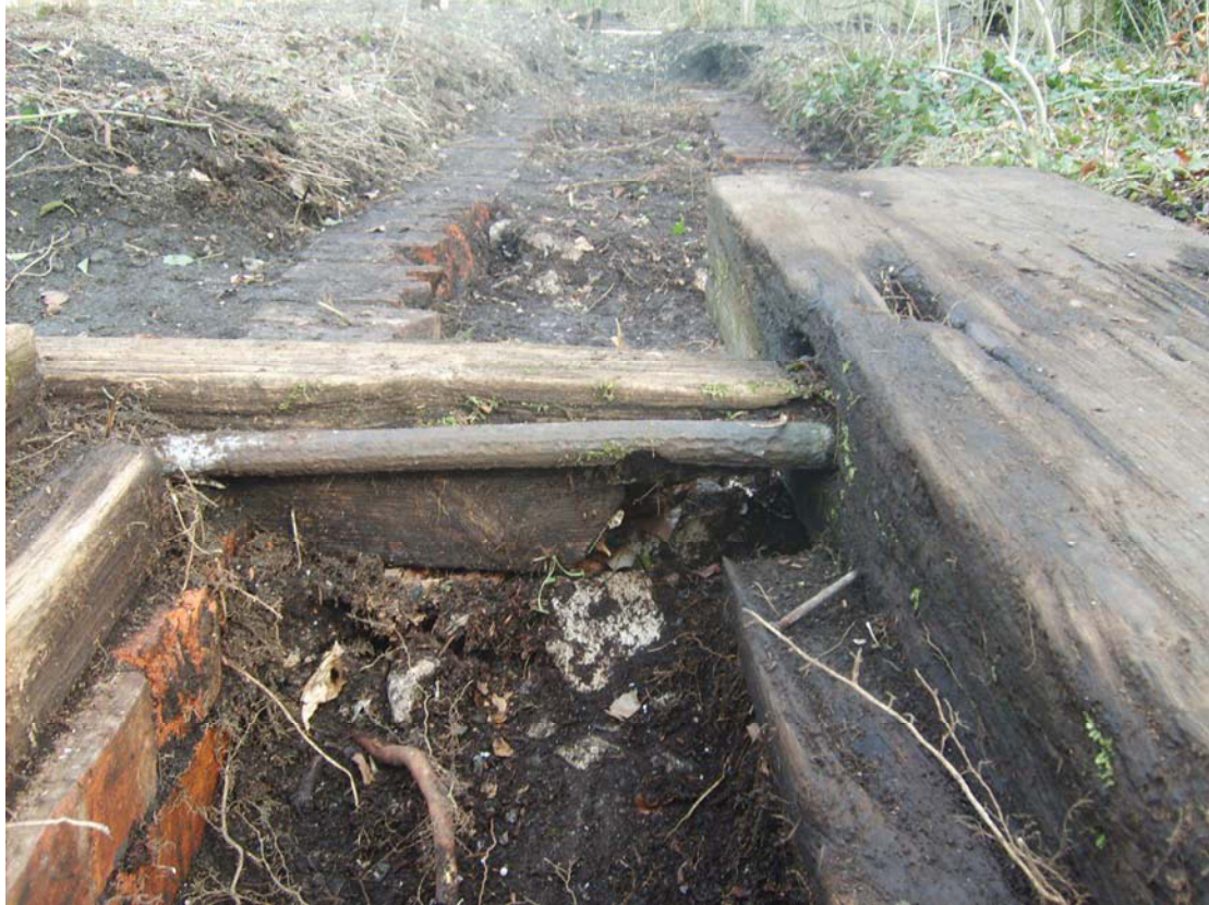
Plate 7: Steel reinforcing bar in [304], where cable emerged. Note semi-circular notch worked by steel cable.
