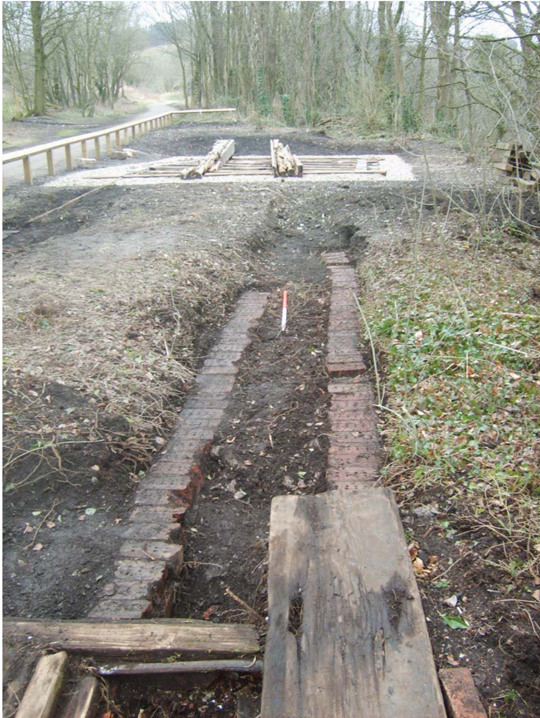
Plate 4: Southern cable runnel [307]/[308], looking east towards the wheel pit. Note timber structure [304] in foreground with steel reinforcing strut where cable emerged from runnel.
