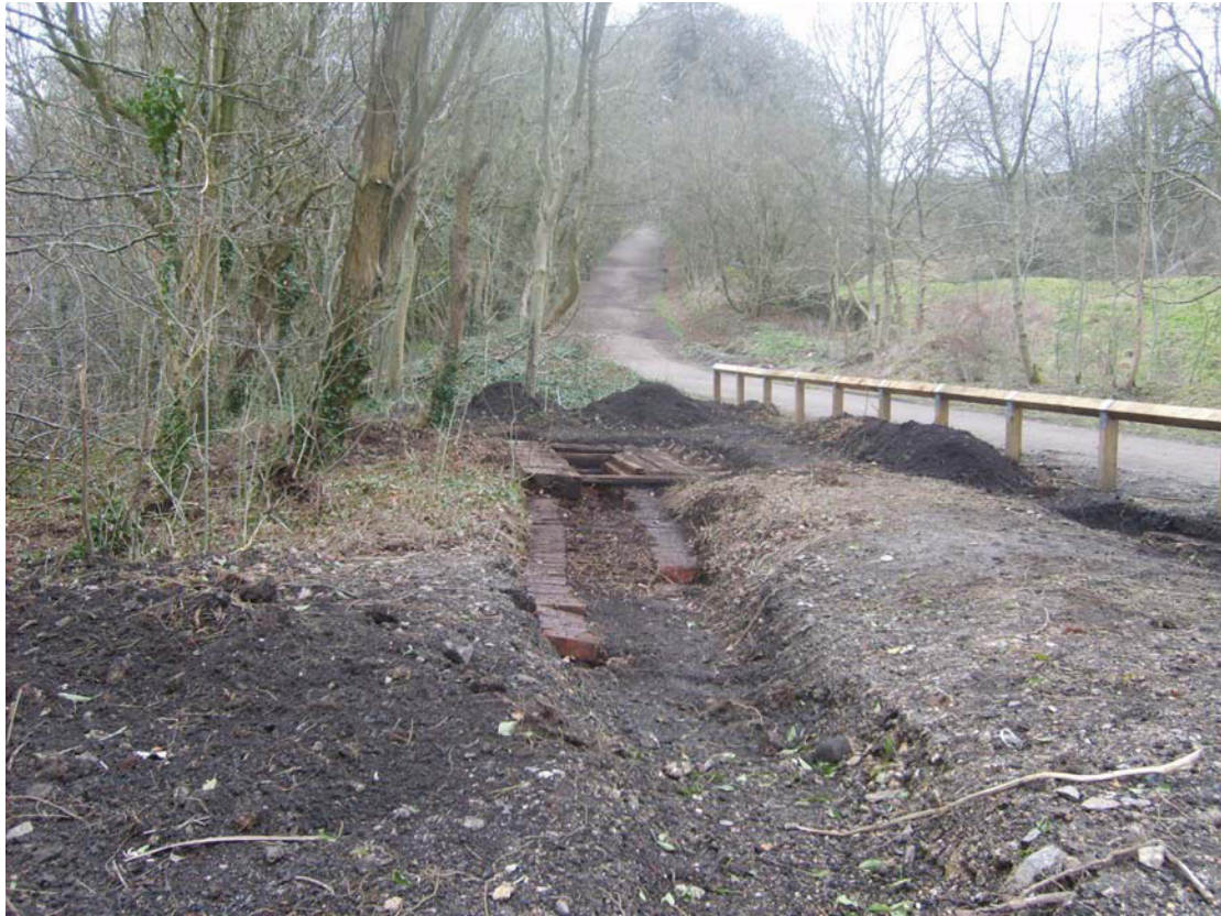
Plate 1: General view of southern cable runnel and timber structure [304], showing base of incline in background. Looking west.
