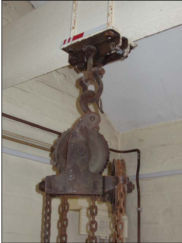
Plate 15 (27): Building A, room 2, feature [2] detail of the block and tackle fixed to the inserted joist (0.2m scale), looking west
