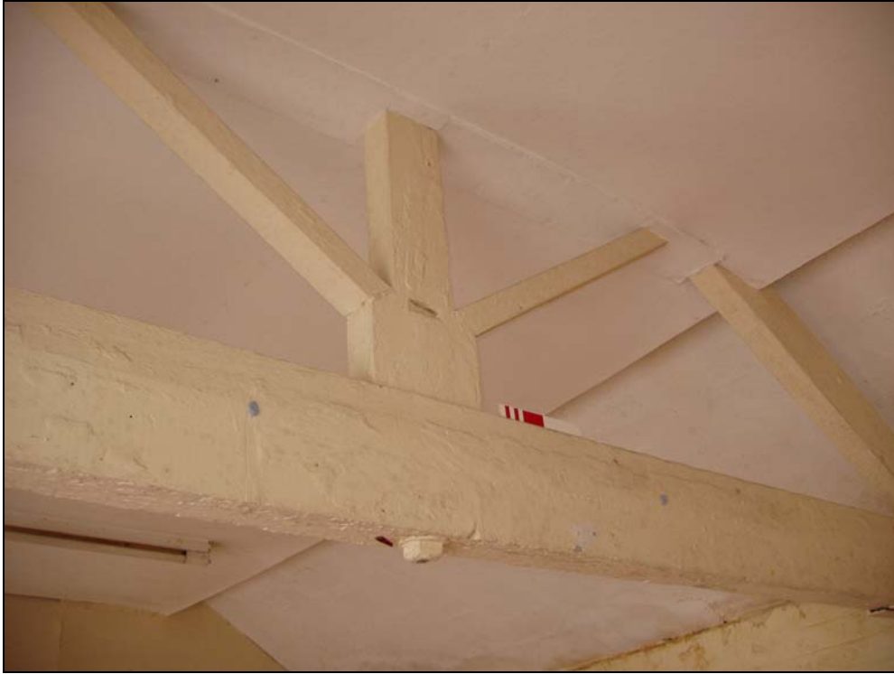
Plate 13 (26): Building A, room 2 detail of the semi-exposed king post truss [5], looking east
