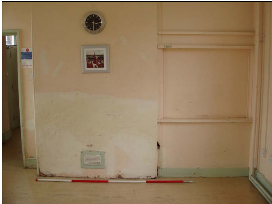
Plate 68: view of the south-west wall with blocked fireplace and inserted stud wall and large hatch, from the north-east
