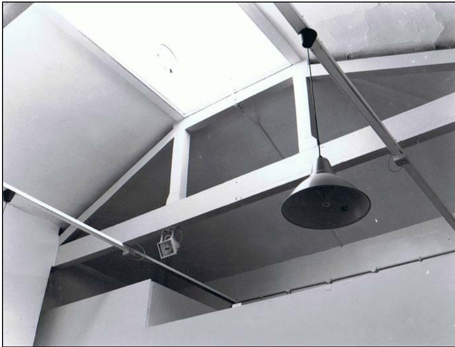
Plate 47: view of the queen post truss [37] (1 of 2), from the south-west
