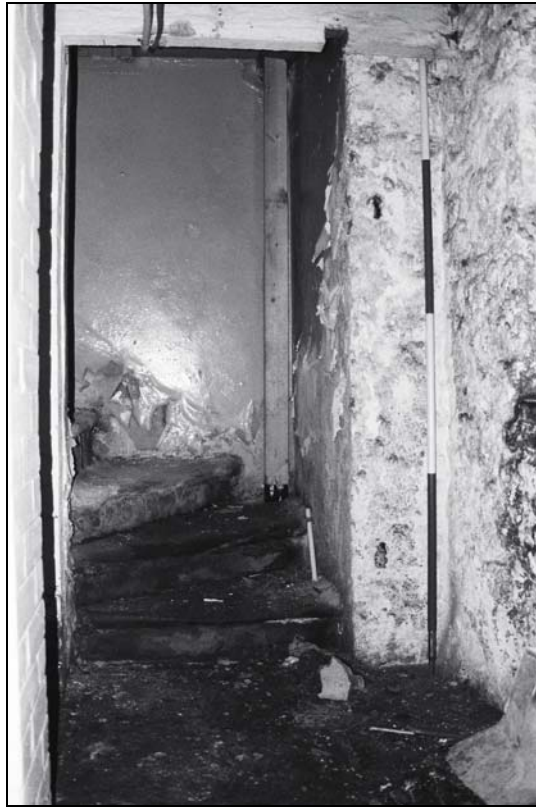
Plate 51: view of the lower staircase [38] with evidence for an internally hinged door, from the south-east
