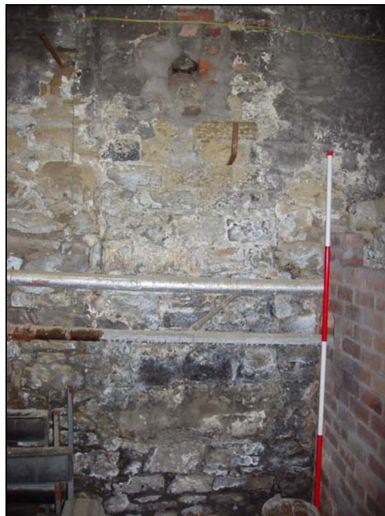
Plate 50: view of the blocked flue, from the south-west
