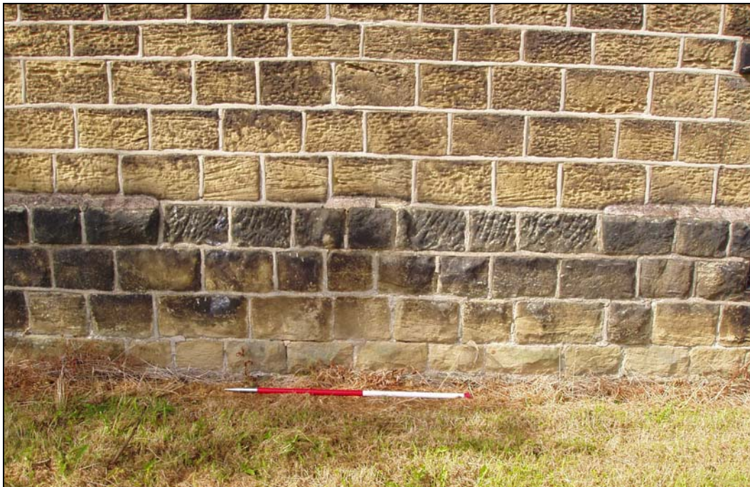
Plate 32: view of the chamfered plinth to the SE elevation of the SE Wing (Blg.3), from the south-east
