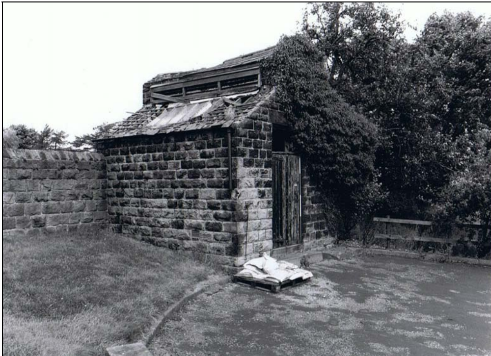
Plate 76: the gabled roofed mortuary house (Building 7) with a central ventilator and roof lights, from the south south-west
