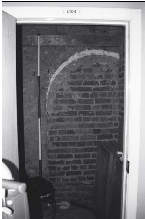
Plate 71: detail of the blocked arched probable stair window [53], from the north-west
