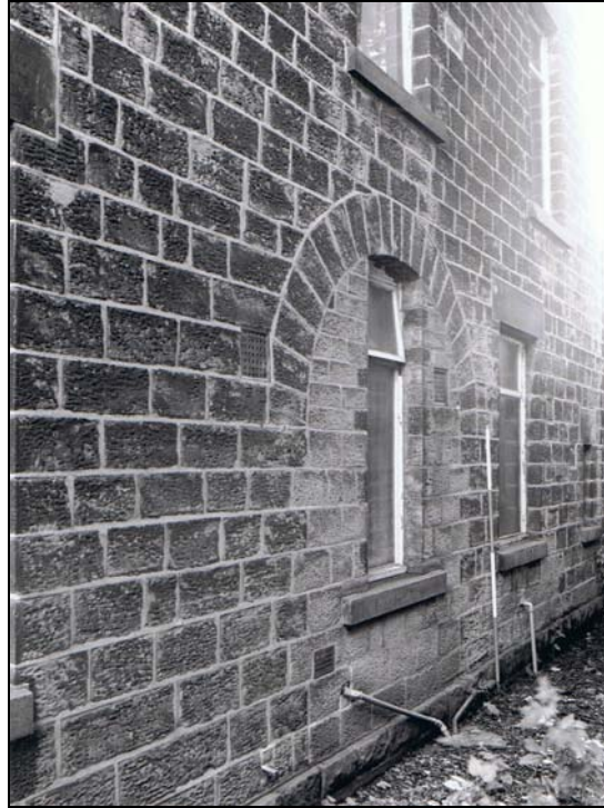
Plate 5: detail view of the blocked arched doorway [3] to the rear north-west elevation (Building 1), from the north-east
