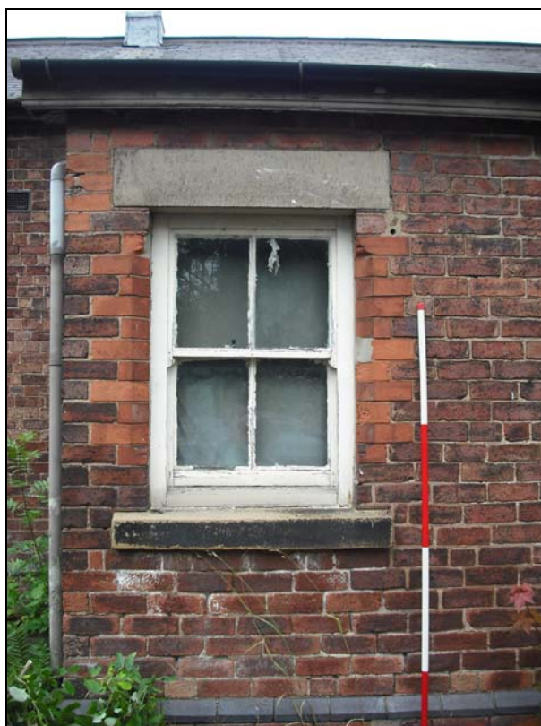
Plate 8, 17: an original 4-light sash window to the Entrance Lobby to the west elevation, from the west
