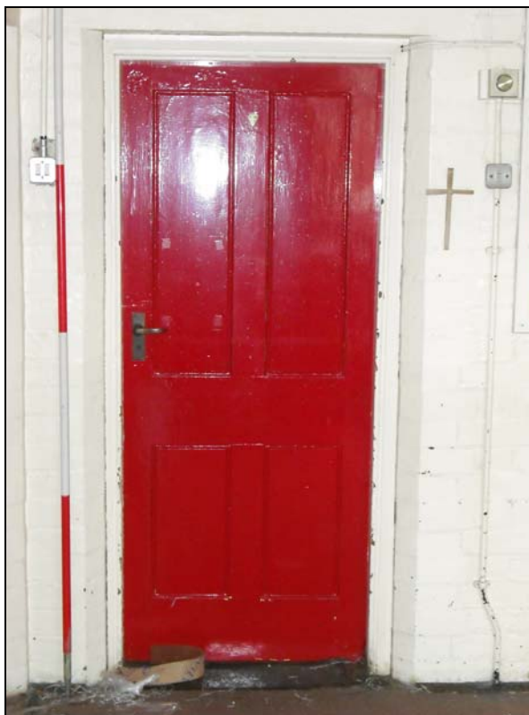
Plate 19, 26: Room 4 detail of the standard 4 panelled door with chamfered jambs, from the south
