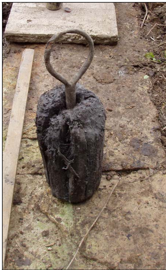
Plate 20: view of the drain plug removed from the dam's drain, looking northwest
