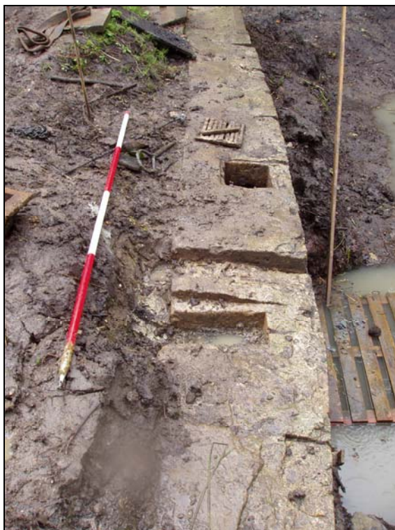
Plate 18: view of the dam wall (Site 2) with a small square access holes to the dam's drain and plug, looking south
