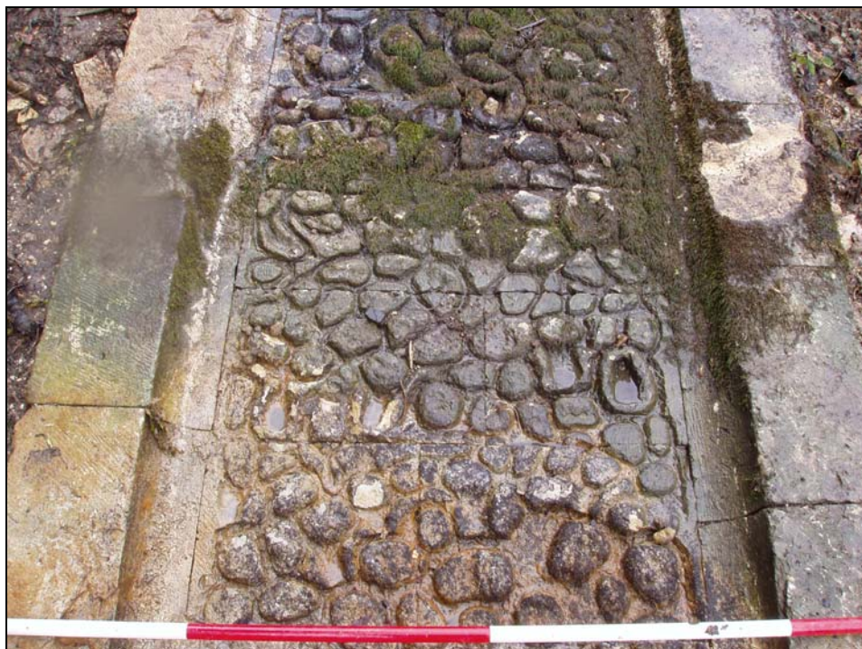
Plate 15: Site 2, detail of the carved pebbles and finely ashlared concave edges, looking southwest
