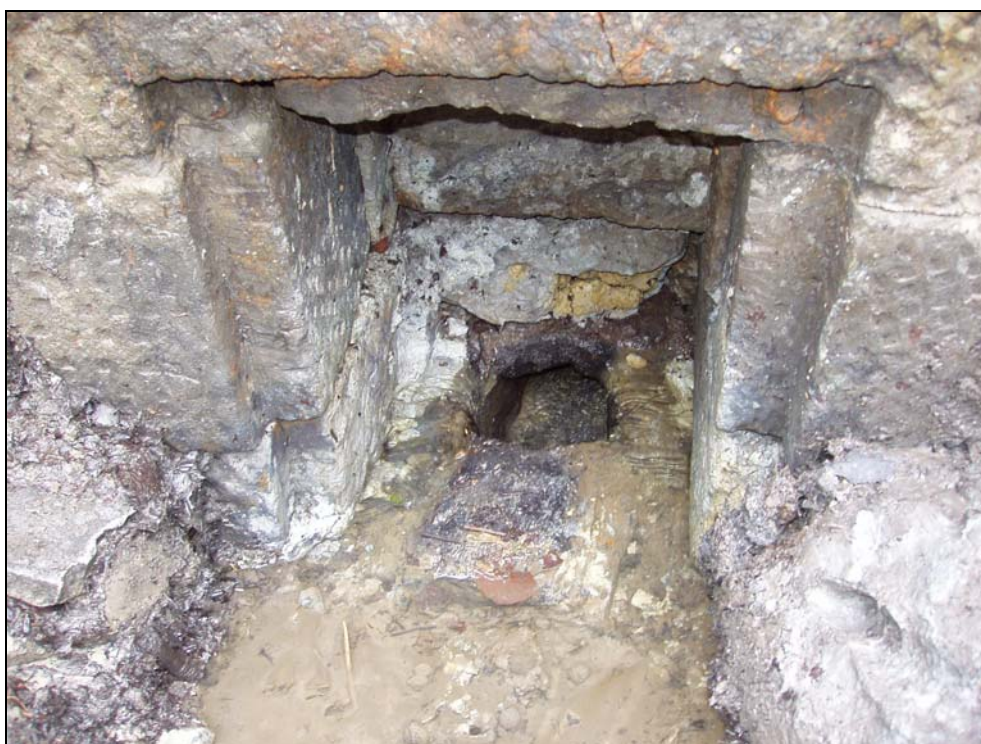
Plate 19: detail of the drain to the dam wall (Site 2) with grate removed, looking northeast
