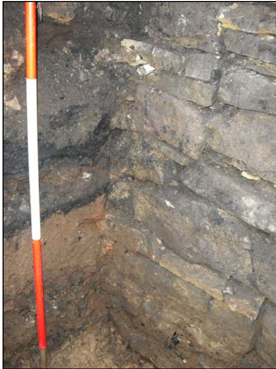
Plate 7: detail of the lower wall [123] and SE facing section, looking north
