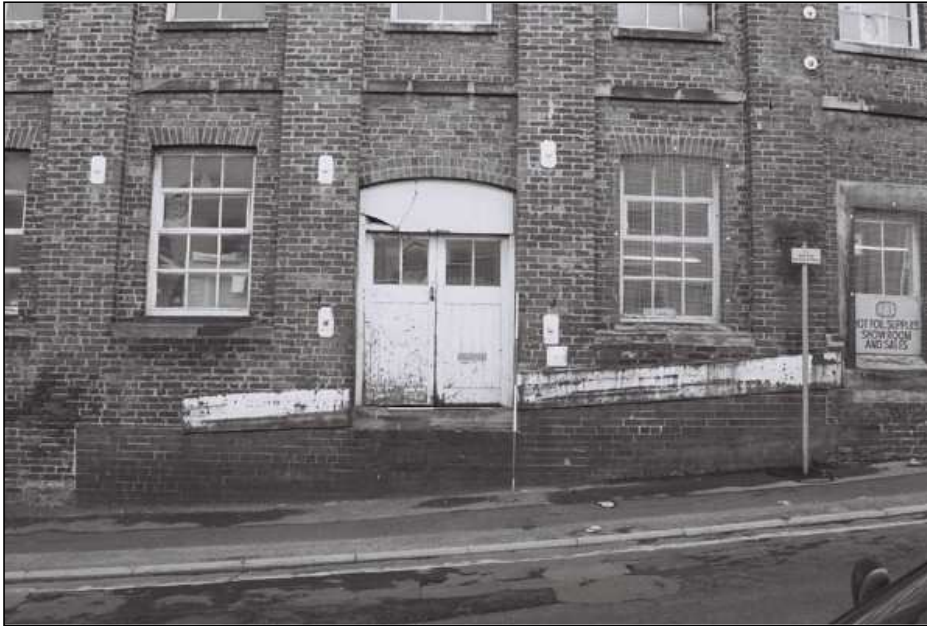
Plate 5: Taking-in door, building A, from Upper Allan Street, NW elevation, looking SE (film 001:18)
