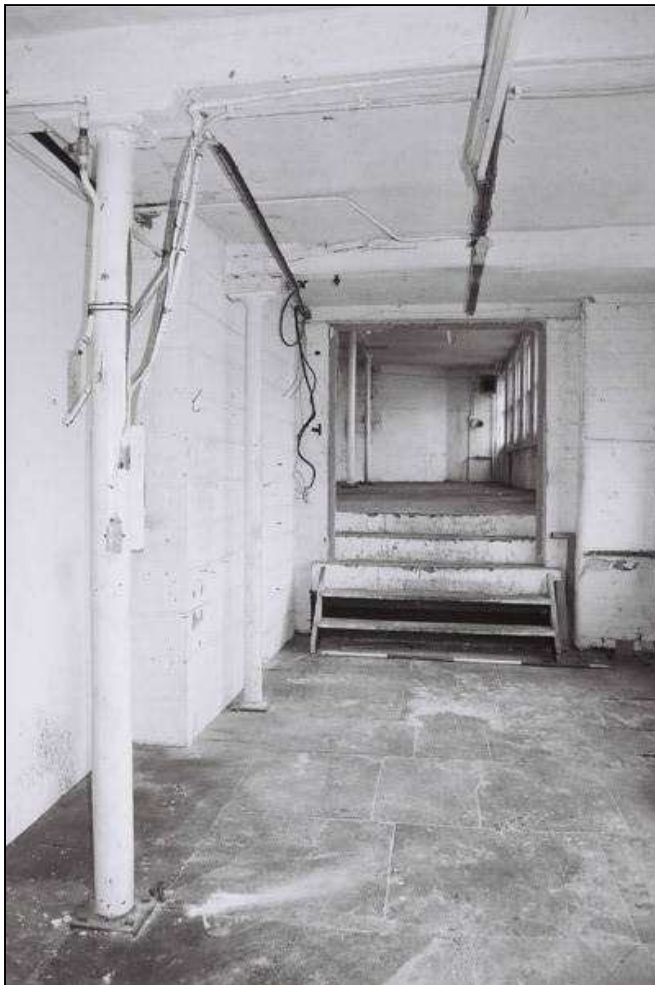
Plate 20: General shot from A20, through A21, showing columns, flagstone floor and change in floor height between buildings, looking SW (film 002/29)
