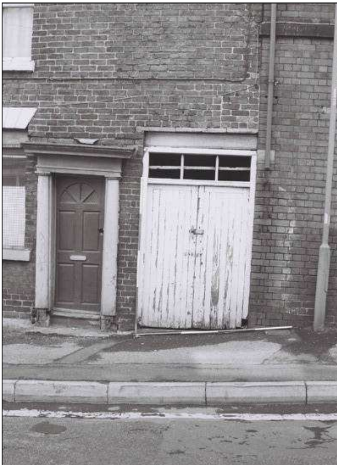
Plate 5: Taking-in door, building A, from Upper Allan Street, NW elevation, looking SE (film 001:18)
