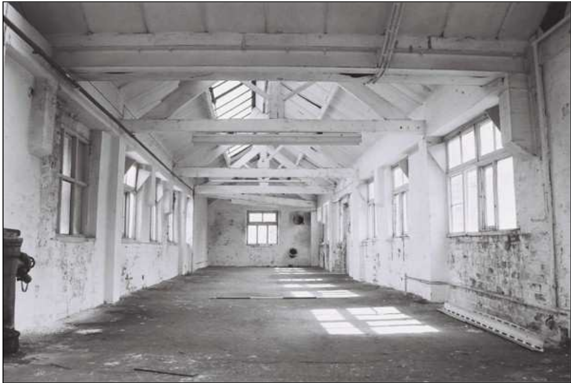
Plate 27: General shot, A32 (showing reused roof trusses), looking SE (film 002/15)
