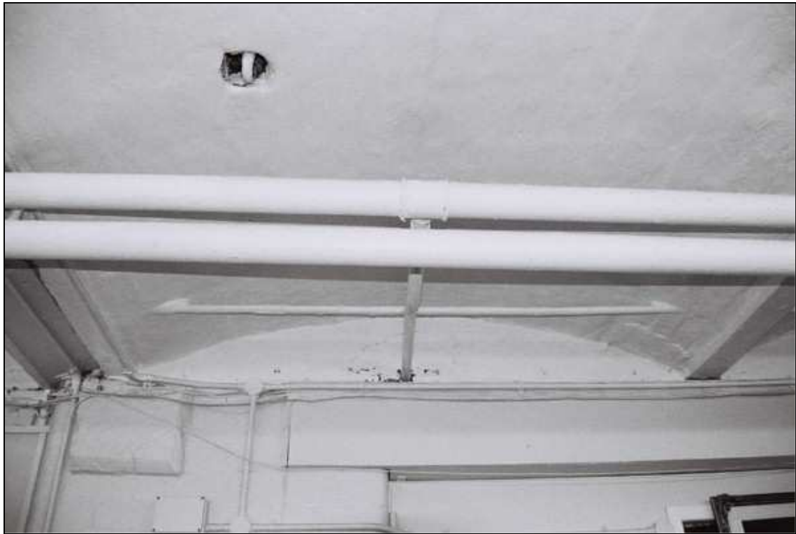
Plate 17: Detail of original brick jack arch ceiling with tie rod, A2, looking E (film 003/12)
