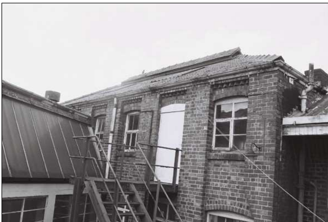
Plate 25: Exterior upper floor of A29/A30 showing hot working vent on roof, looking W (film 002/24)
