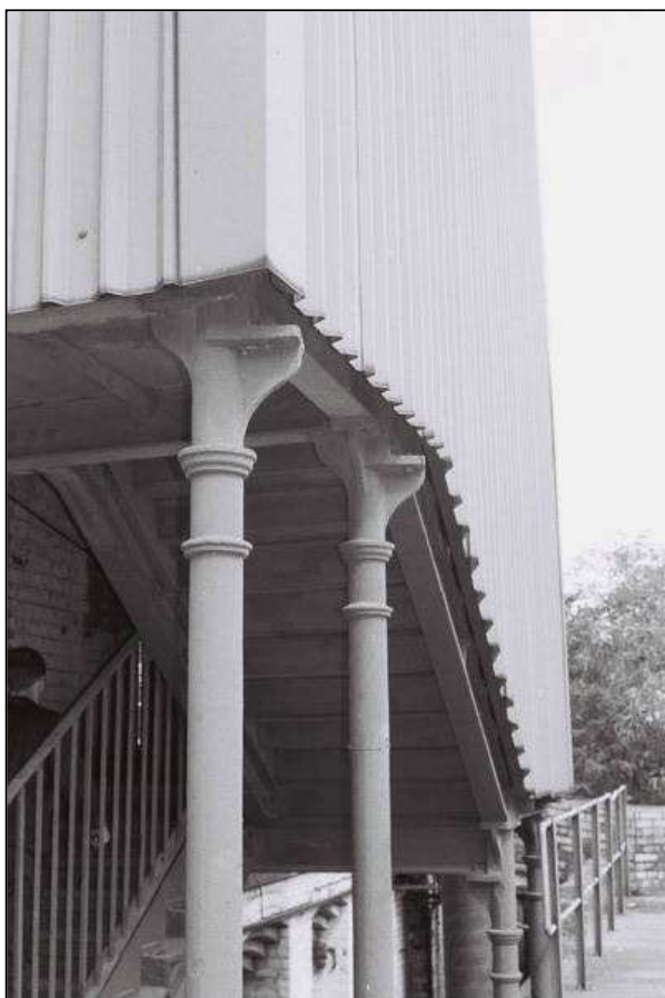
Plate 9: Columns at base of stair tower, note empty seating for removed walkway, looking N (film 002: 03)
