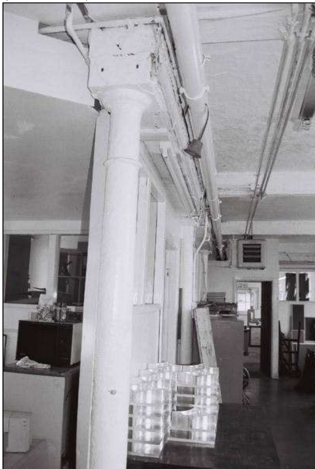
Plate 17: Detail of original brick jack arch ceiling with tie rod, A2, looking E (film 003/12)
