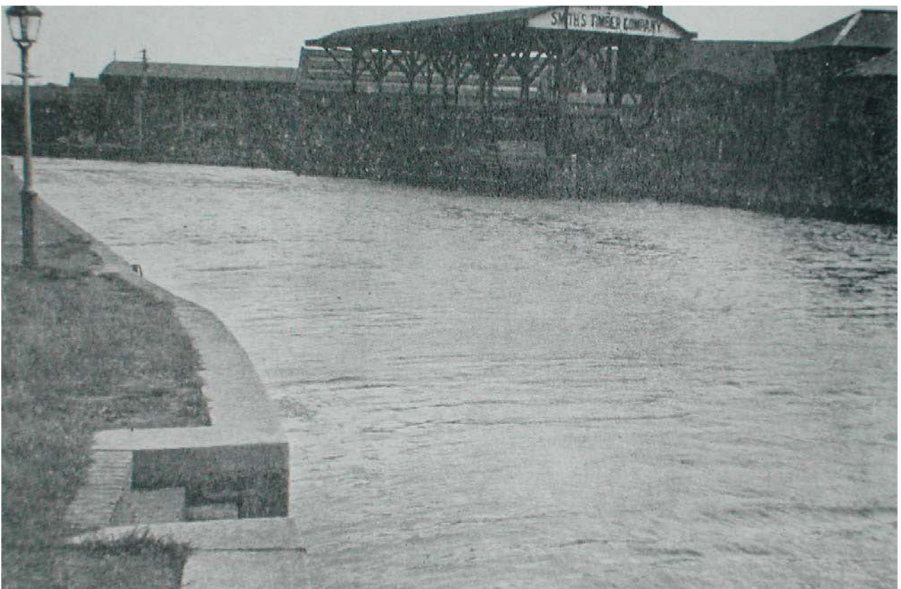
Plate 3.8: River Nene from South Bridge, Northampton after dredging. (River Nene Catchment Board)
