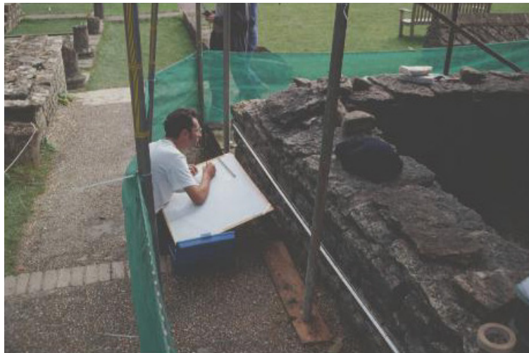
Detailed recording of masonry in the West Wing
