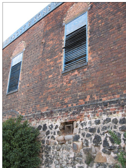
The former premises of the metal processing company Frost & Sons (Moxley) Ltd next to the Walsall Canal, established in the 19 th century (HBL5148). This view shows iron slag used in the construction of the building. While this part of the five hectare site now appears to be disused, the remainder is still an active location for the steel manufacturer Wesson W Glynwed Steels Ltd .
