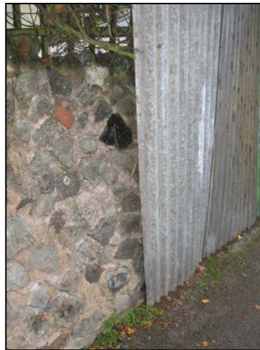
Left: Like the products of the brick industry, local iron (and later steel) works provided materials which became literally embedded in the landscape of the Black Country. Here an iron-slag wall in Smethwick has been repaired using corrugated iron (HBL12014).
