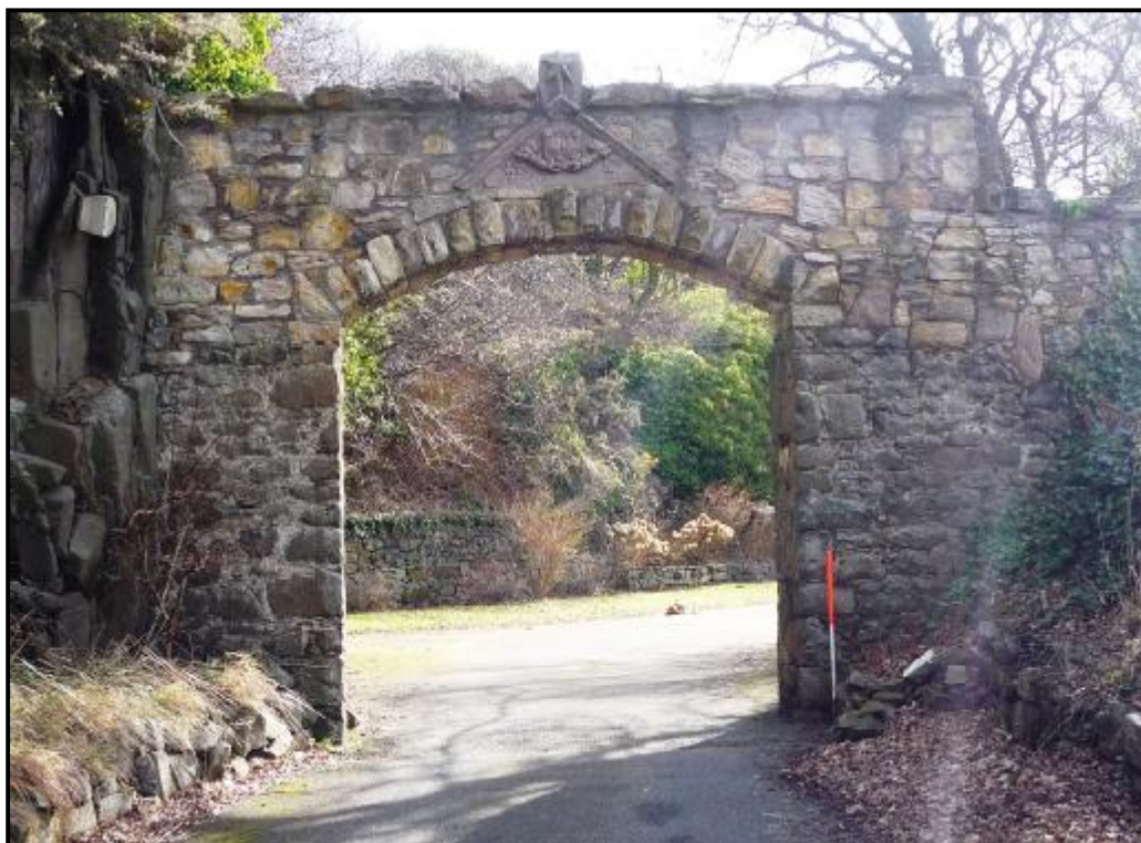
Plate 1: The archway, west facing elevation: from west.
