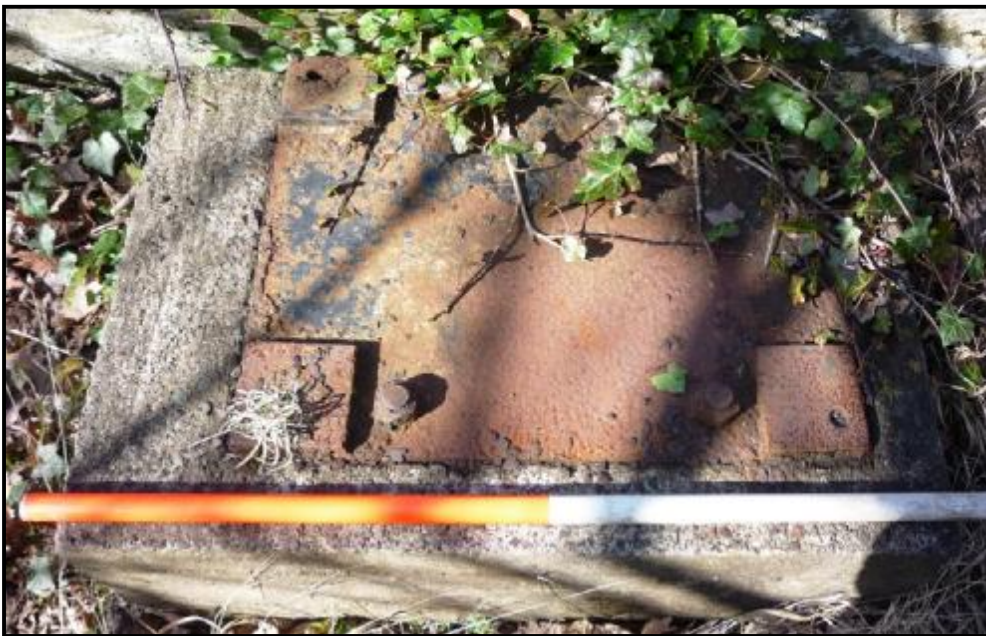
Plate 9: Detail of Signal Lamp base: from south.
