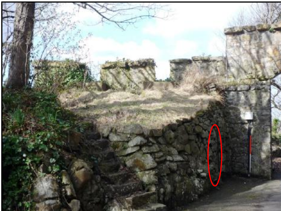
Plate 7: Embankment and crenulations and the location of the gate bar (circled): from north-east.
