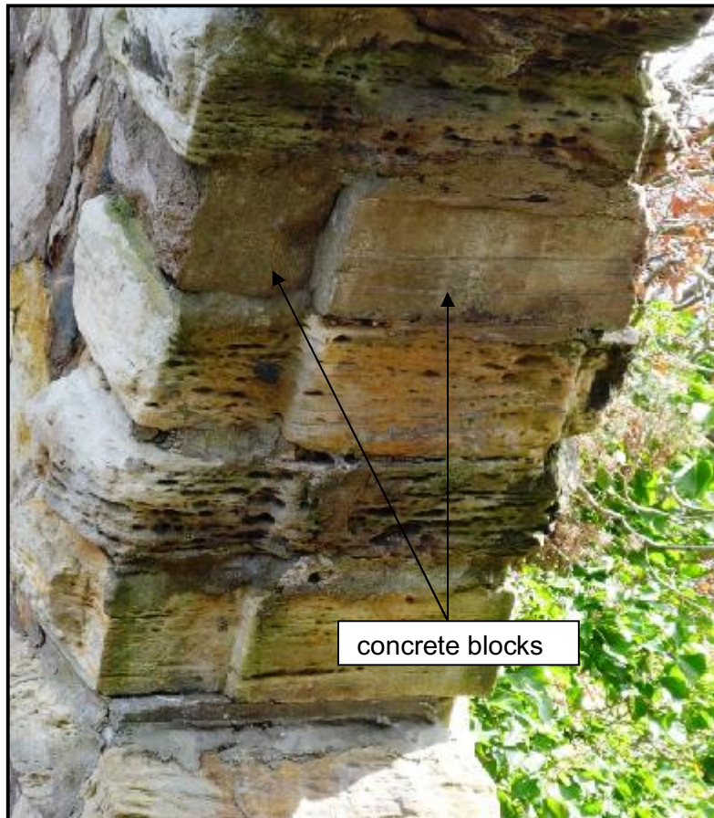
Plate 6: Detail of gate rebate: from South-west.
