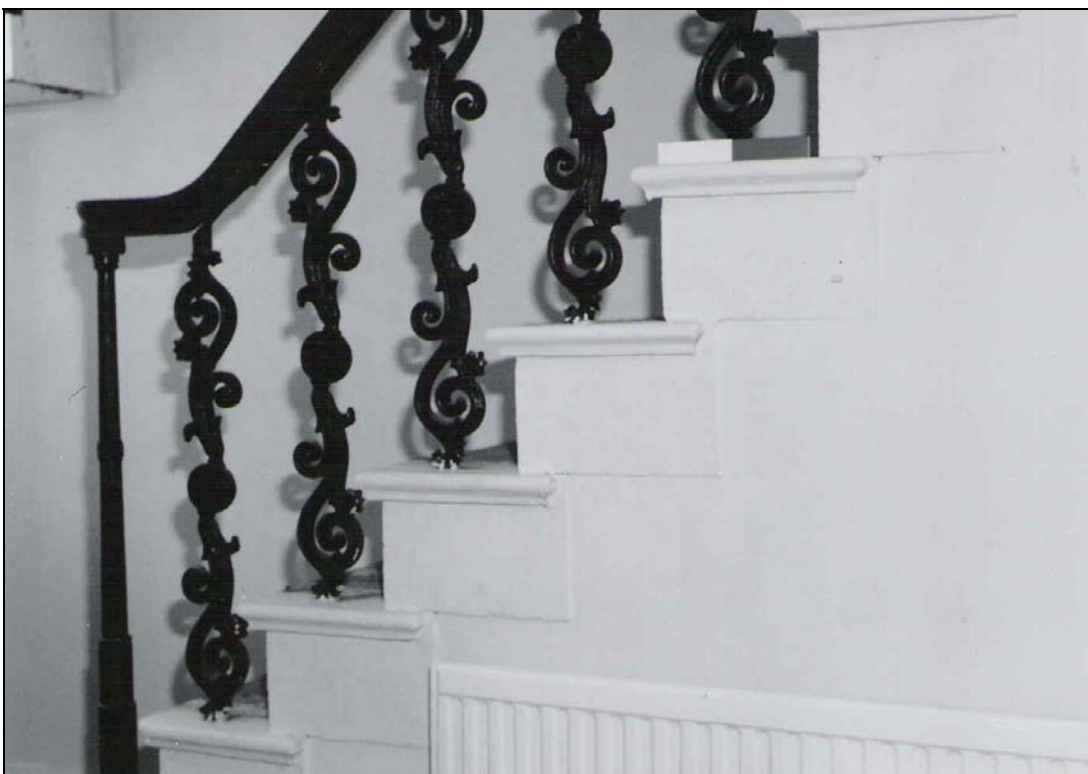
Plate 38: Ornate cast iron balustrade to stone stairs in Lodge
