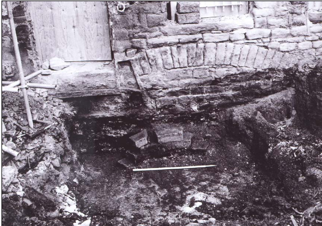
Plate 9: Location shot of arch in south end of east elevation of main building
