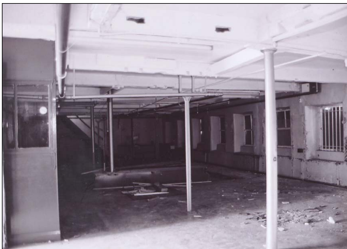
Plate 14: Ground floor looking south-west
