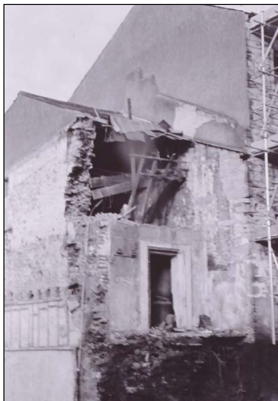
Plate 2: East elevation south building
