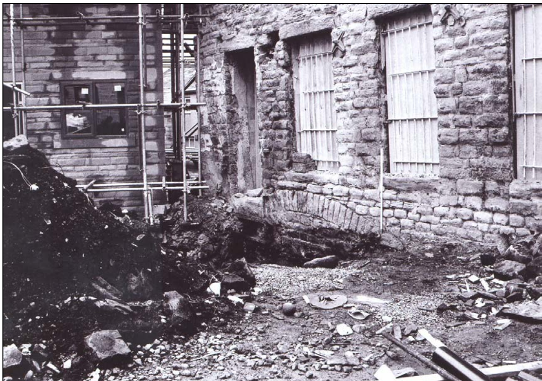
Plate 10: Arch in south end of east elevation of main building
