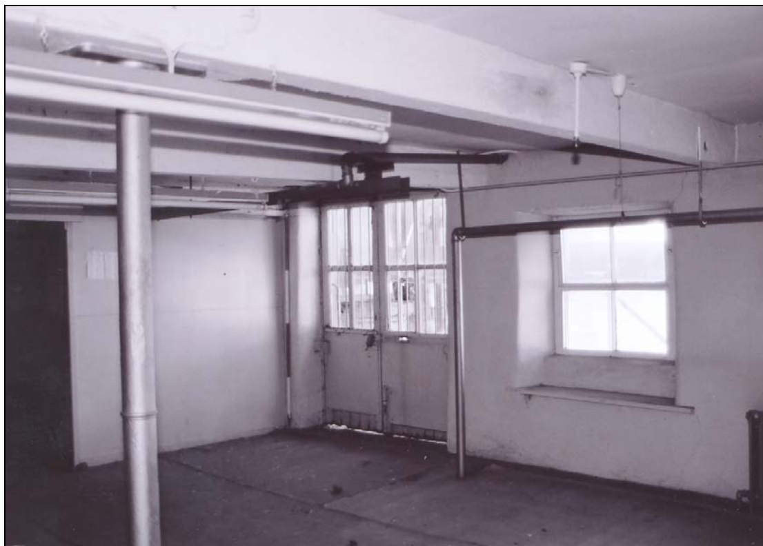
Plate 19: Loading doors first floor
