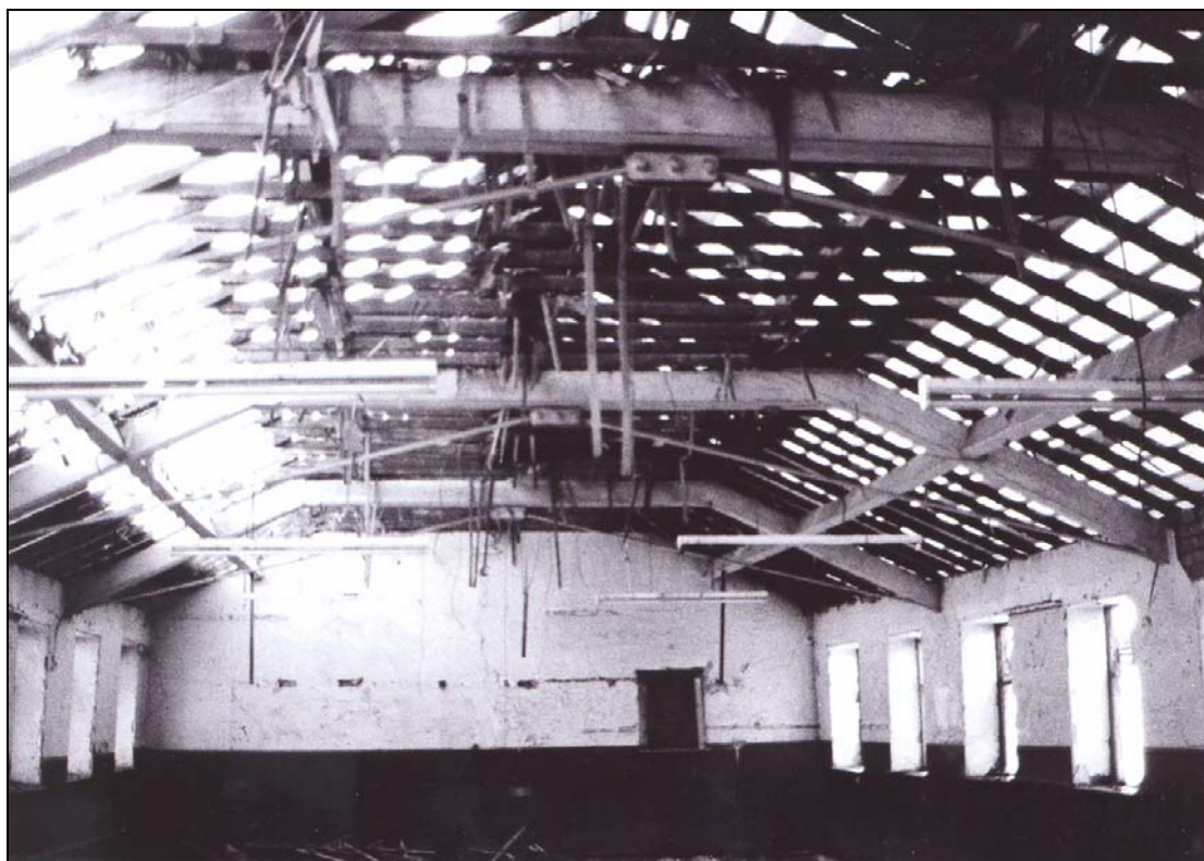
Plate 22: Roof timbers second floor
