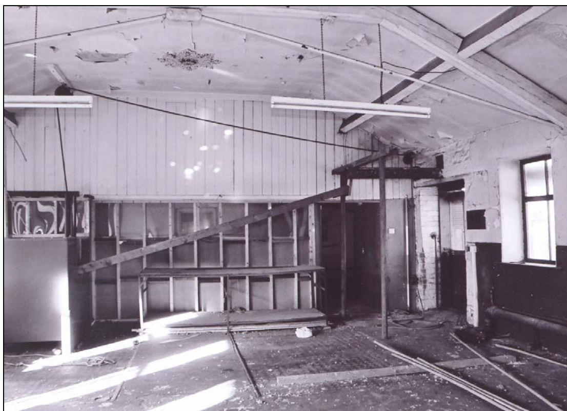
Plate 23: Loading doors and hoist second floor
