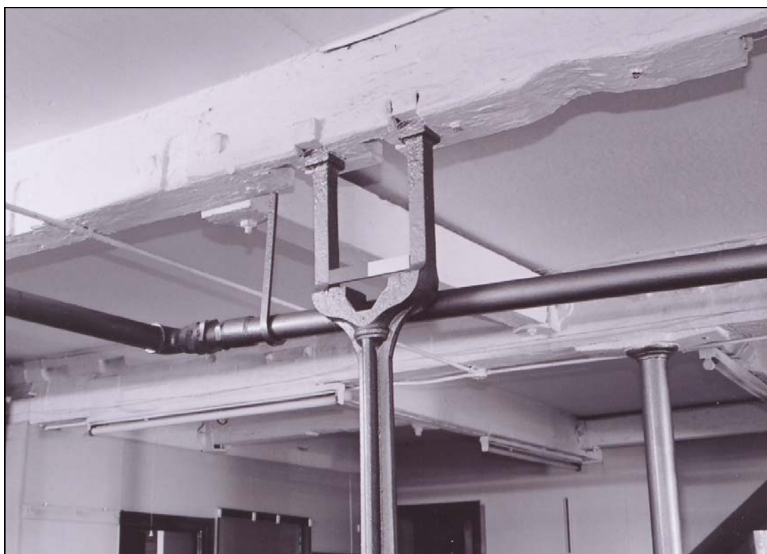
Plate 16: Type B stanchion ground floor
