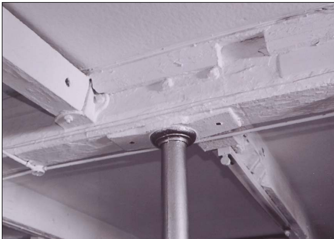
Plate 17: Type A stanchion ground floor
