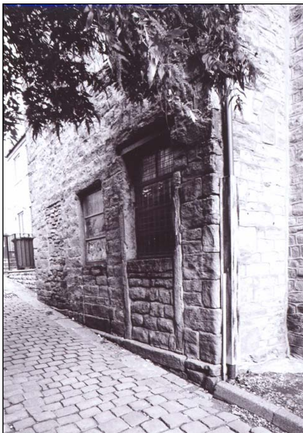
Plate 5: Blocked doors in north building
