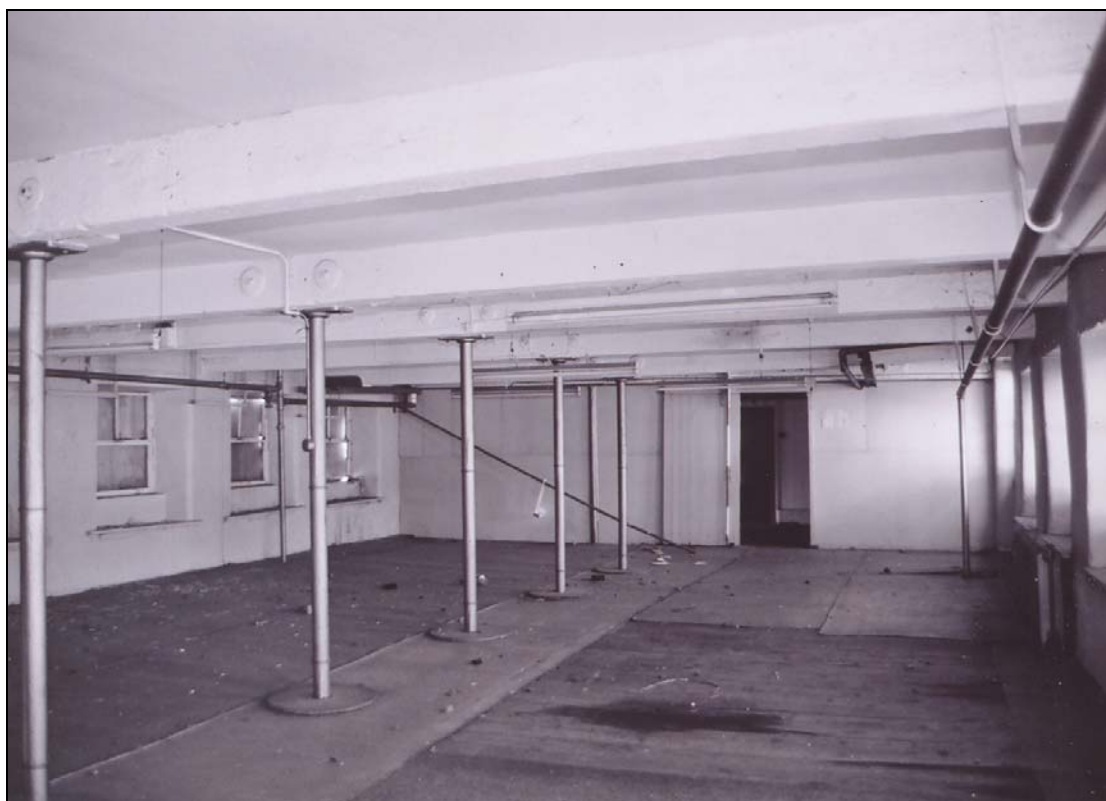
Plate 18: First floor looking north
