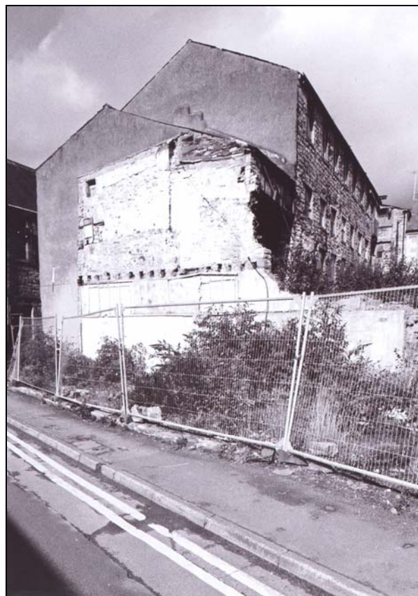
Plate 12: Former roof line of south building
