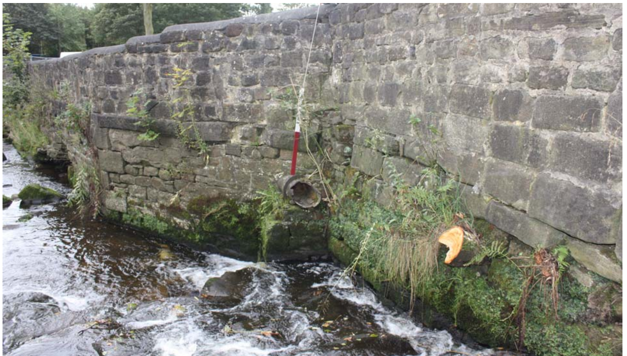
Plate 26: Right bank of Weir 2. Protruding iron pipe marks the foot of the weir
