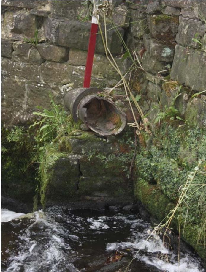
Plate 27: Detail of protruding iron pipe at foot of Weir 2.
