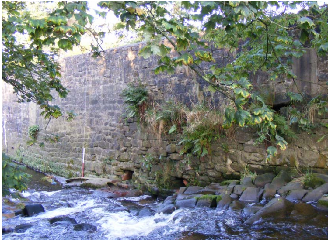
Plate 15: Random and tooled stonework in right wall; coursed beyond foot of Weir 1
