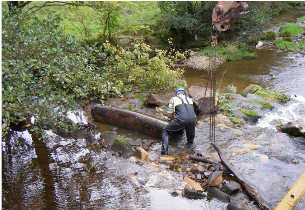
Plate 22: Pipes being removed from lip of Weir 2
