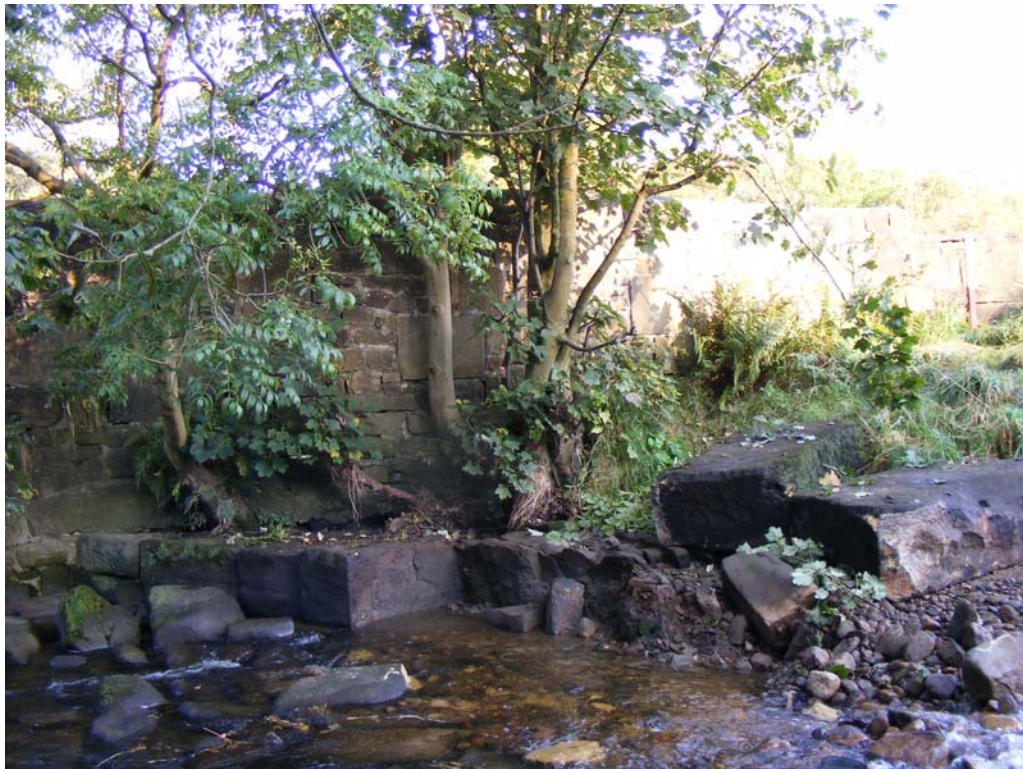
Plate 9: Flanking blocks still in place on right bank after lip has been removed
