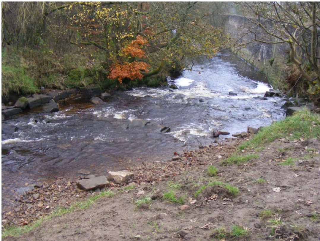
Plate 4: Weir 1 looking downstream after removal of lip (flanking blocks still in place)
