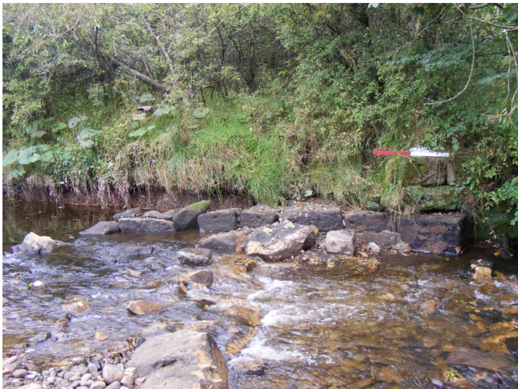
Plate 8: Flanking blocks still in place on left bank after lip of Weir1 as been removed
