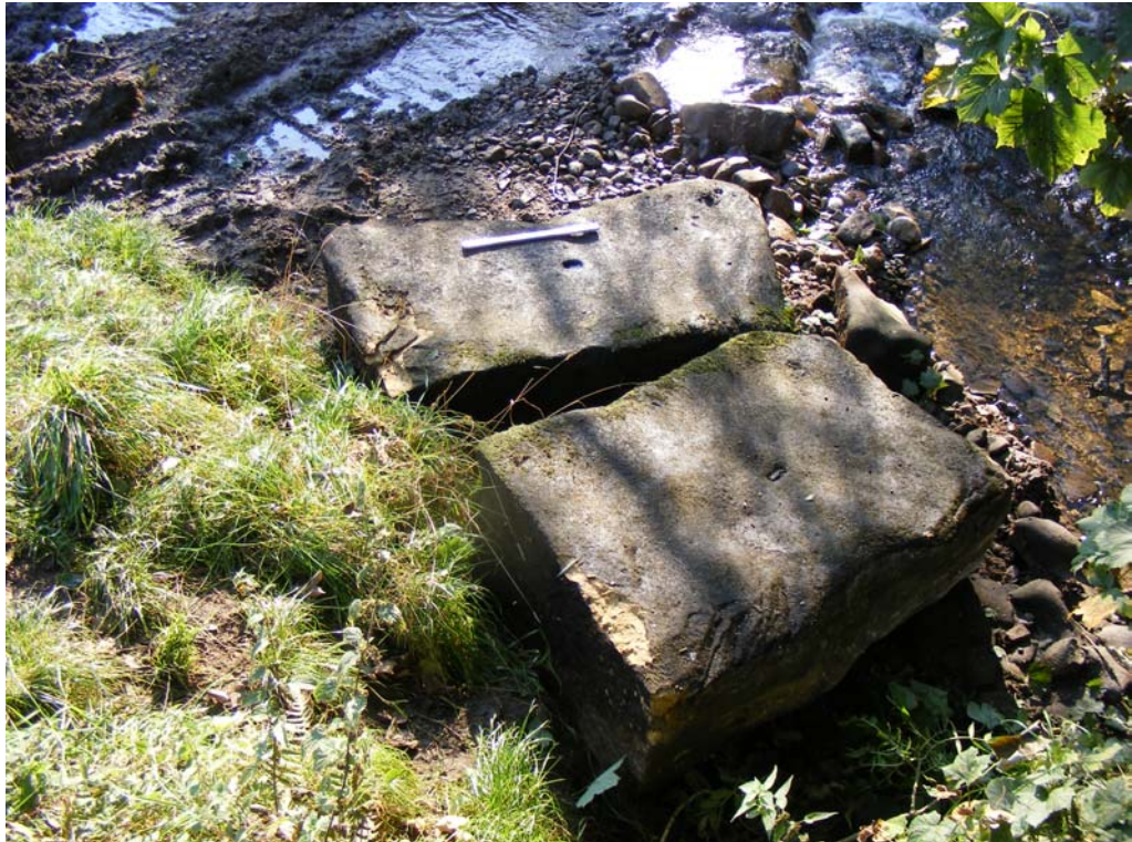
Plate 10: Central blocks after removal from Weir1. NB wedge shape and Lewis Holes
