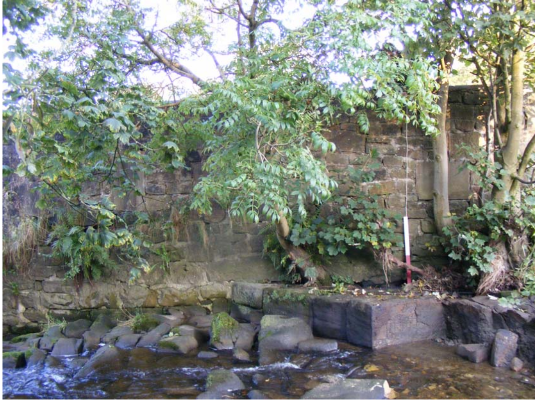
Plate13: Right retaining wall above lip of Weir1. Stonework changes at the large block
