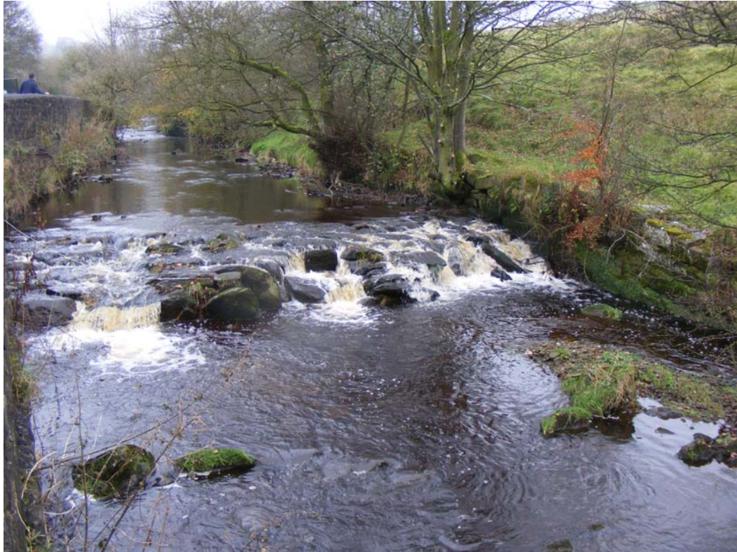
Plate 29: Looking upstream at Weir 2 after removal of pipework on lip
