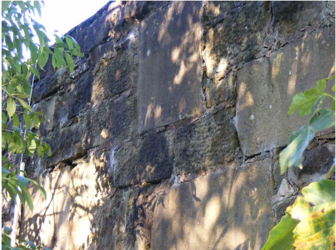
Plate14: Tooled stonework in upper part of right wall above lip of Weir 1.
