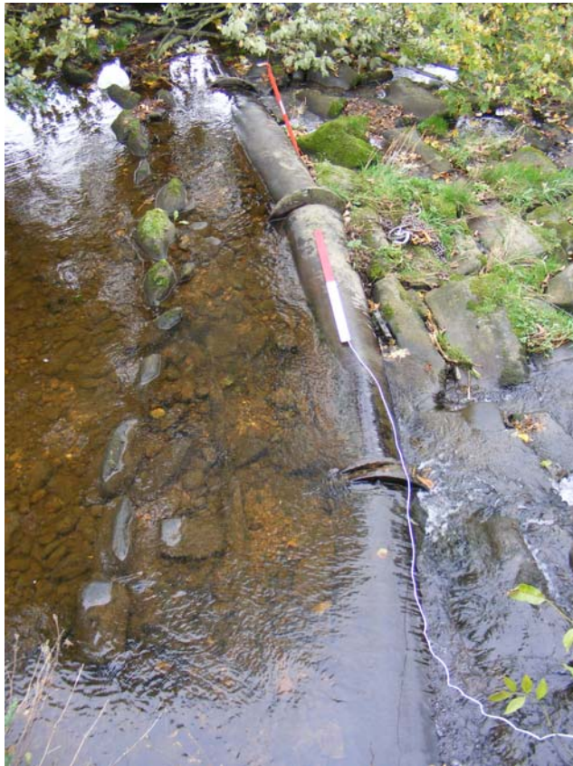
Plate 21: Pipework forming lip at head of Weir 2
