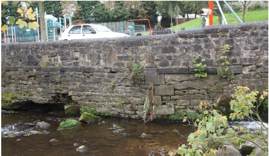
Plate 28: Detail of undercut wall below foot of Weir 2.
