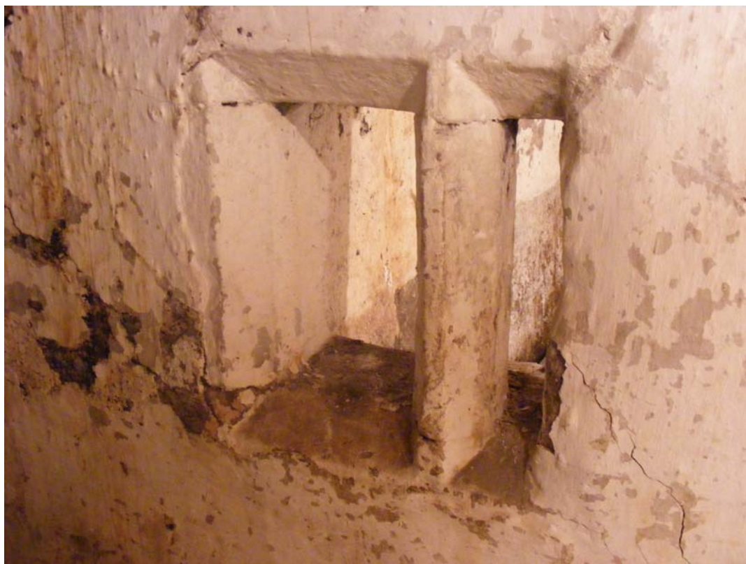
Plate 30: Detail of mullioned window in wall between room 6 and passage 5 from passage 5
