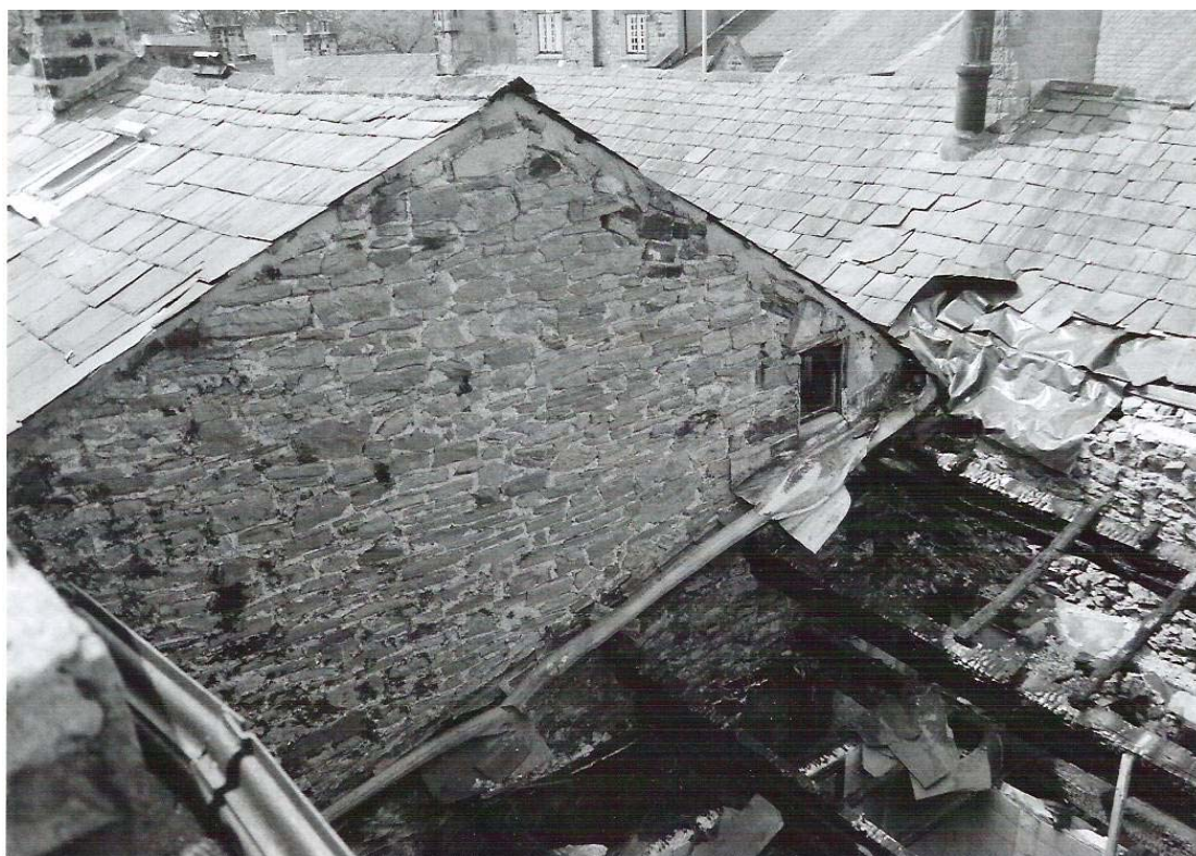
Plate 5: Roof and north wall of east pile of Inn with burnt out lean-to in foreground
