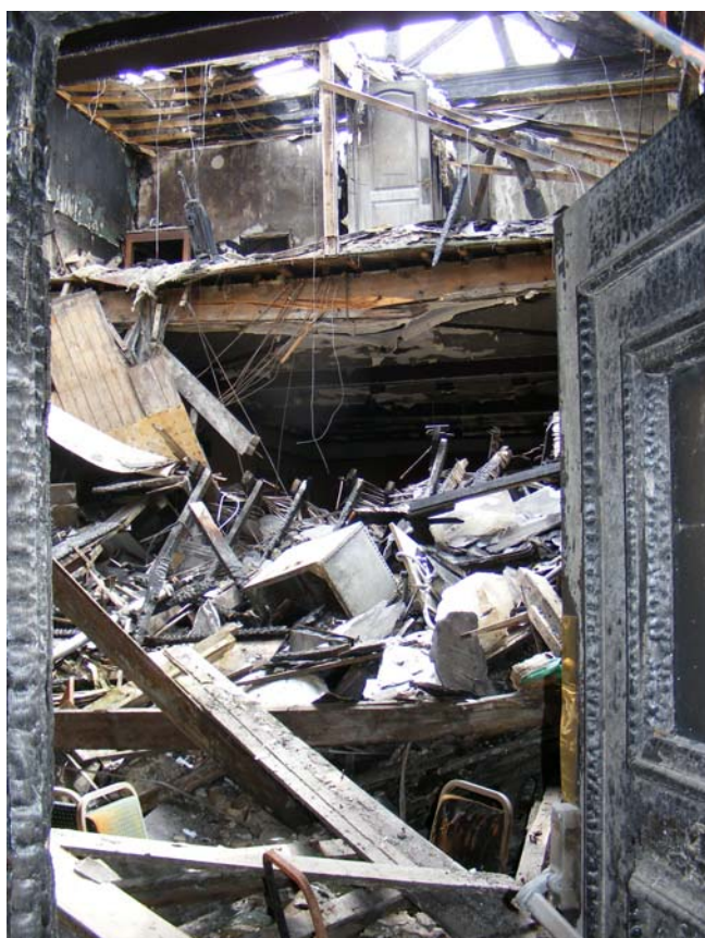
Plate 40: View of debris in function room and remains of 2 nd floor above viewed from stairwell
