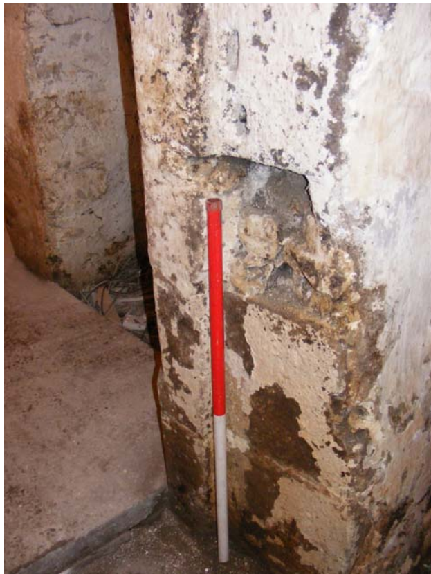
Plate 32: Receiving hole for bar in doorway between room 6 and passage 5
