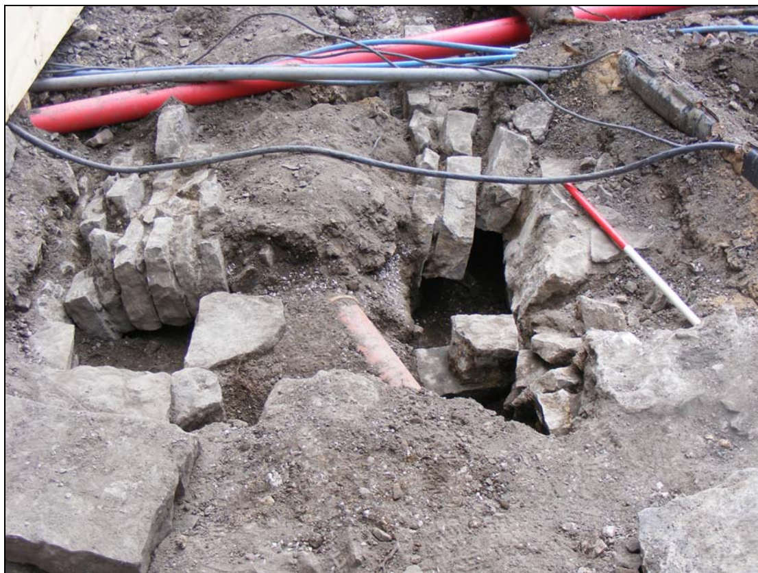
Plate 61: Vaulted roof over cavity
