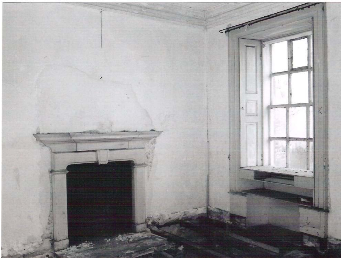
Plate 45: North west first floor bedroom: original stone chimney piece on west wall and window with panelled soffit and jambs in north wall
