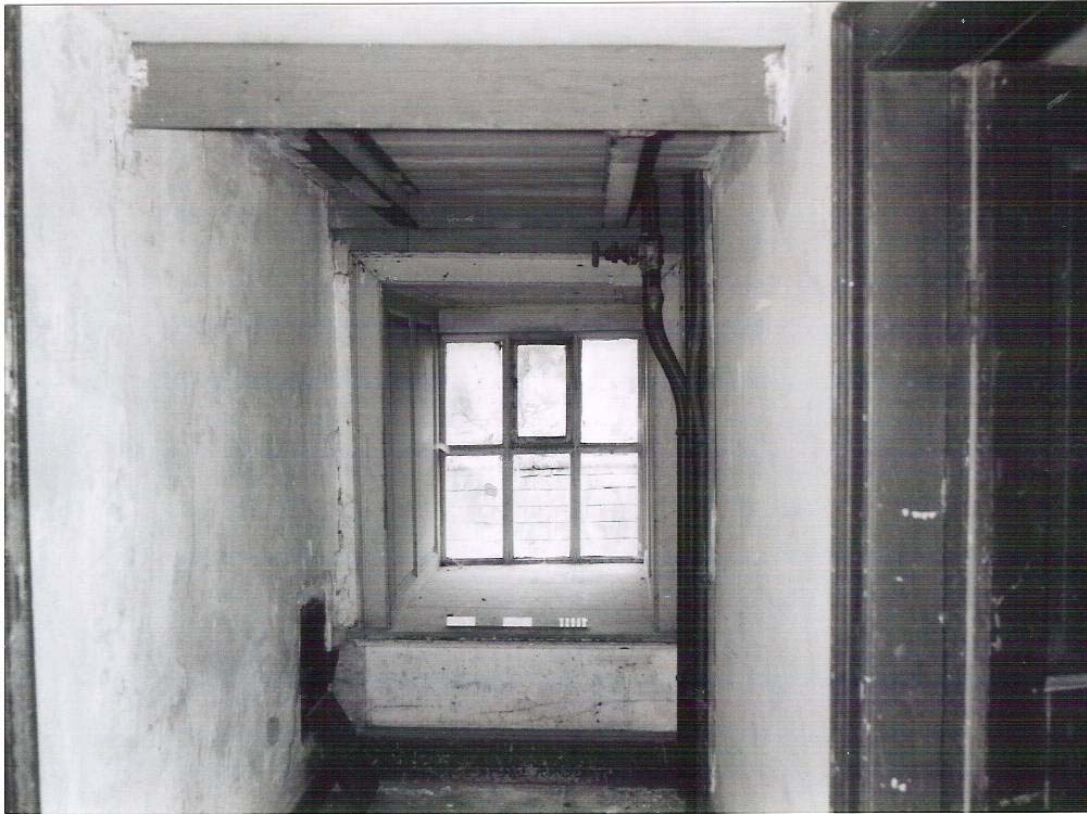
Plate 49: Deep window with ash chute in left wall at west end of attic corridor
