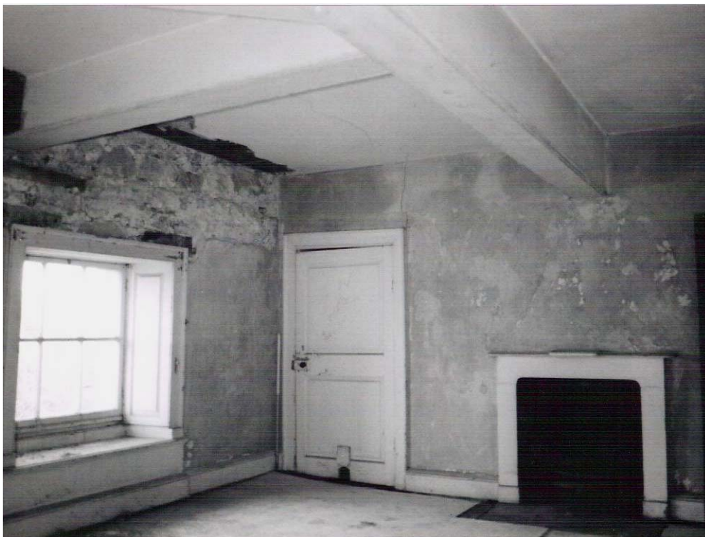
Plate 48: North-east attic bedroom: original fireplace and fielded panel door on south wall and window with panelled soffit and jambs in east wall
