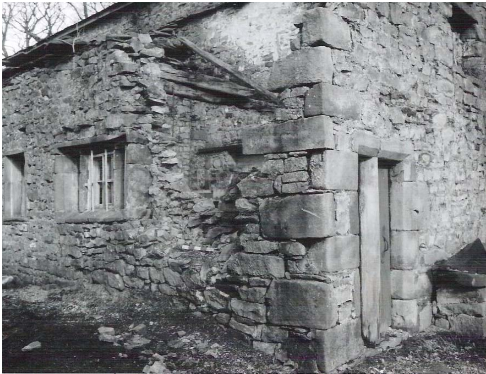
Plate 63: 17 th century mullioned window in south elevation of barn
