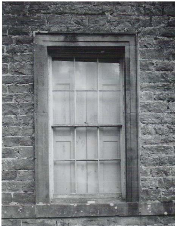
Plate 8: Window on ground floor of south elevation with moulded surround and cill with vertical toolmarks
