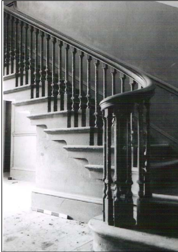
Plate 33: Open string staircase
