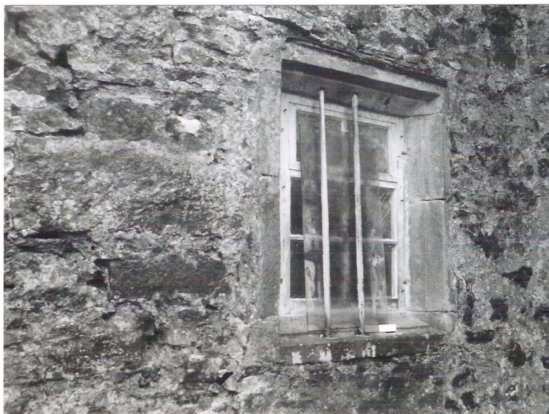
Plate 62: Reused 17 th century window with recessed chamfered surround in south wall of outshot
