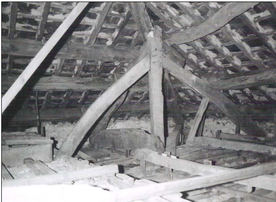
Plate 50: North west hipped corner to roof of main house
