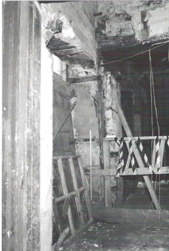
Plate 15: Original service doorway in north wall converted to window
