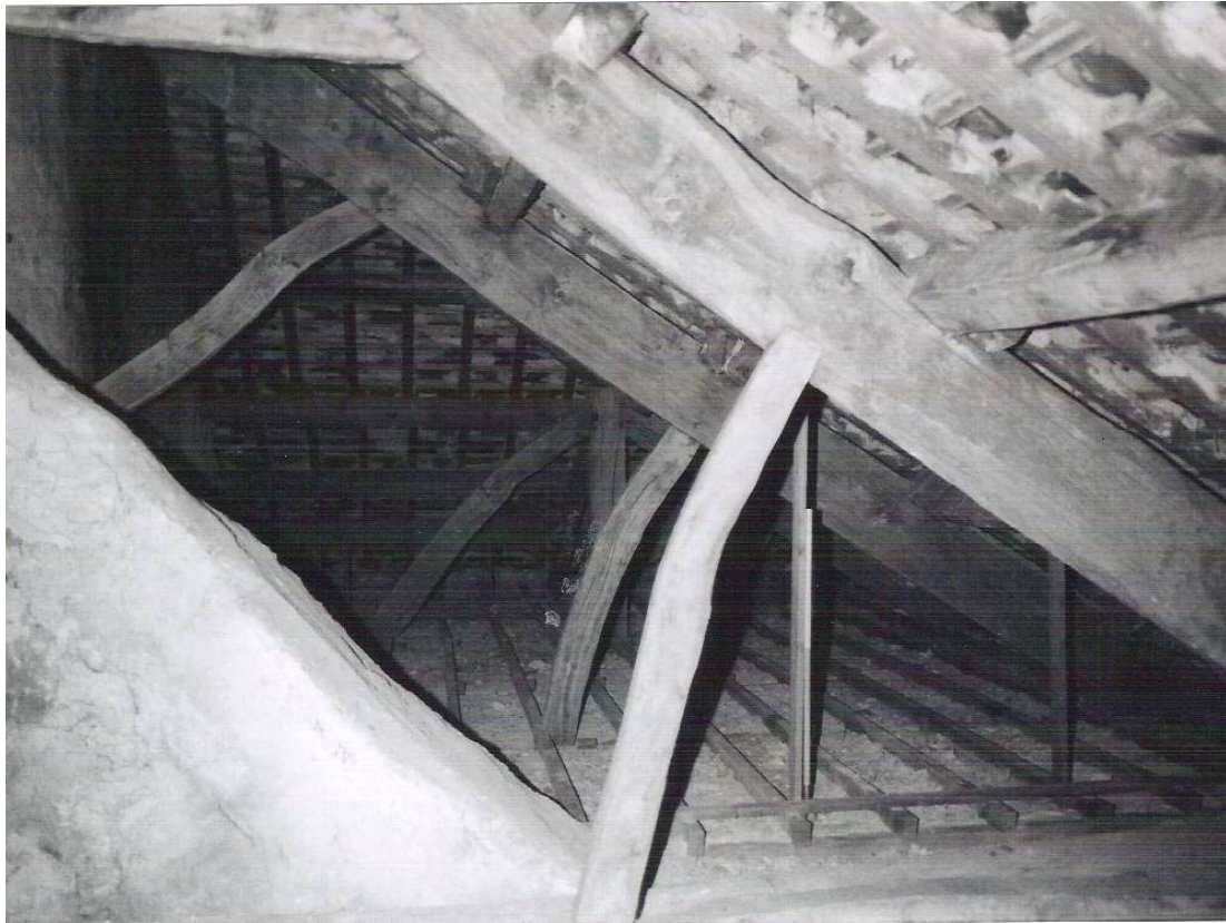
Plate 51: Principal rafters with curved strut looking east along south pitch of roof to main house
