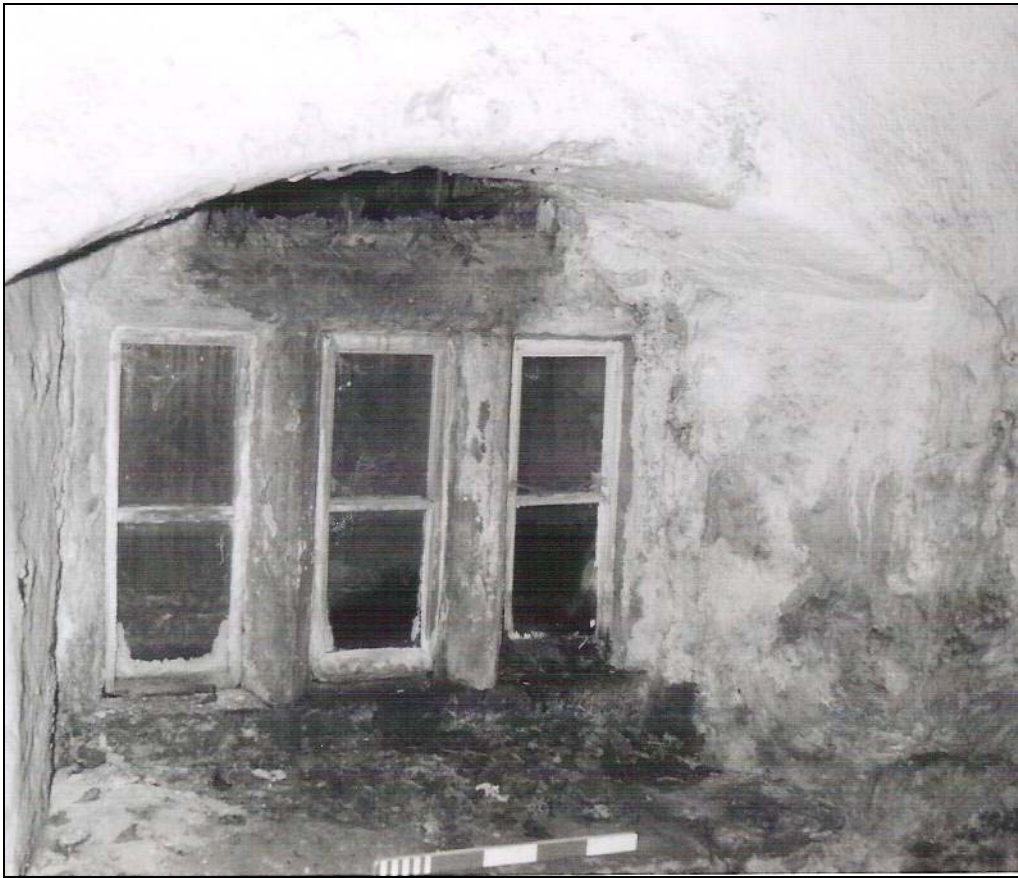
Plate 53: Mullioned window in west elevation of northern basement room
