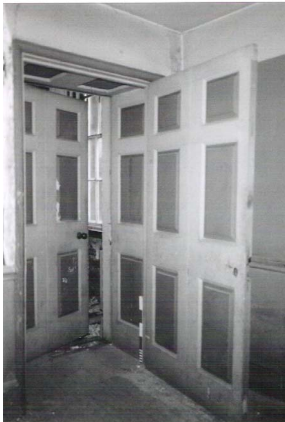
Plate 16: Double doors from stairs hall to drawing showing inner panel between
