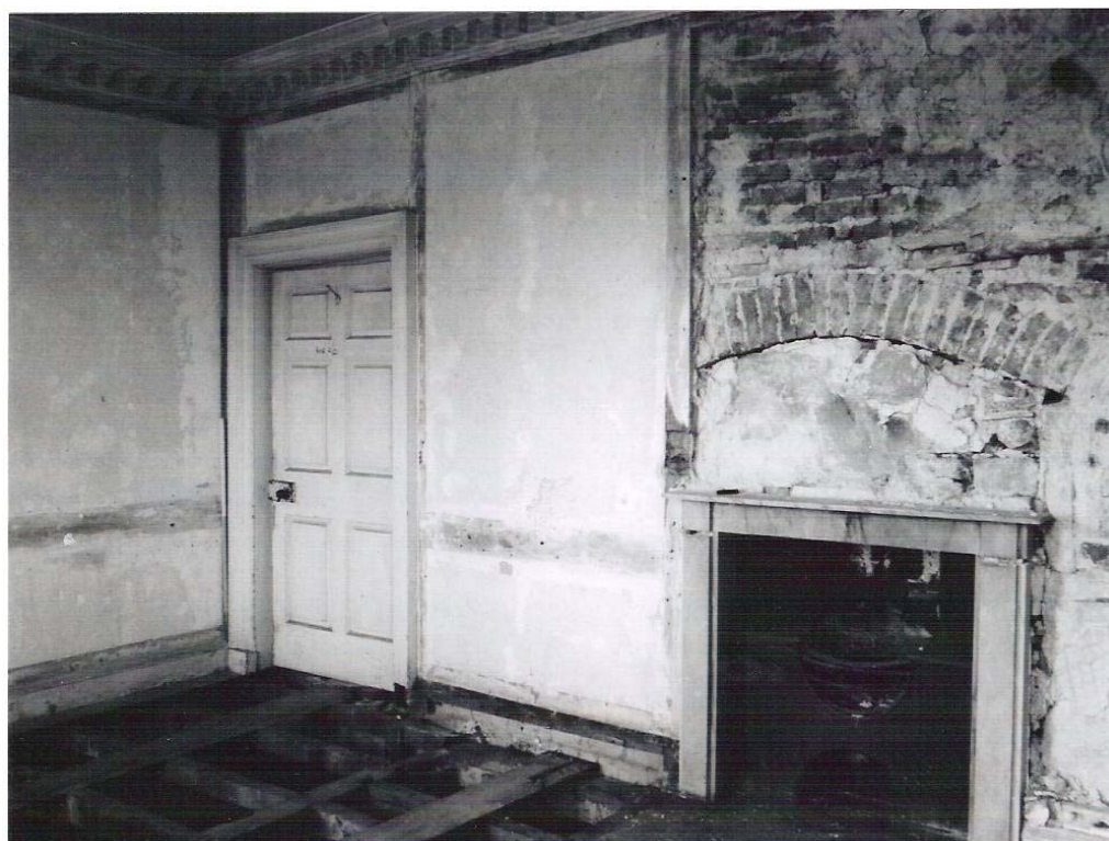
Plate 46: North east first floor bedroom: Later fireplace installed under earlier brick arch and door with six fielded panels in west wall
