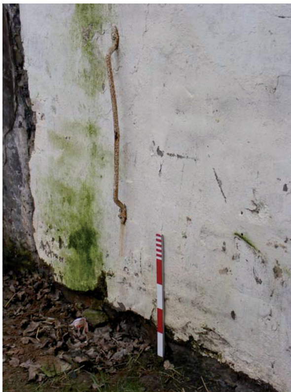
Plate 10: Detail of tying rail in former shippon in south west corner of barn
