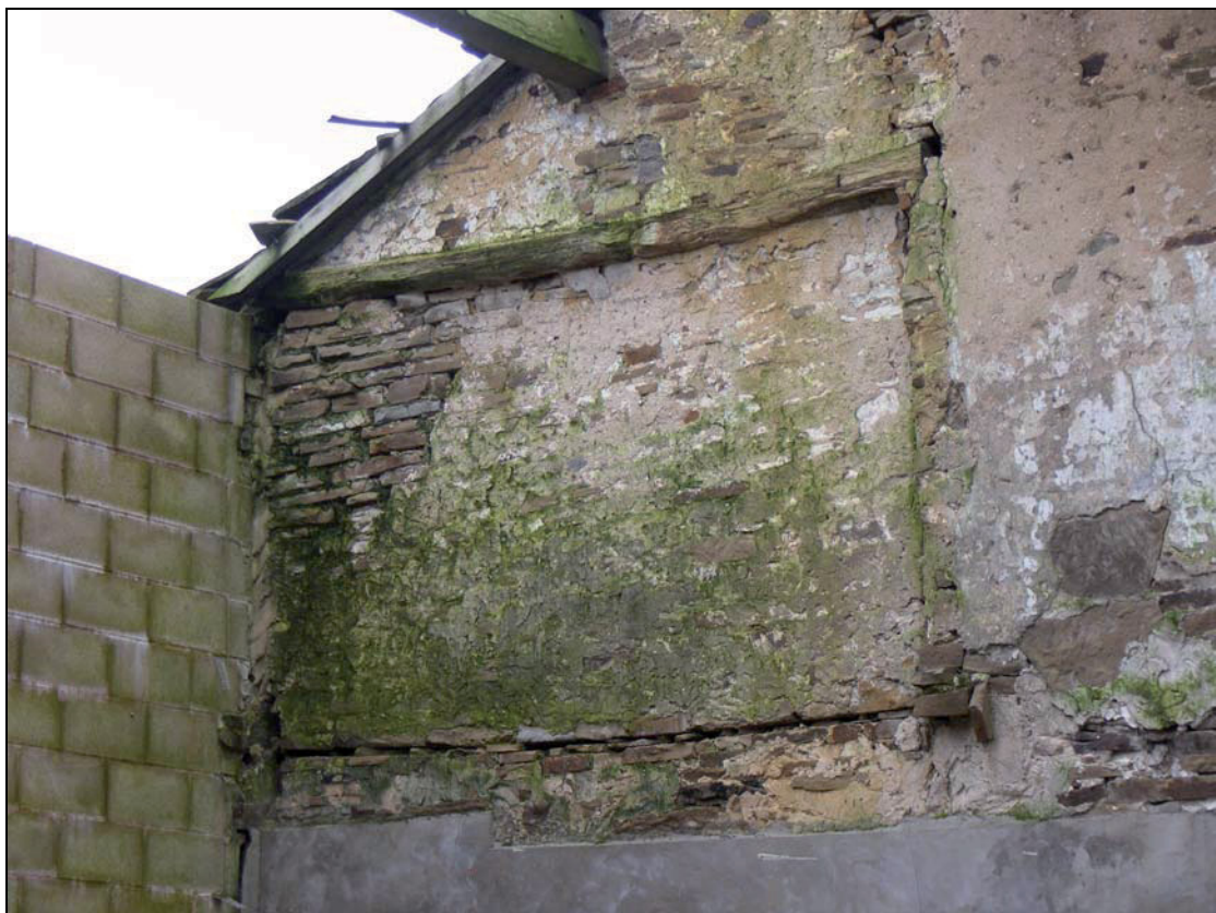
Plate 12: Handcut lintel over opening in east wall of barn
