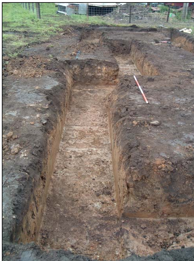
Plate 5: Trenches 3 – 5 for toilet block
