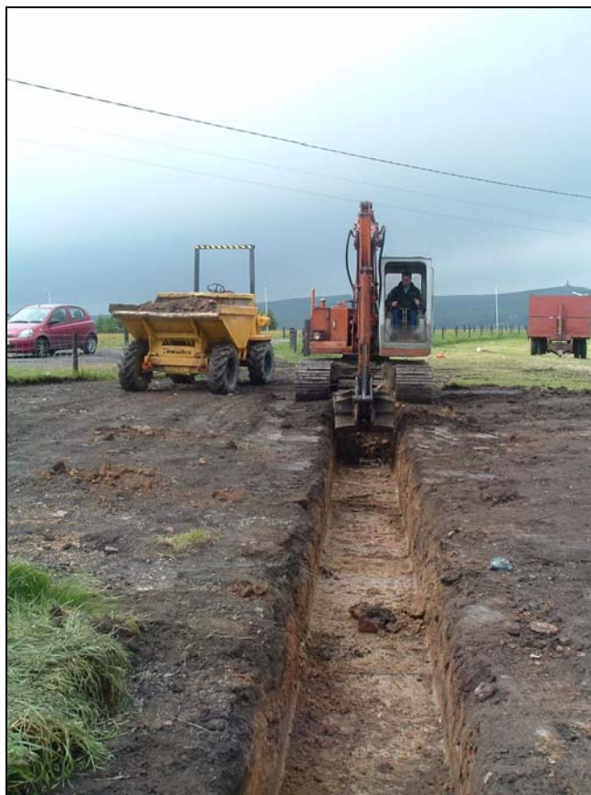
Plate 3: Excavation of trench 1
