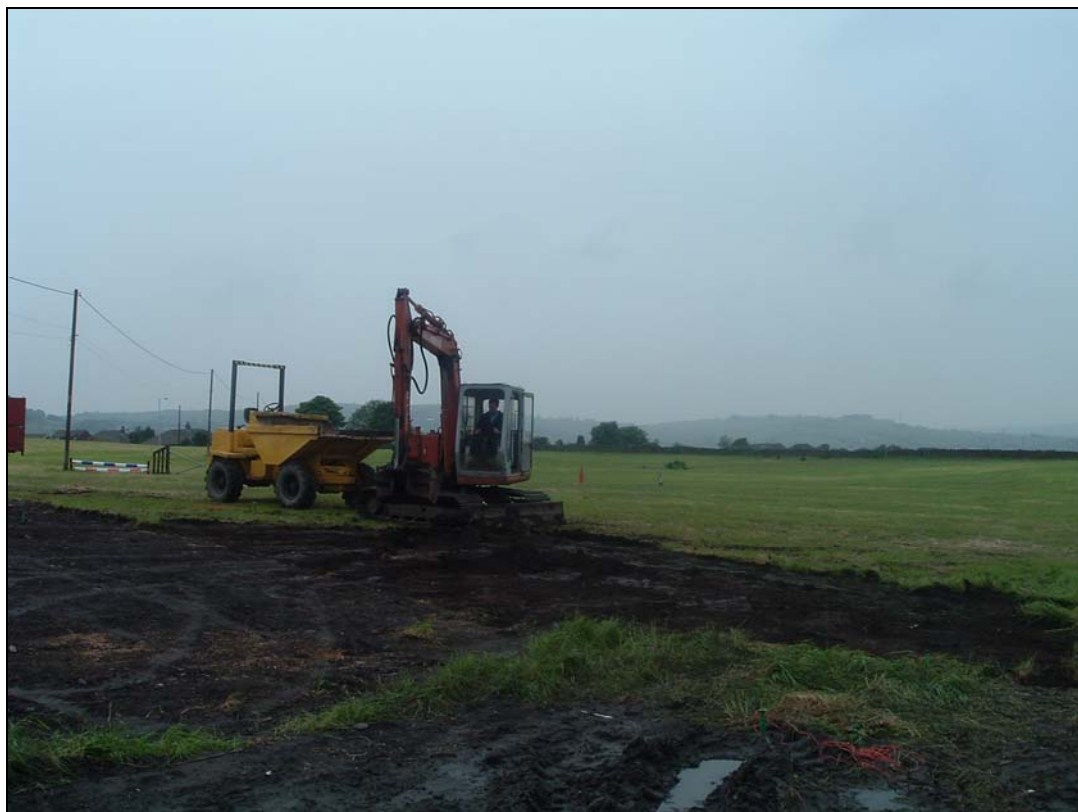
Plate 1: Working shot of initial turf stripping for toilet block
