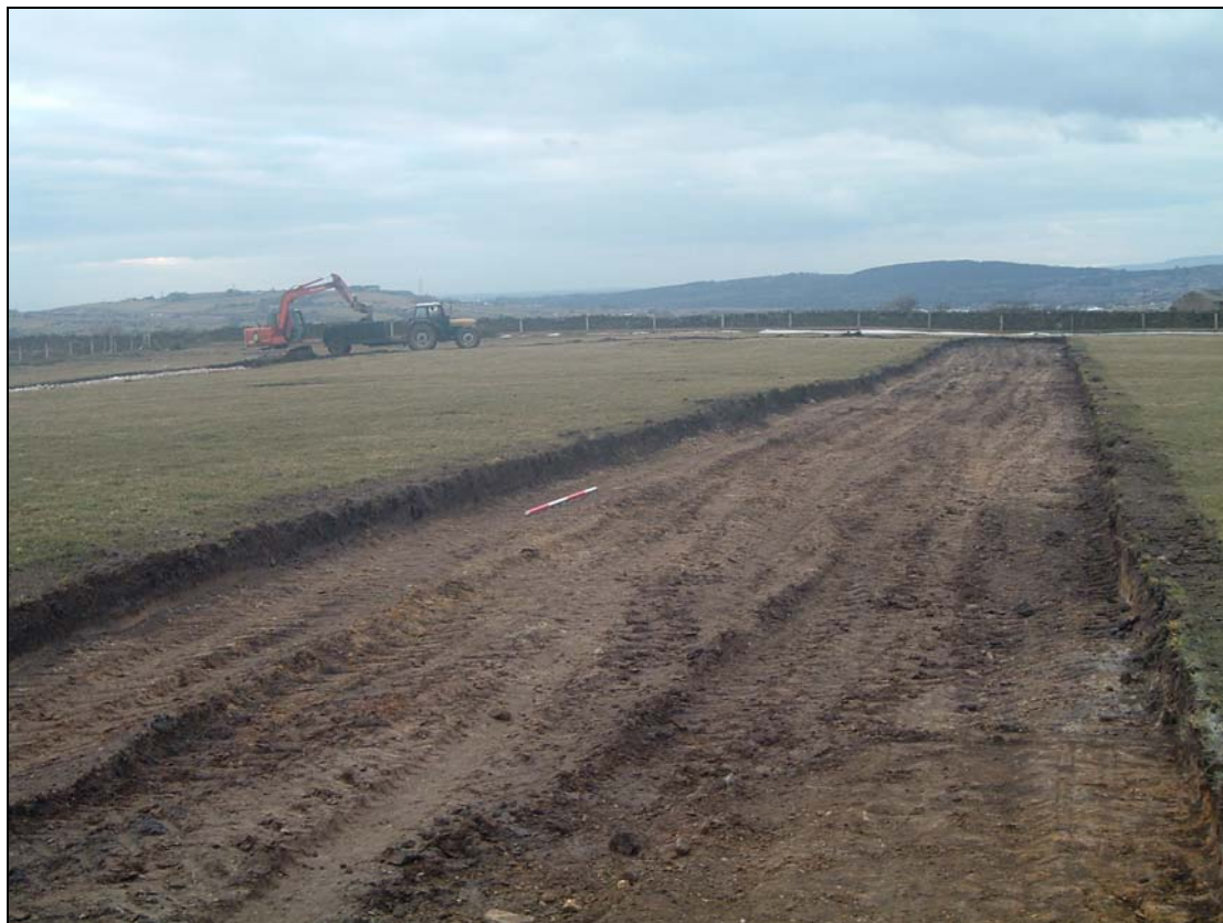
Plate 9: Caravan access track under excavation
