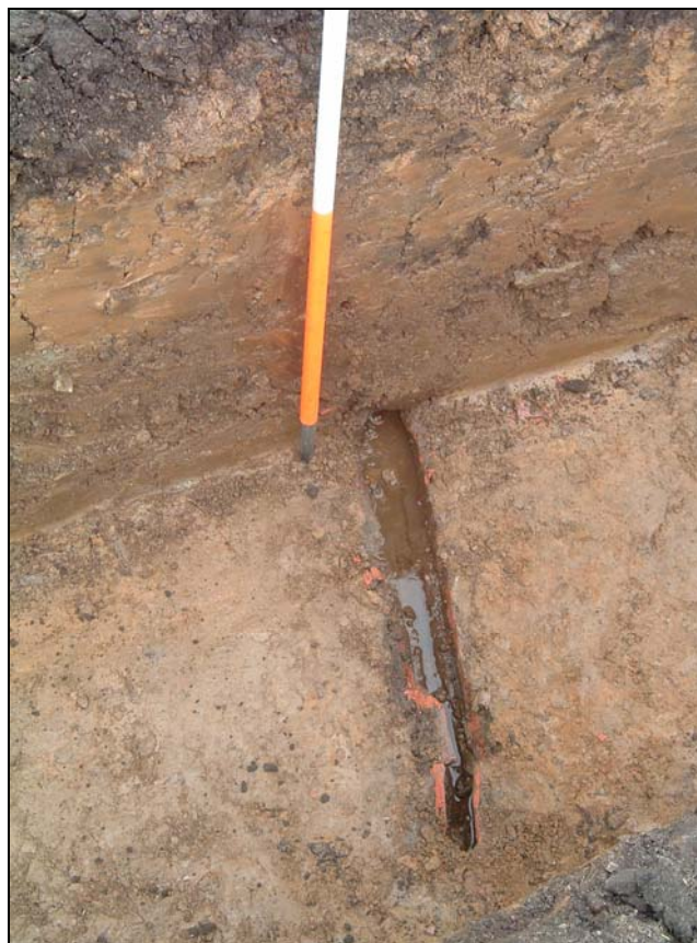
Plate 8: Top of land drain in trench
