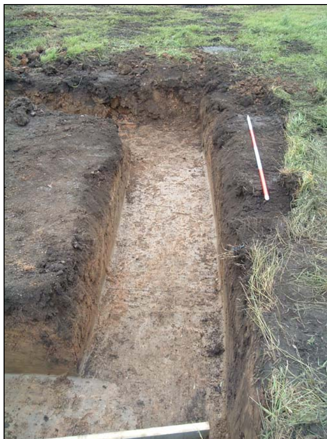
Plate 6: Trench 6 for toilet block
