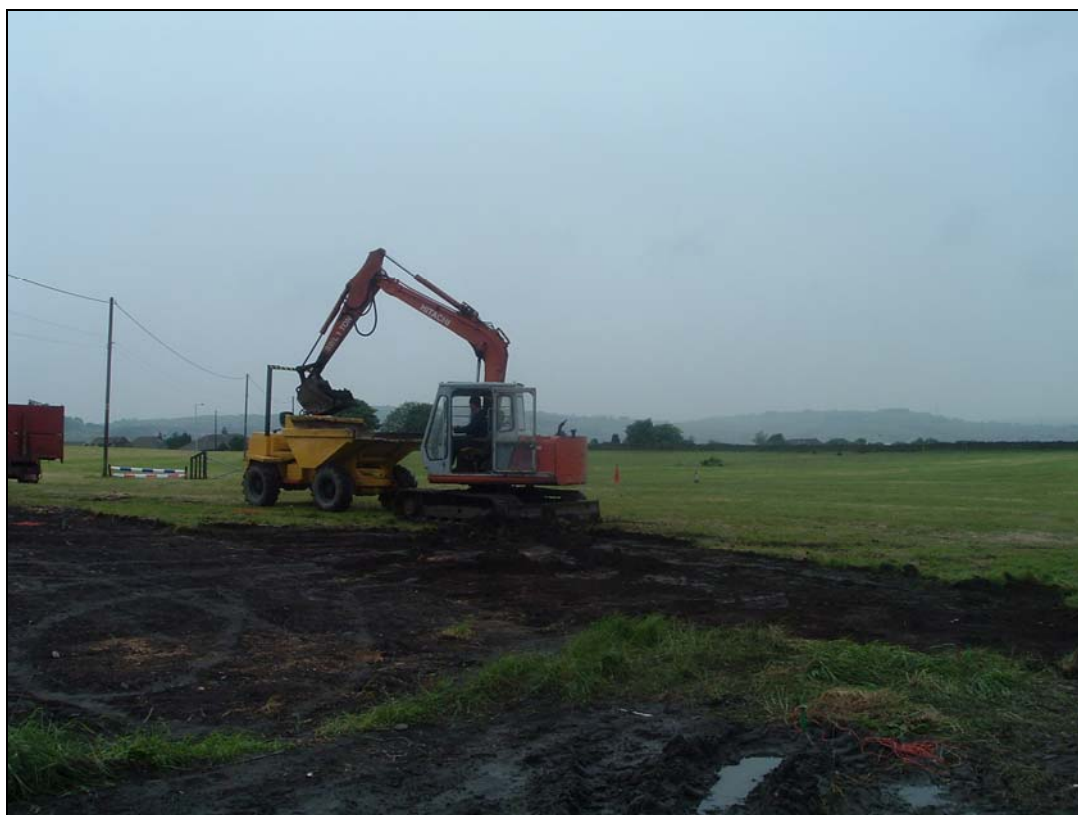
Plate 2: Working shot of initial turf stripping for toilet block
