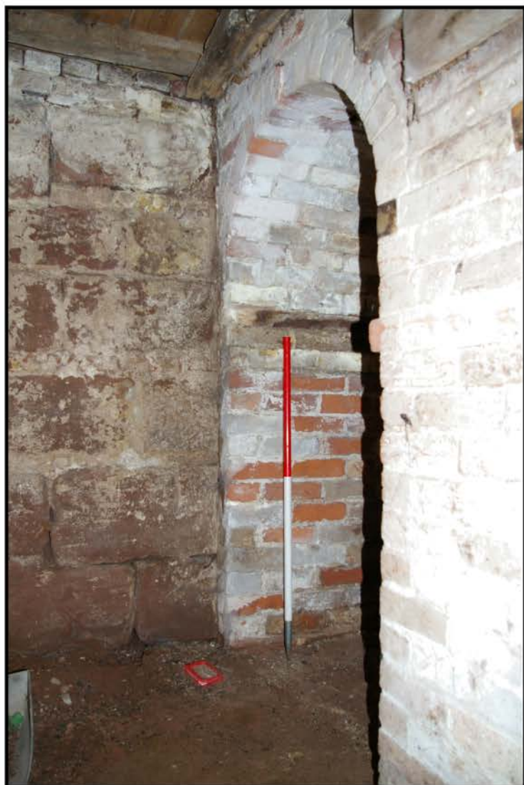
Fig 9: Farm house, cellar; phase 2 stair, showing phase 1 masonry
