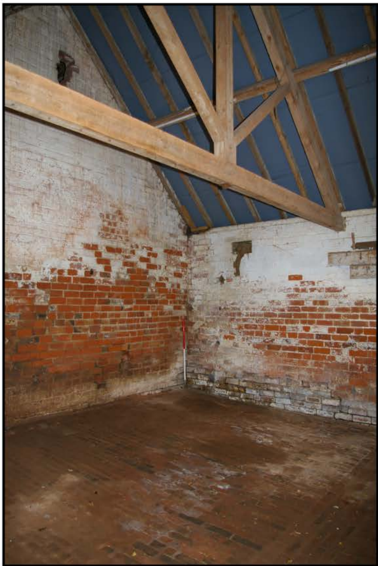
Fig 41: Combination barn and stable; stable showing king post roof truss
