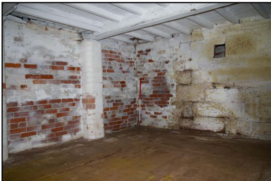
Fig 8: Farm house, cellar; phase 2, showing phase 1 masonry
