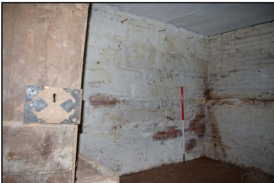
Fig 11: Farm house, cellar; phase 2, showing phase 1 masonry
