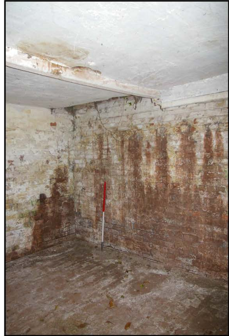
Fig 48: Stable, showing gap in ceiling for filling hay rack
