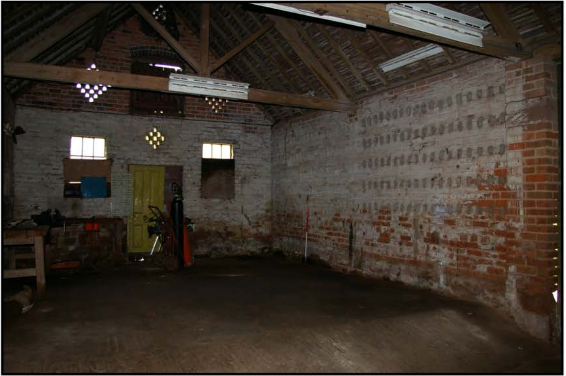
Fig 42: Combination barn and stable; barn showing king post roof truss
