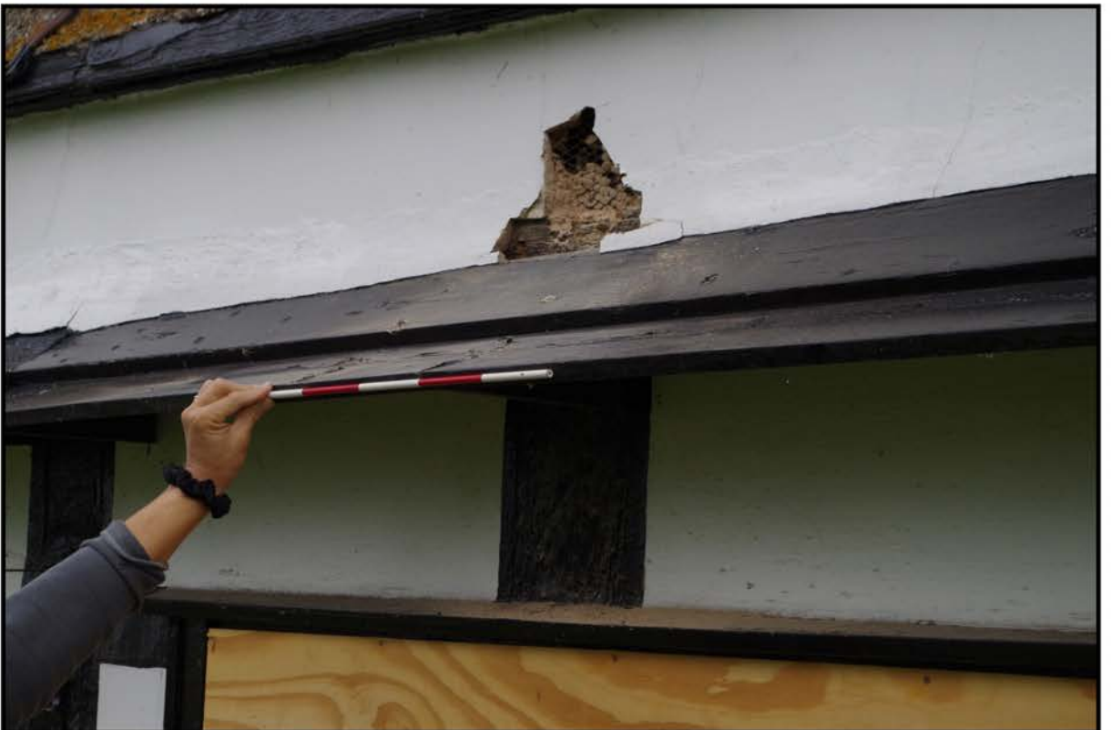
Fig 5: South-west elevation; detail of drip boards
