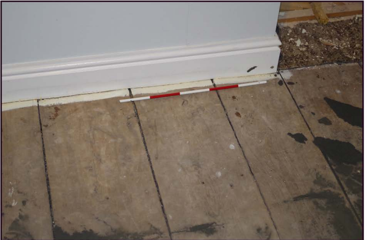
Fig 24: First floor; existing bedroom 1; detail of floorboards (scale is 0.5m)
