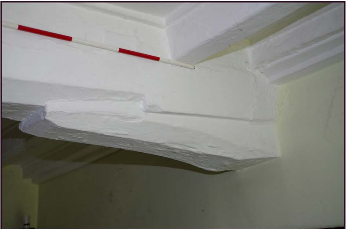
Fig 21: Ground floor; existing living room; detail of ceiling beam and support bracket
