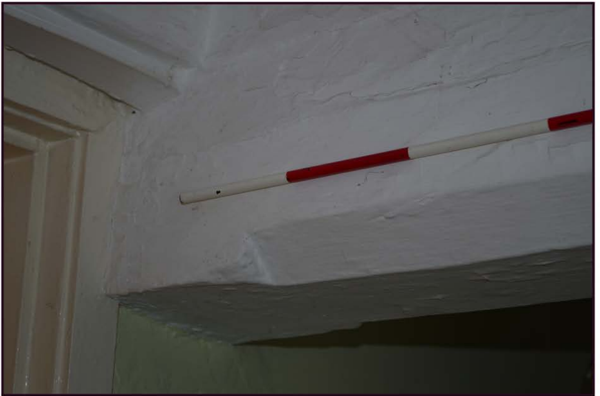
Fig 20: Ground floor; existing living room; detail of ceiling beam, chamfer and stop
