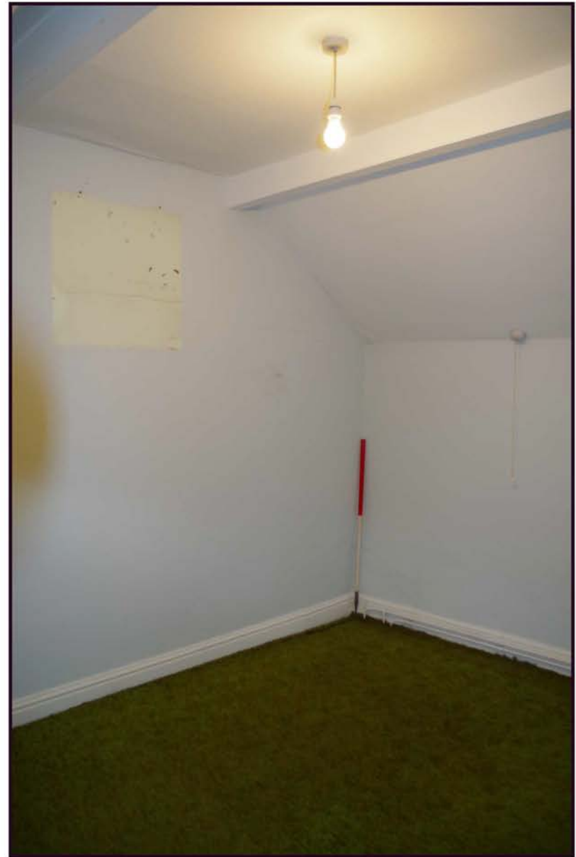
Fig 26: First floor; existing bedroom 2
