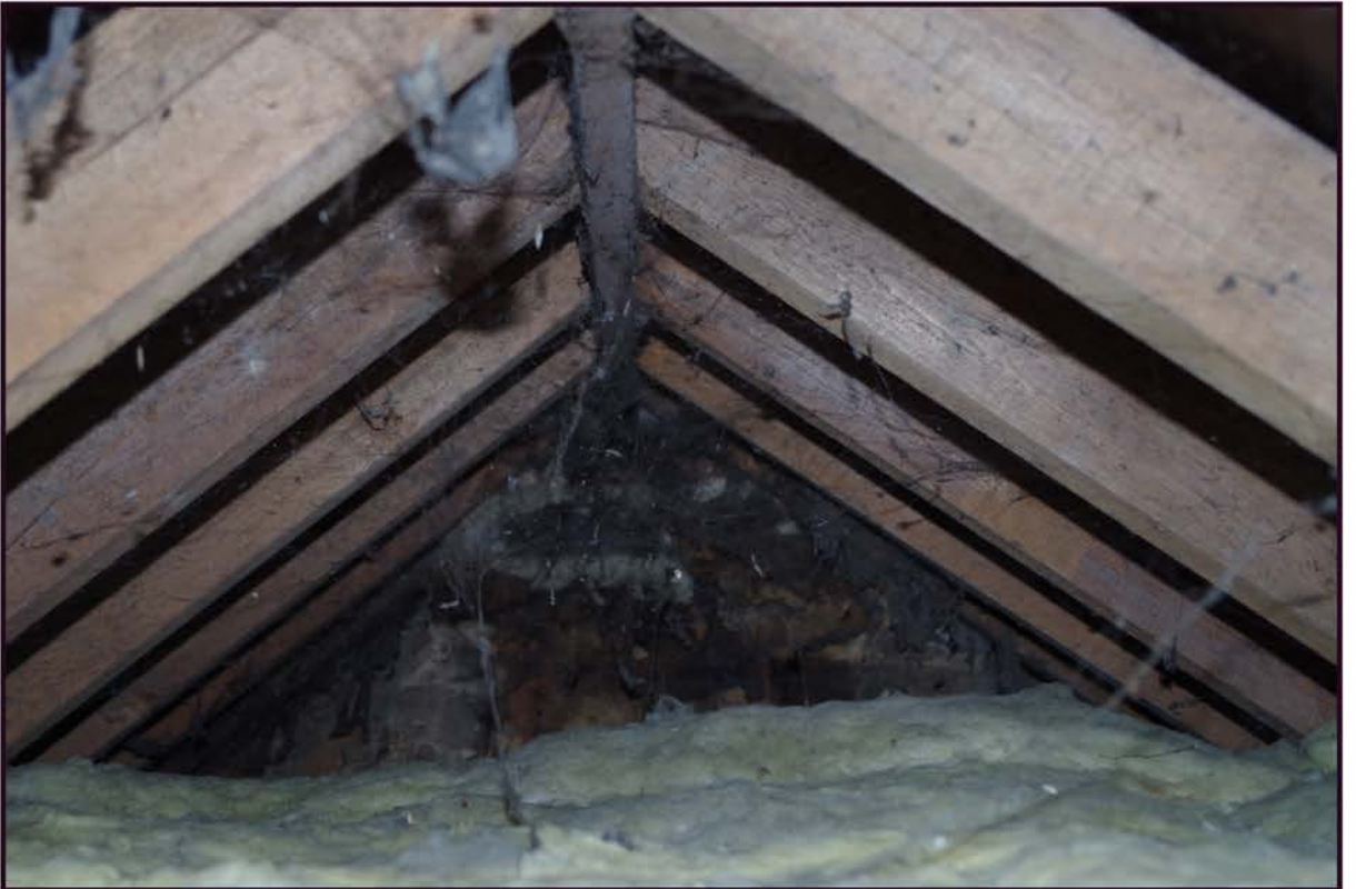
Fig 28: Roof space; detail of modern timbers
