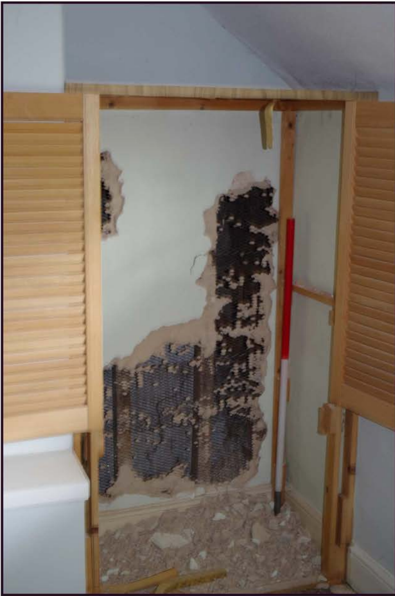
Fig 25: First floor; existing bedroom 1; detail of area of removal of plaster
