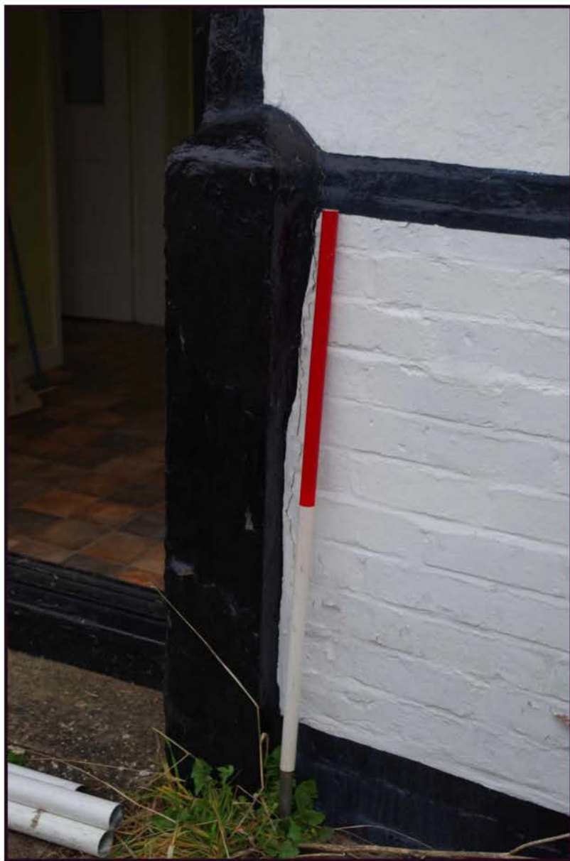
Fig 8: South-west elevation; detail of part of Phase 1 timber frame
