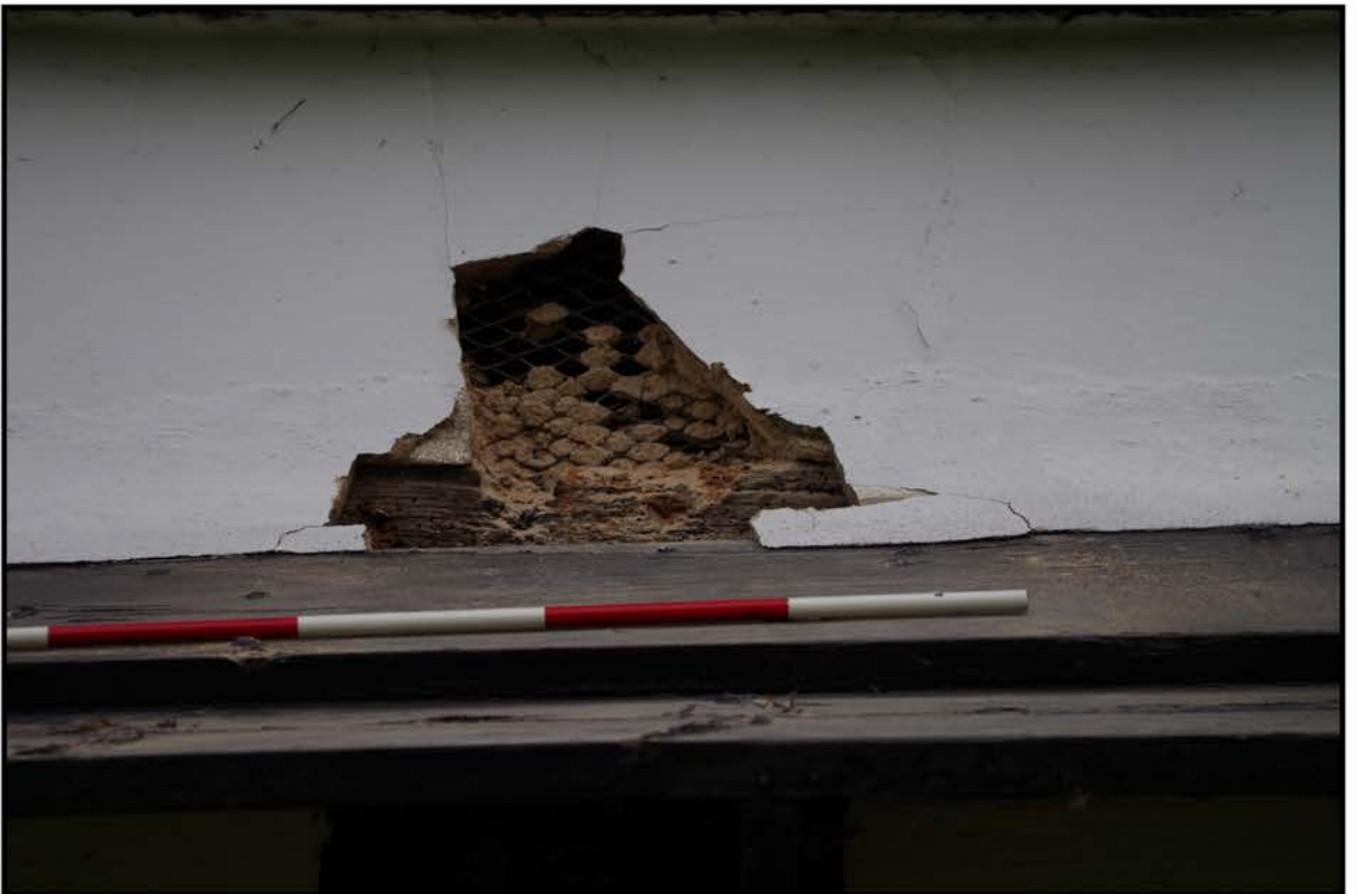
Fig 7: South-west elevation; detail of head plate or rail
