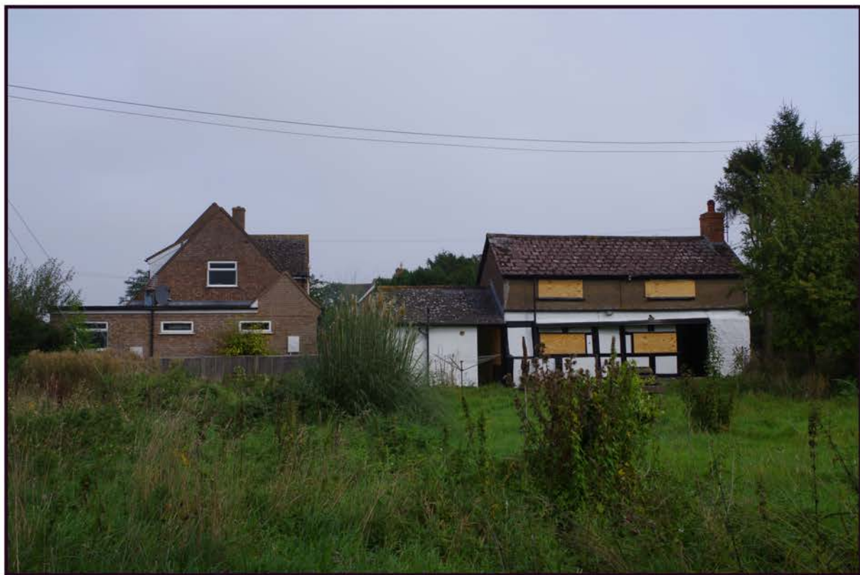
Fig 29: View of Folley Cottage from the south-west
