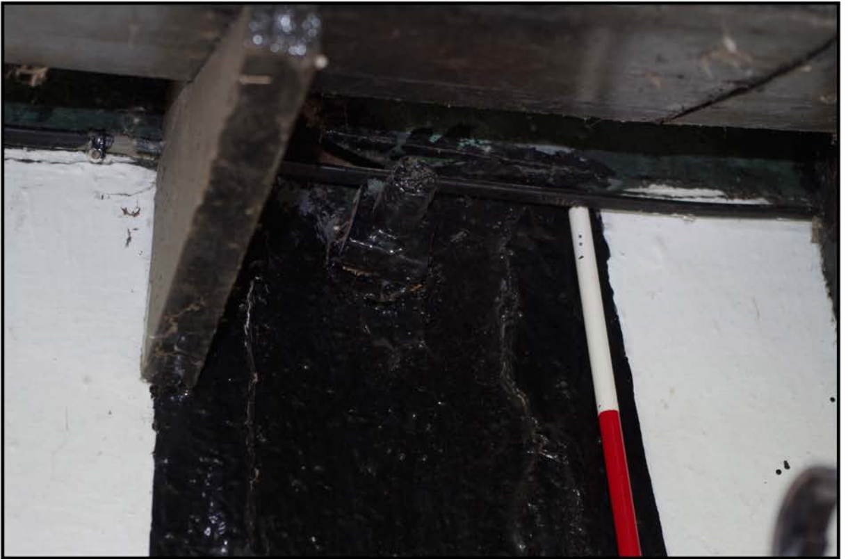
Fig 6: South-west elevation; detail of square nut securing timber frame
