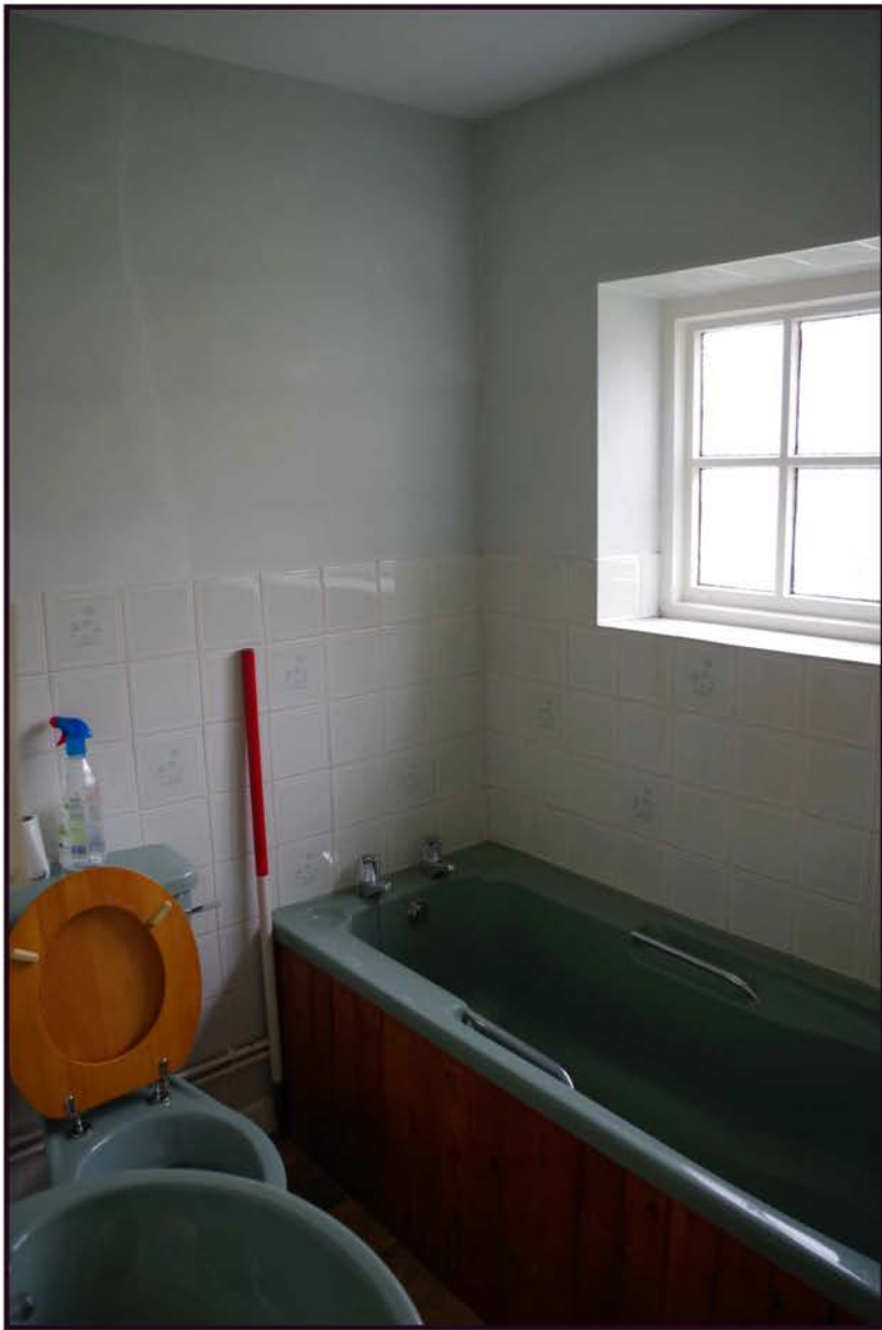
Fig 16: Ground floor; existing bathroom and toilet
