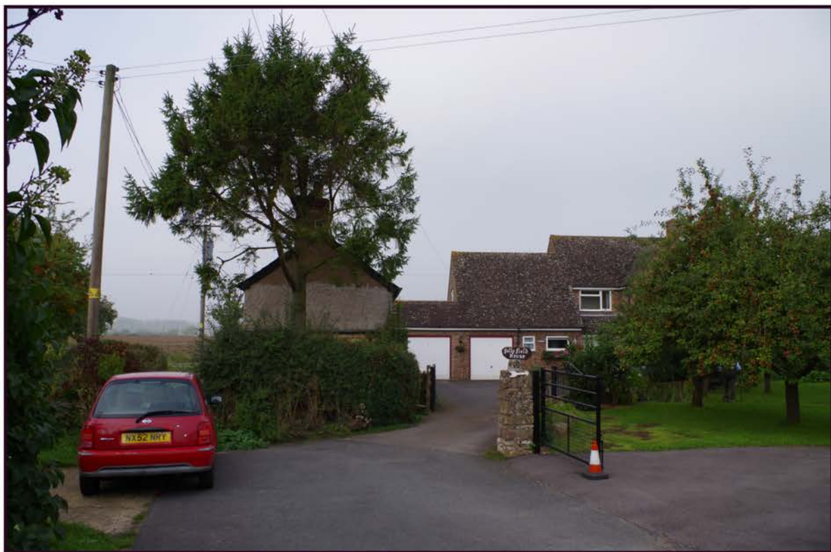
Fig 30: View of Folley Cottage from the south-east
