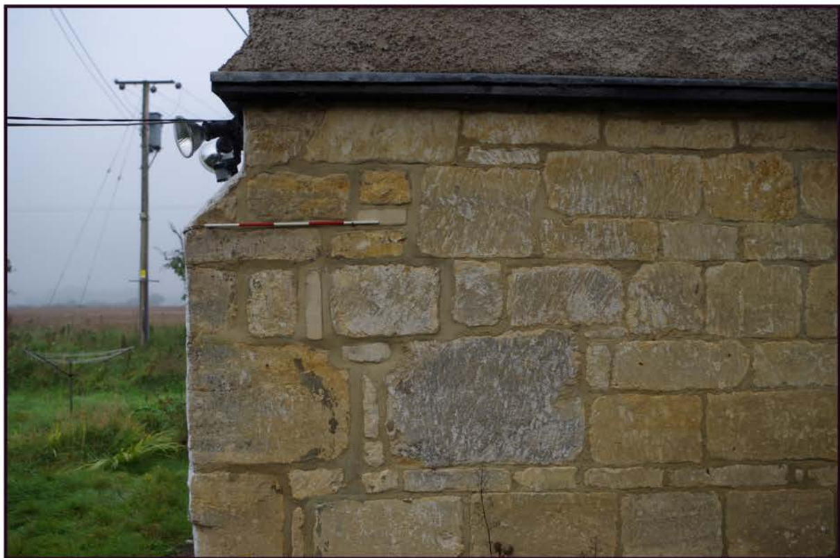
Fig 10: South-east elevation; detail of blocked window and stone with sloping end
