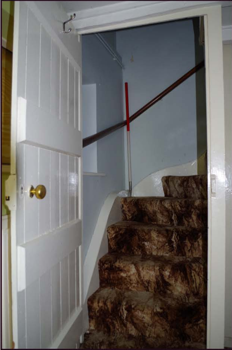
Fig 22: Ground floor; existing kitchen/diner; detail of stairwell
