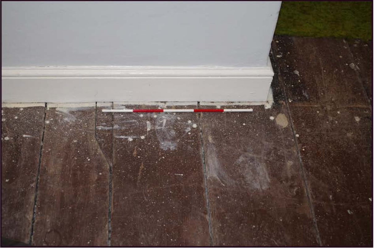
Fig 27: First floor; existing bedroom 2; detail of floorboards (scale is 0.5m)
