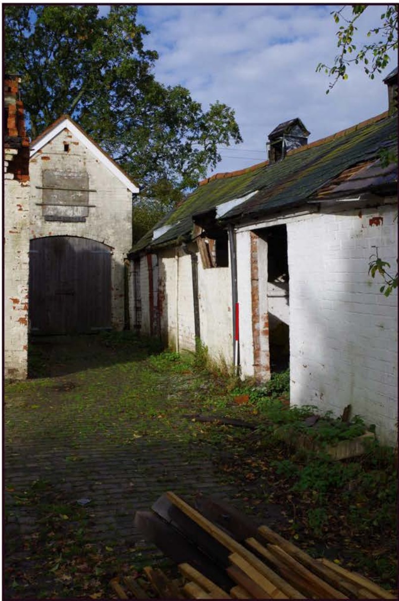
Fig 10: View of cattle and cart sheds from south-east
