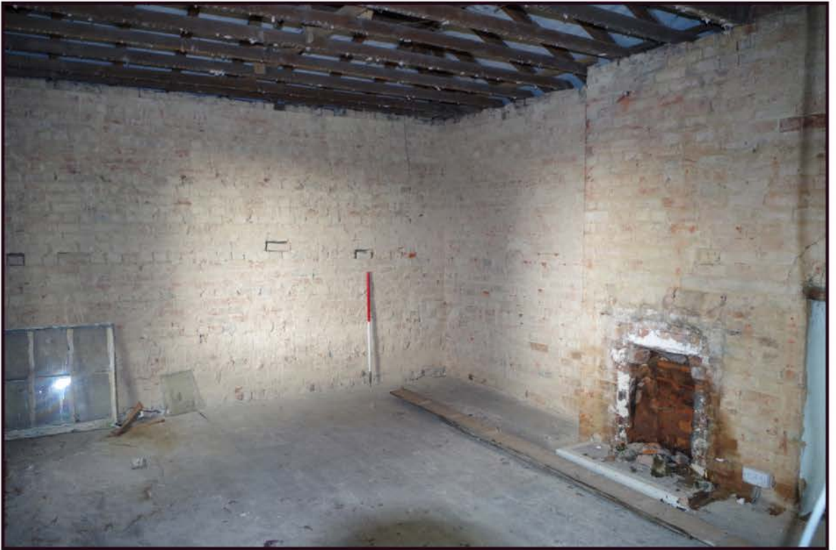
Fig 40: Phase 4; Georgian farmhouse, first floor, primary bedroom
