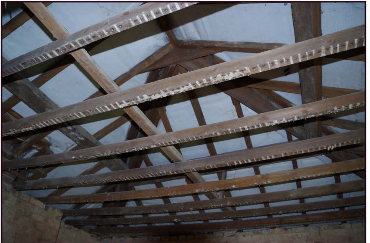
Fig 43: Phase 4; Georgian farmhouse, detail of roof structure
