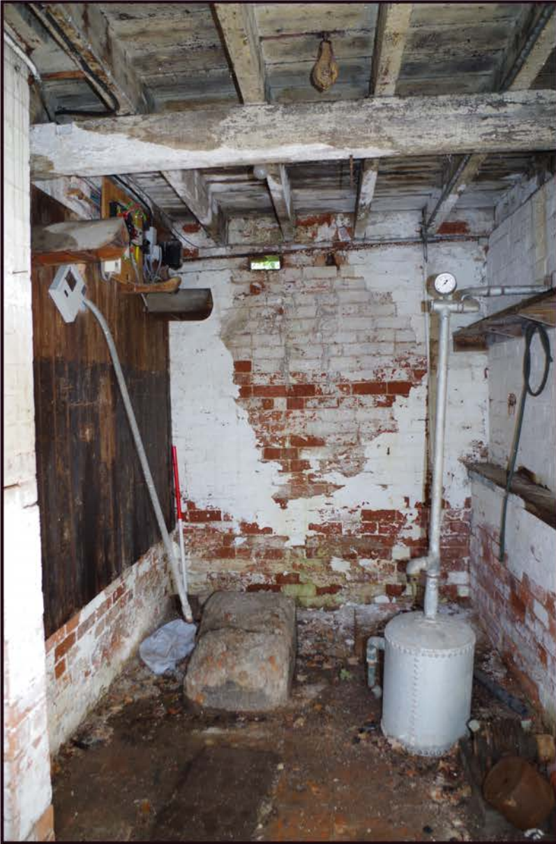
Fig 17: Tack room, subsequently generator room
