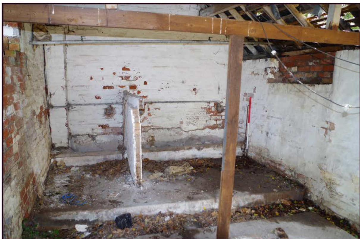
Fig 15: Stalls of cattle shed
