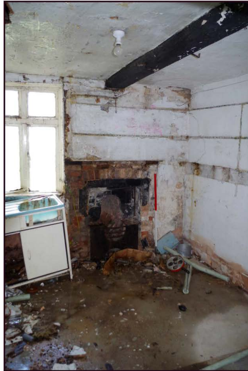
Fig 25: Phase 3; farmhouse, ground floor, kitchen
