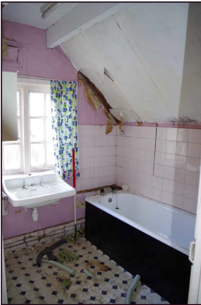
Fig 35: Phase 3; farmhouse, first floor, probably originally a bedroom
