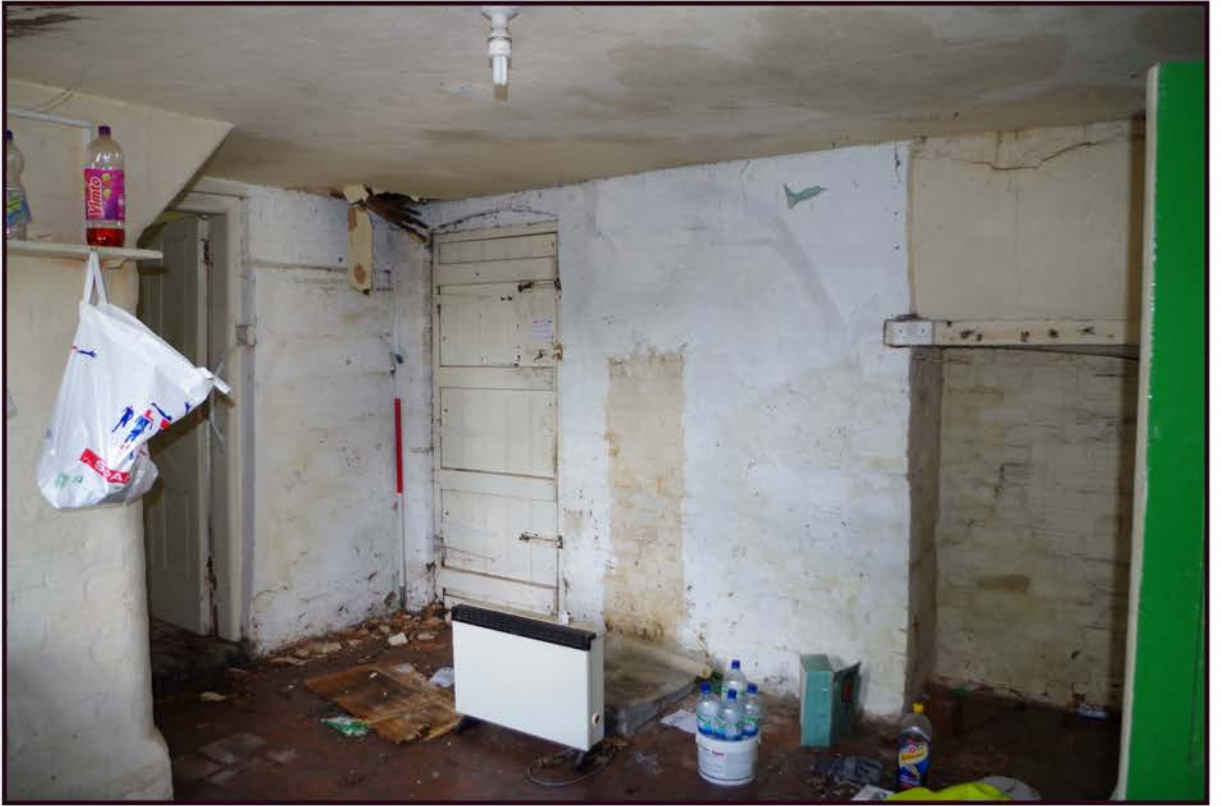
Fig 21: Phase 1; cottage, ground floor showing door to privy
