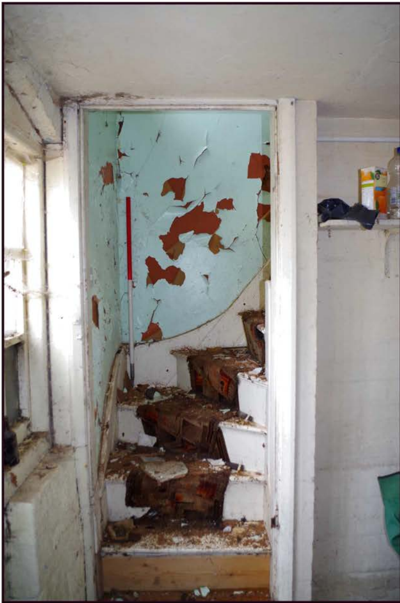
Fig 32: Phase 1; cottage; stair to first floor
