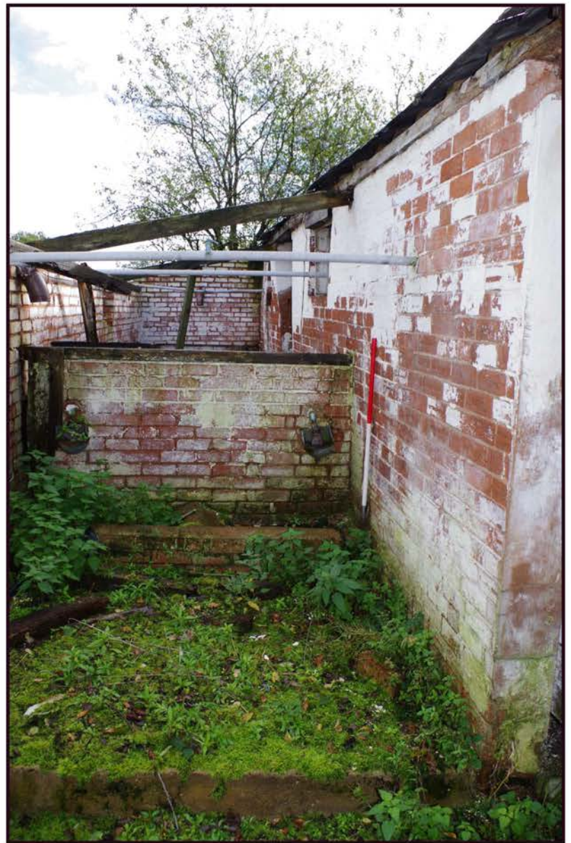
Fig 13: Stalls of cattle shed
