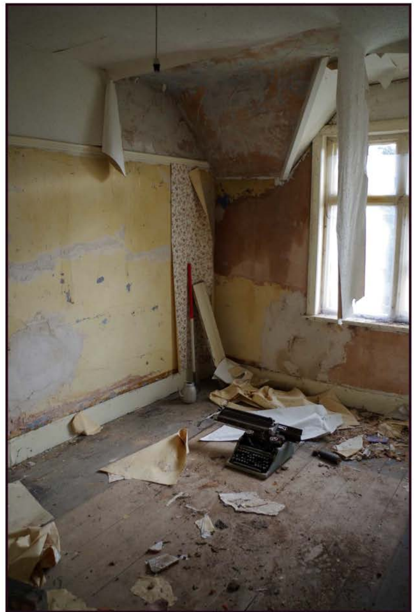
Fig 36: Phase 3; farmhouse, first floor, bedroom
