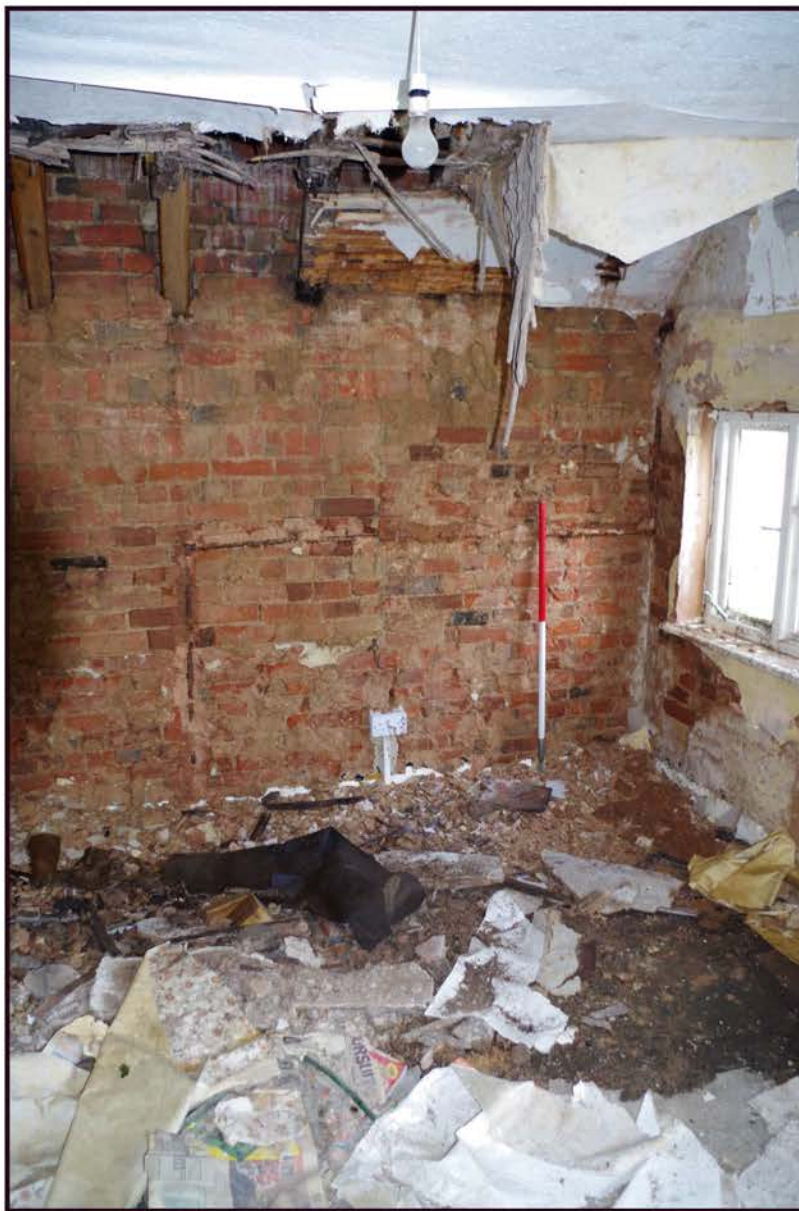
Fig 37: Phase 3; farmhouse, first floor, bedroom
