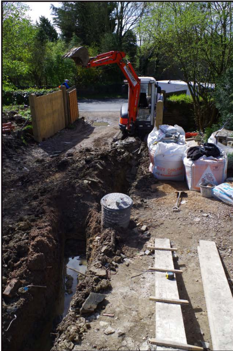
Fig 6: View of excavations looking south-west
