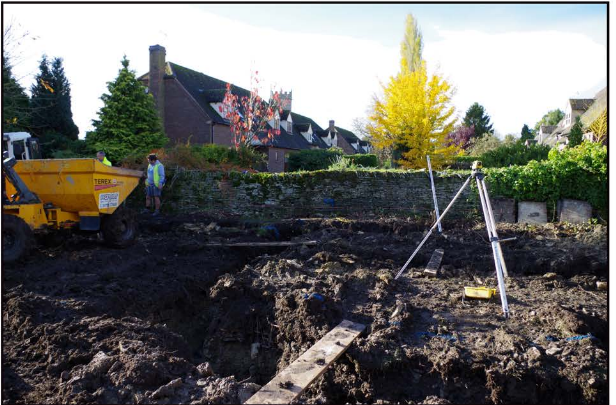
Fig 5: View of excavations looking west
