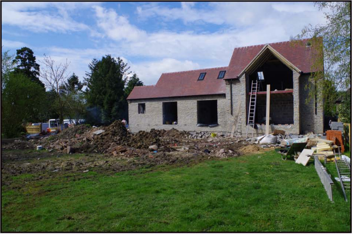
Fig 7: General view of site after erection of new building
