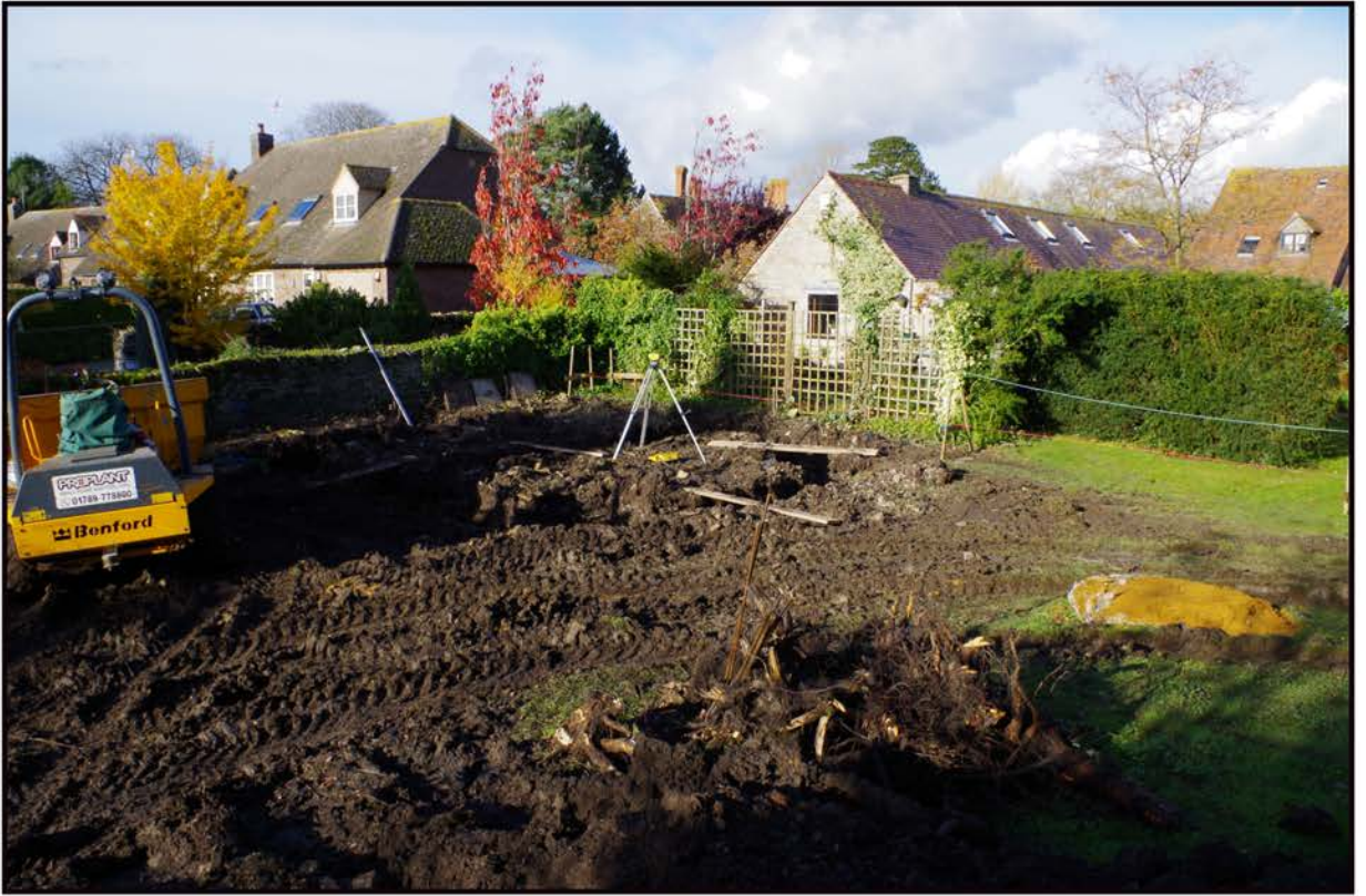
Fig 4: View of excavations looking north-west
