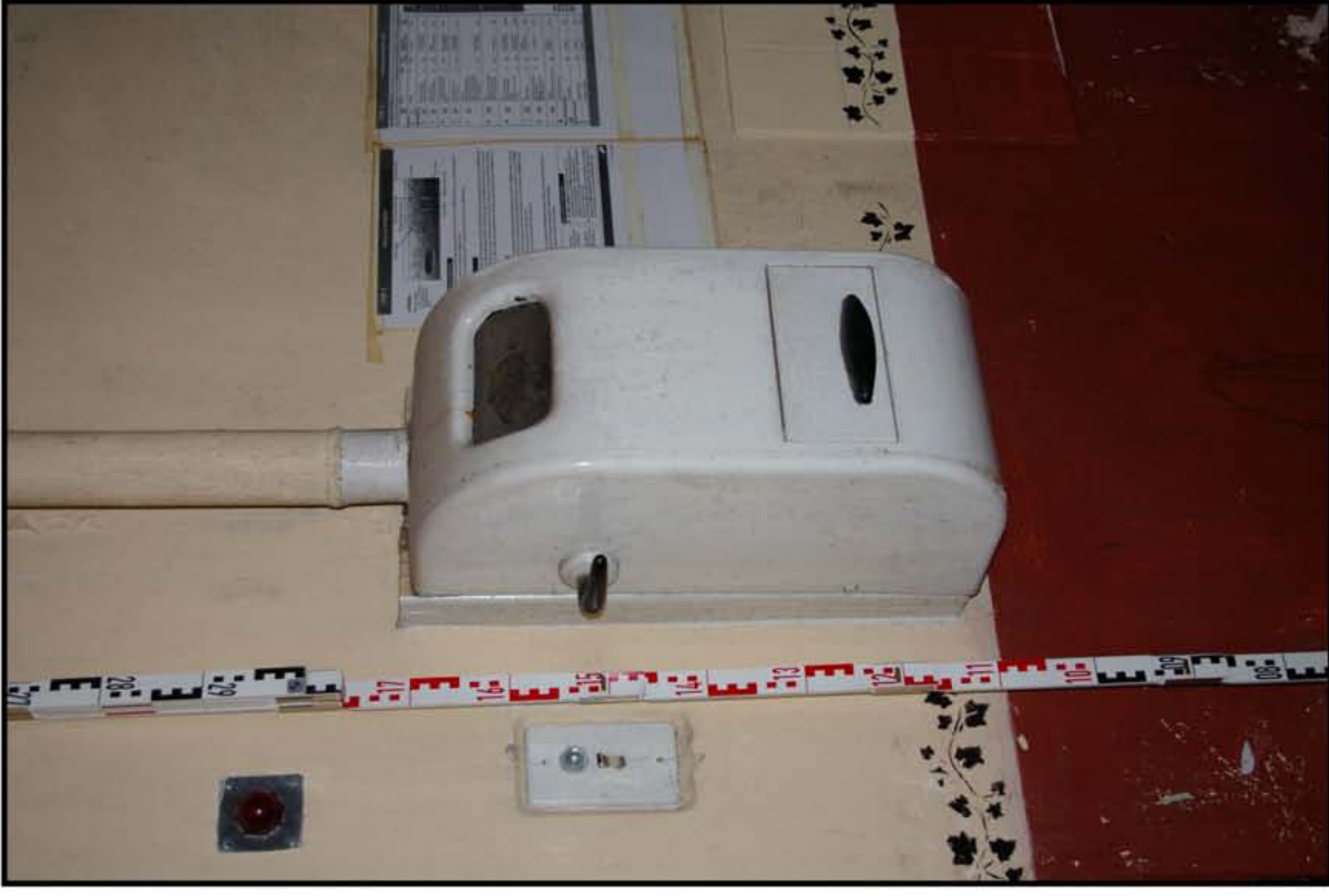
Fig 21: Incinerator for disposal of female hygiene items
