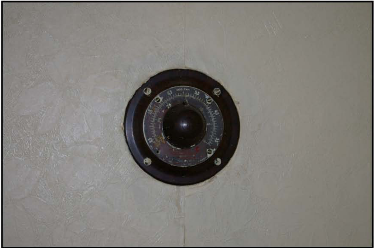
Fig 16: Example of original underfloor heating control, Wulfruna Court
