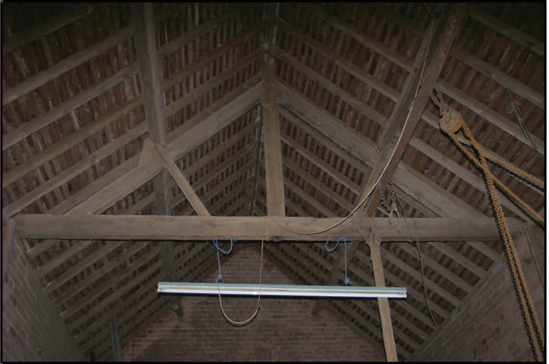
Fig 30: King post roof truss in barn
