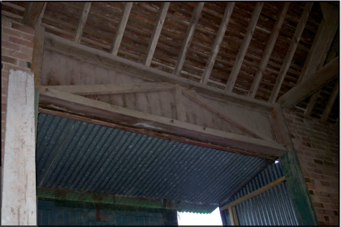
Fig 31: Wooden beam bridging cart entrance in barn
