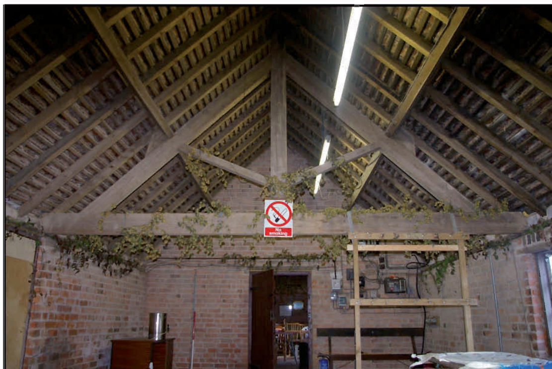
Fig 29: King post roof truss in hay loft
