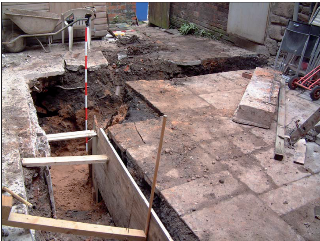
Plate 2. The 'L' shaped footings trench taken from the west
