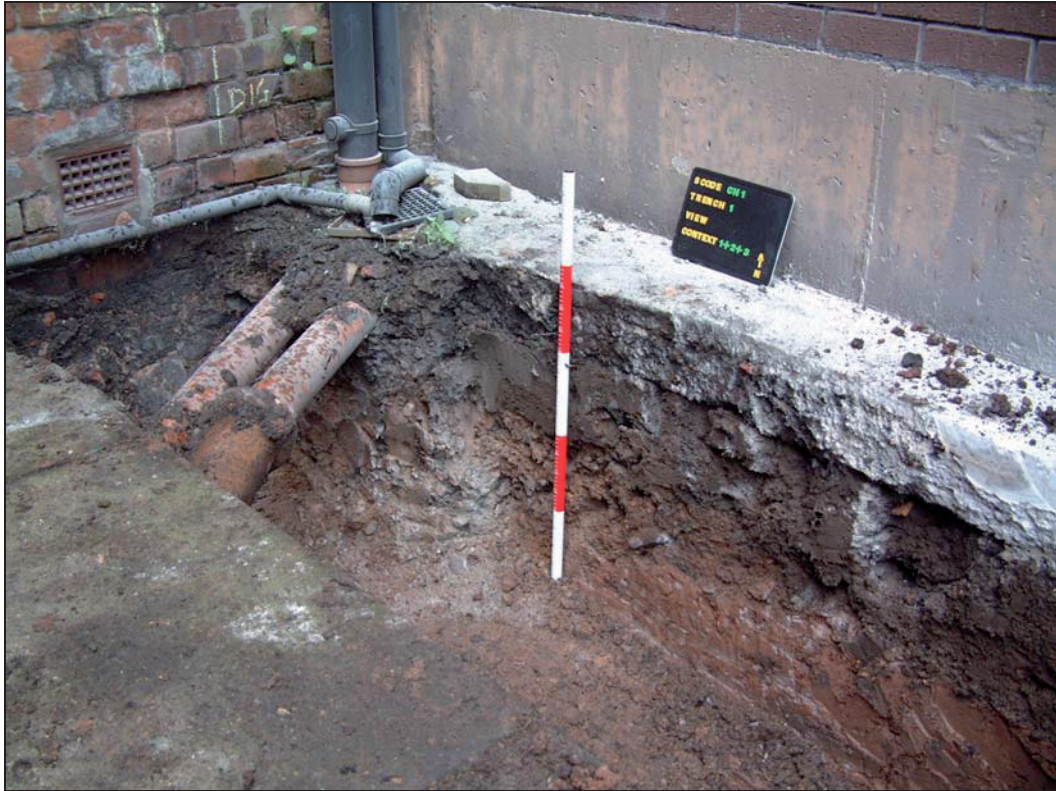
Plate 3. 6" pipes located at the western end of the trench from the southeast
