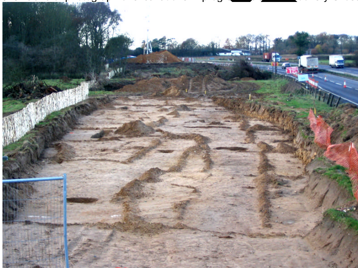
Plate 5. General photograph of excavations in progress at Site 2, Rookery Crossroads
