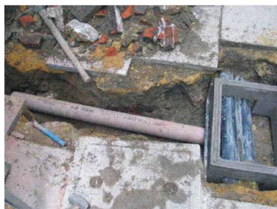
4 Connection to Priory House, showing ground conditions
