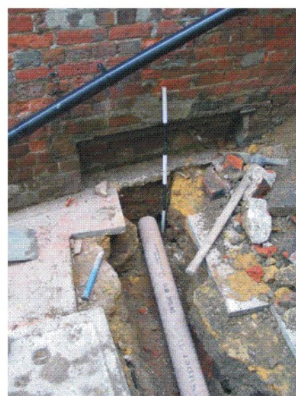
5 Connection to Priory House, showing new supply going through blocked basement window
