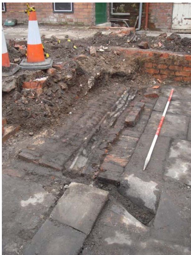
Plate 12: Factory F3 and drains
