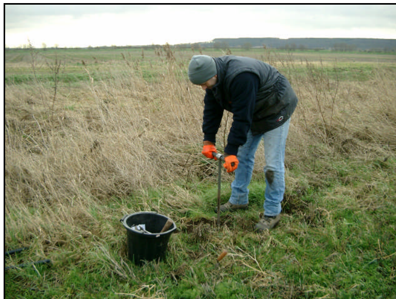
Plate 4.2: Excavation of piezometer borehole in advance of installation (© Malcolm Lillie).
