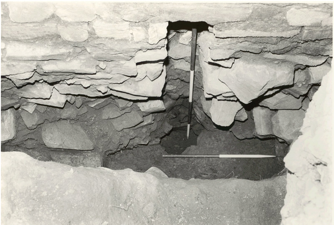
Fig. 12: Site A. The corner turret pile slot from the north-west
