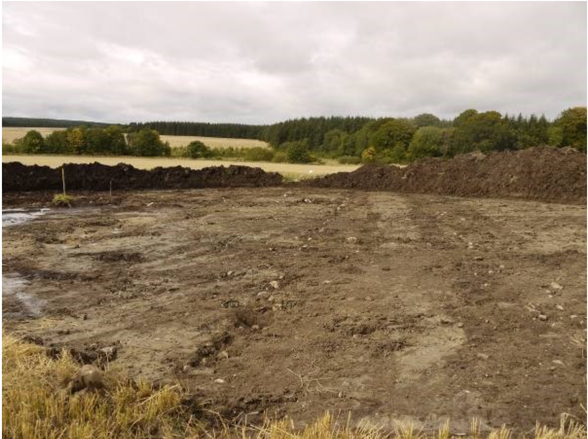
Illus 9 Stripped area for Turbine 2 looking North West, field drains visible running diagonally across area
