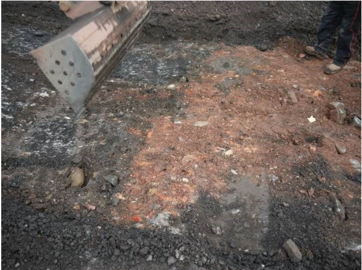
Illustration 6 Apparent edge to crushed brick and slab surface at Northern end of stripped area
