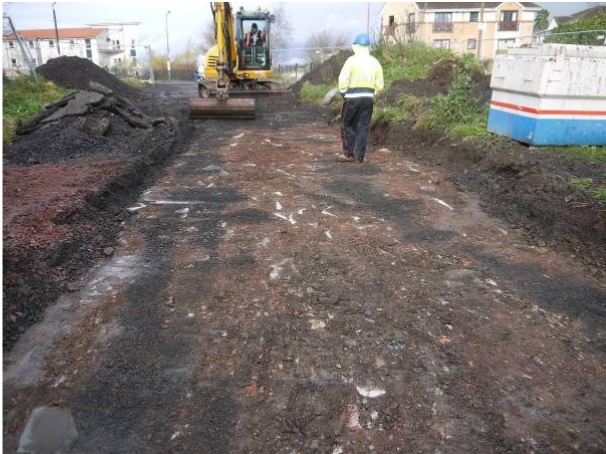
Illustration 4 Stripping of road planings and Type 1 hard core revealing broken paving slabs and crushed brick looking North West
