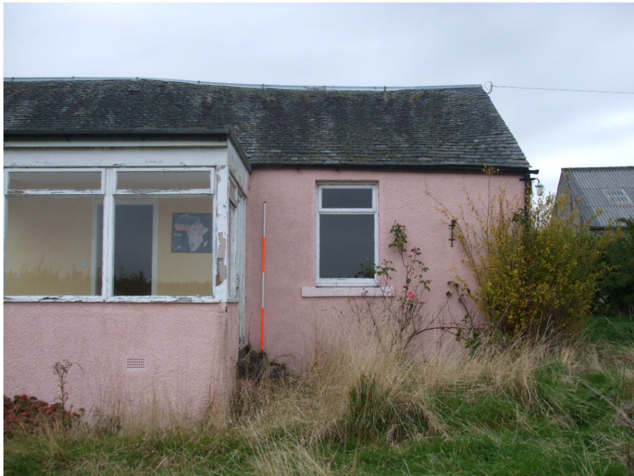
Illus 12 window at eastern end of south facing elevation of southern wing and porch (note sag in roof line)
