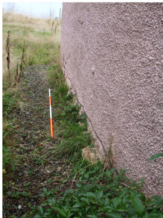
Illus 14 stepped foundation course under western wall of southern wing of farmhouse
