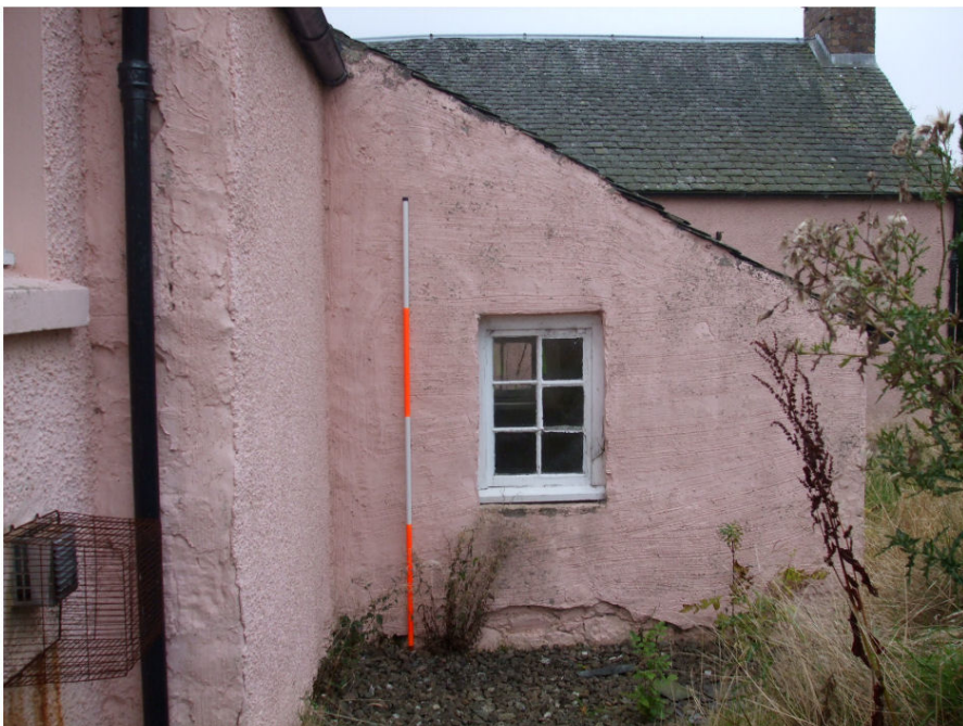
Illus 8 North facing gable of Western extension (stonework visible in cracked harling)
