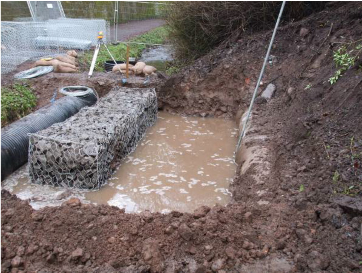
Illustration 5 Excavated area to West of Skinner's Burn looking North showing existing sewer pipe and wall and foundation trench in section
