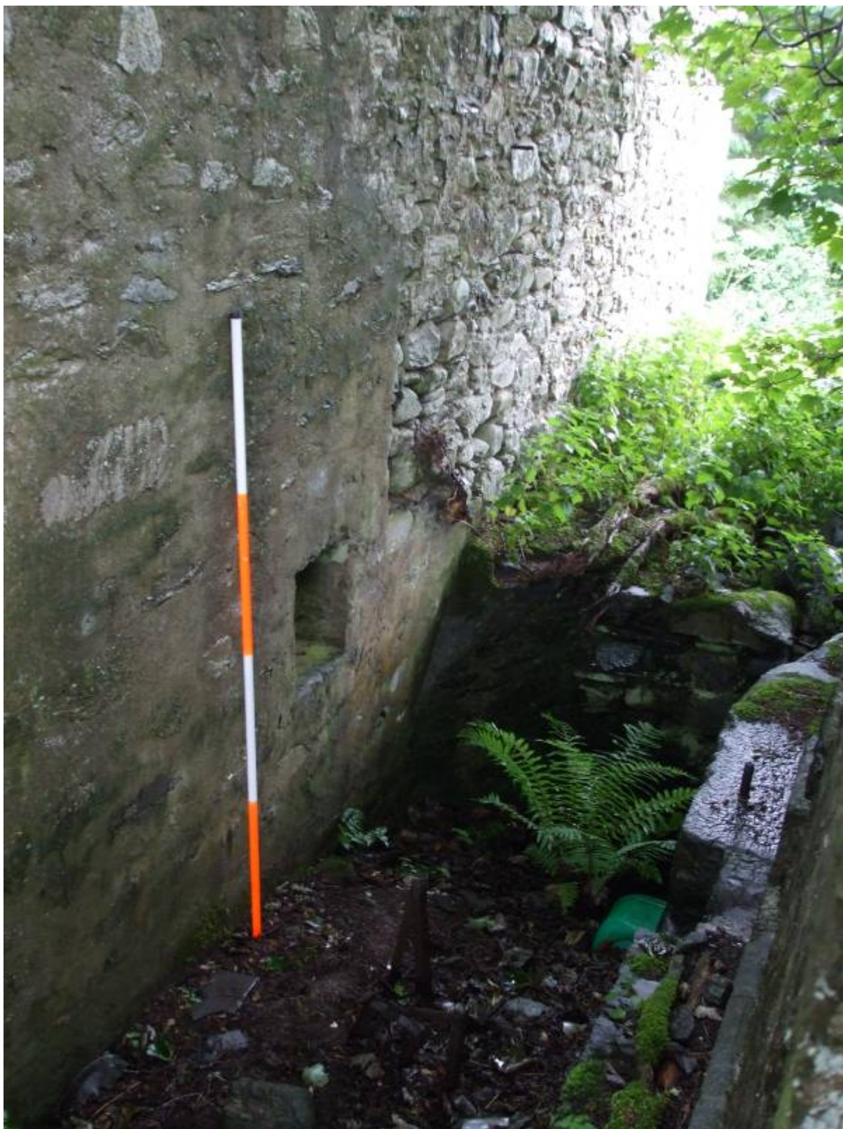
Illustration 18 Socket for mill wheel in Western elevation of Building A
