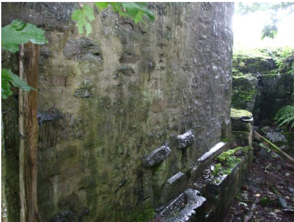
Illustration 17 Wall on Western side of wheel pit looking North West showing socket for mill wheel
