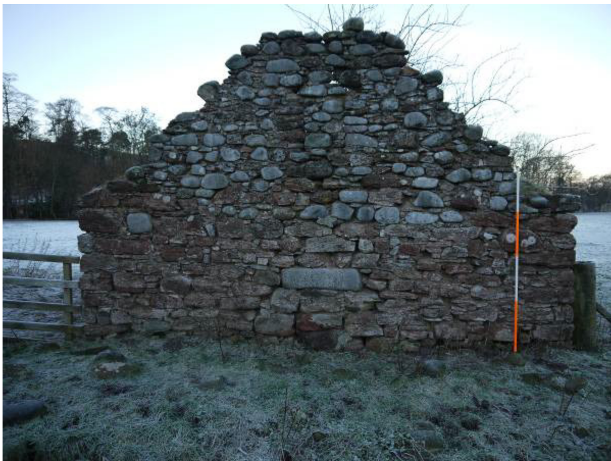
Illustration 8 Eastern gable of mill cottage/dam house showing blocked window just below gable and access point at ground level looking West
